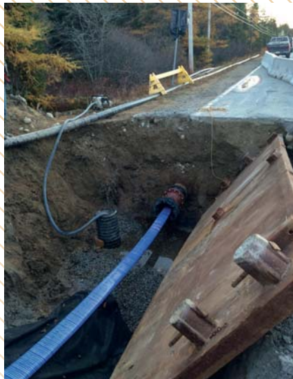
The Primus Liner exits the host pipe.
