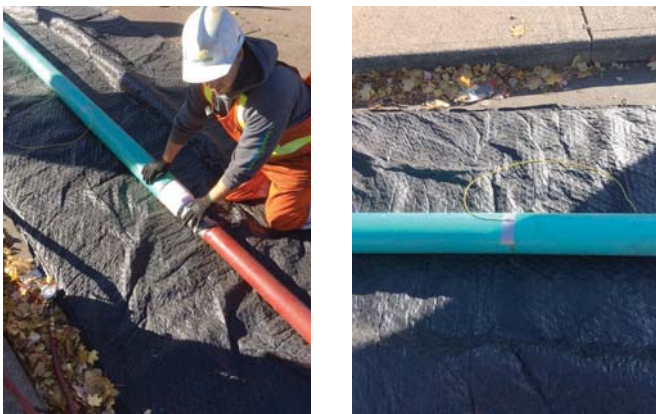
Figure 3: Lateral sample creation on site with thermocouple for temperature monitoring.
