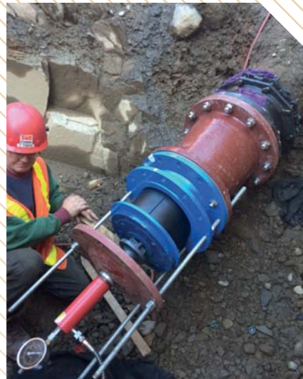
A Primus Line connector during assembly.
