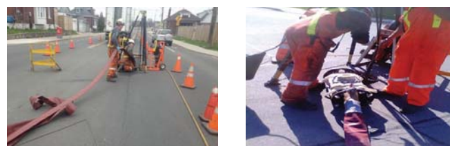
Figure 1: Installation setup for lateral liner.
