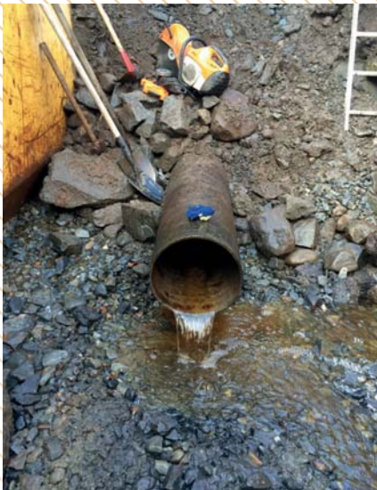
Host pipe after the cleaning cycle.
