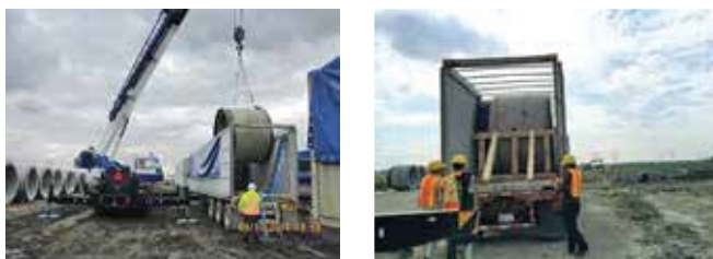
Figure 4. Pipe Delivery and Removal from Shipping Container
