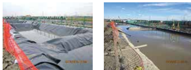
Figure 5. Slurry Settlement Ponds Prior and During Construction
