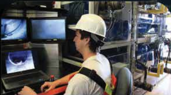
Totally Trenchless Lateral & Mainline Lining
