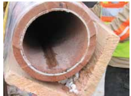
Figure 2. The invert of the CIP liner.
