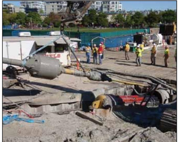
Figure 2 – Reaming and swabbing operations were completed without any serious complications.
