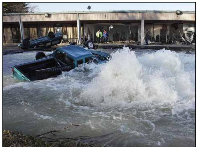
**Figure 1 – The result of a 54-in. PCCP failure in January 2011.**
