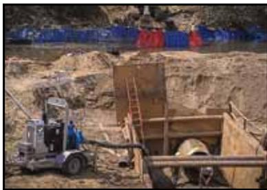
A pipeline construction project replacing a deteriorating 42-in. pipeline more than 20 ft below the surface of a small river met with trouble as unstable shores prevented directional drilling. Rain also brought constantly changing river levels,
