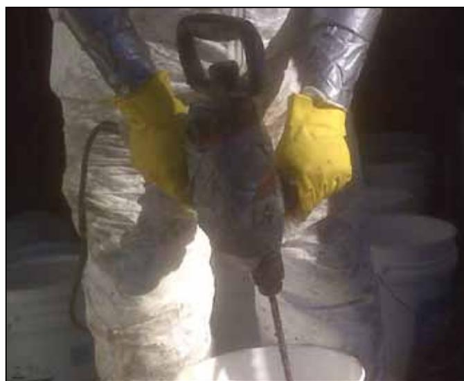
Figure 5 – Mixing of the epoxy material.
