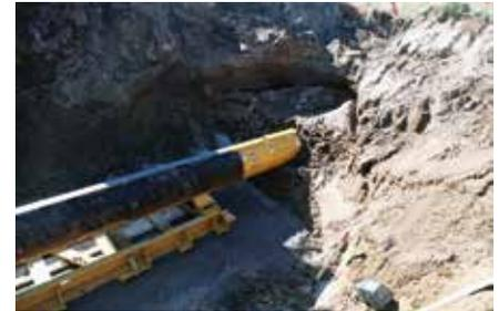
A McLaughlin On Target steering system was used during auger boring on the Rush Creek Interceptor Project. The massive wastewater pipeline project in Hamburg, N.Y., is expected to last into early 2017. Rush Creek is a project for the Erie County Department of Environment and Planning. The project is designed to abandon an existing wastewater treatment plant. Right now, the plant cannot handle the water capacities it is taking in. The project will also eliminate overflows into Rush Creek.
