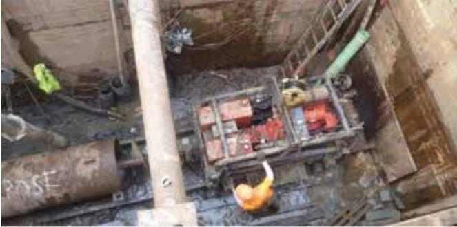
Figure 2 – Crane ready to pick ABM in the event of significant water flow through casing.
