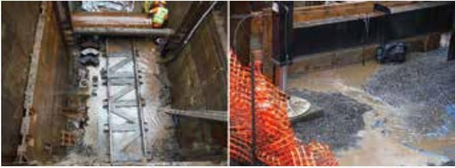
Figure 1 – (Left) Flooding within the launch shaft; (Right) Channel of surface water flowing into the launch shaft
