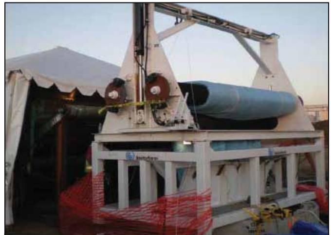
Figure 3 – Over-the-hole wet out.
