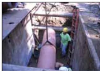
which required a 1,400-ft section of the total 2,400 lf of sewer pipeline to be sliplined. The section consisted of manhole drop connections and elevation changes, creating a hill that would require extensive excavation for insertion pits, making it difficult to avoid public disruption. It was determined that sliplining was the best option for the section.
