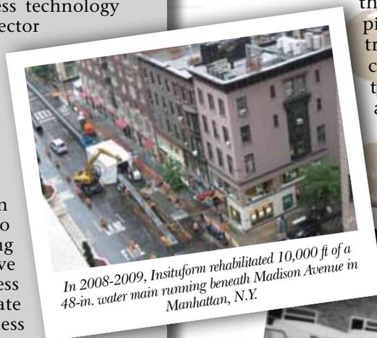
*In 2008-2009, Insituform rehabilitated 10,000 ft of a 48-in. water main running beneath Madison Avenue in Manhattan, N.Y.*
