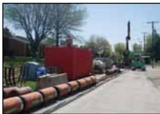
The Shively Interceptor Project in Shively, Ky., is the third largest pilot-tube microtunneling (PTM) project ever completed in the United States. Midwest Mole was the contractor on the project that consisted of the installation of more than 10,678 lf of vitrified clay pipe (VCP)
