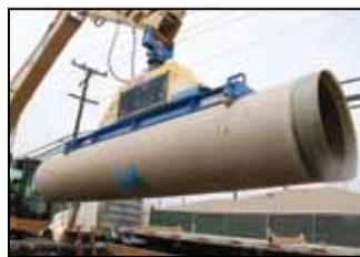
Akkerman, Inc. and HOBAS Pipe USA were involved in the Magnolia Trunk Sewer Rehabilitation. The project was named 2012 *Trenchless Technology* Project of the Year for Rehabilitation and included sliplining 2,600 ft of a 78-in. pipe and 23,810 ft of a
