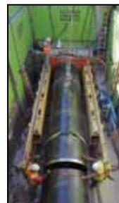
Cardno TBE recently completed the design of two major projects that included four trenchless crossings for Hillsborough County, Fla. The Duck Pond Phase I included microtunneling 350 ft of 60-in. steel casing pipe under SR582; and horizontal auger boring and pipe jacking 200 ft of 60-in. steel casing pipe under CSX RR. The SR 674 FM Phase 2 included two microtunnels of 450 ft and 300 ft of 48-in. steel casing pipe under I-75 and SR674.
