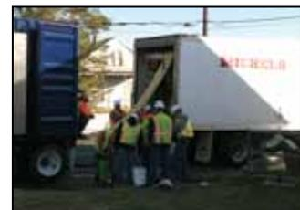
ft under six sets of active railroad tracks and had to be done without taking the tracks out of service. Michels installed a NSF 61-approved Class IV fully structural Nordipipe liner. A pressure vessel was used to invert the tube and it was cured with steam to a statically self-supporting pipe within a pipe. Each installation took 12 hours.
