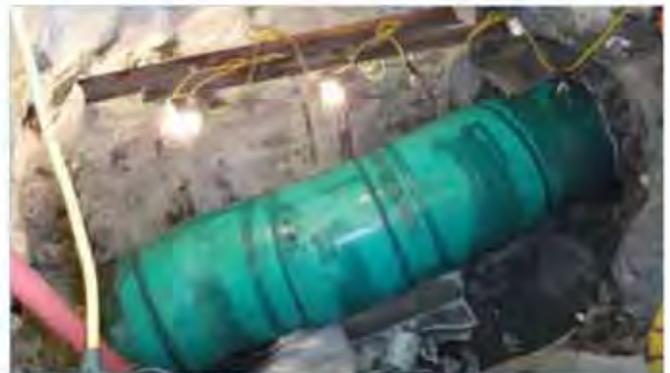
**Figure 4: The completed 36-in. diameter product pipe inside the frozen soil cavity.**
