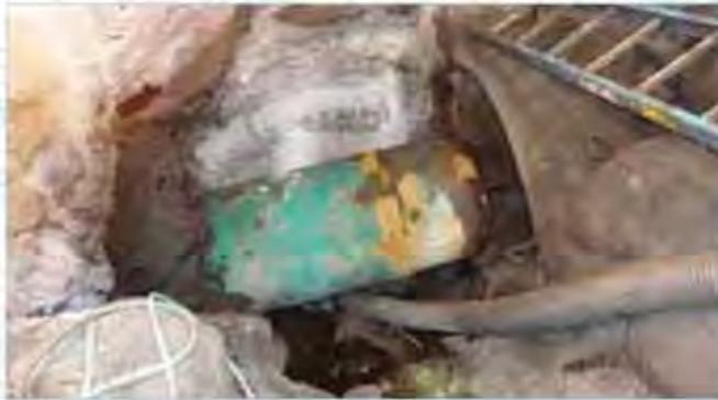
**Figure 3: Initial cavity around the product pipe (green) and casing prior to removal of the pull head and installation of the insulated tarps. Note the frost development on the back and upper face of the cavity.**
