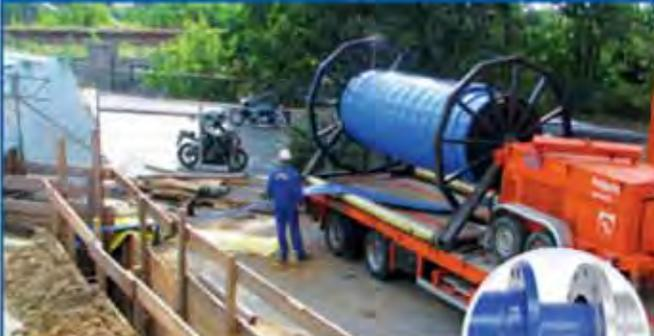
**Trenchless rehabilitation of pressure pipes**
