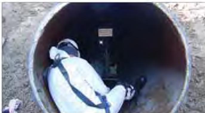
The electromagnetic inspection identified 58 pipe sections with electromagnetic anomalies out of approximately 10,000 pipes inspected, a distress rate of 0.6 percent (industry average is 4 percent). This project provides an example of how utilities can manage aging infrastructure while working within a tight capital budget, effectively extending the useful life of the asset. The project was awarded an honorable mention in *Trenchless Technology* magazine's Project of the Year awards.
