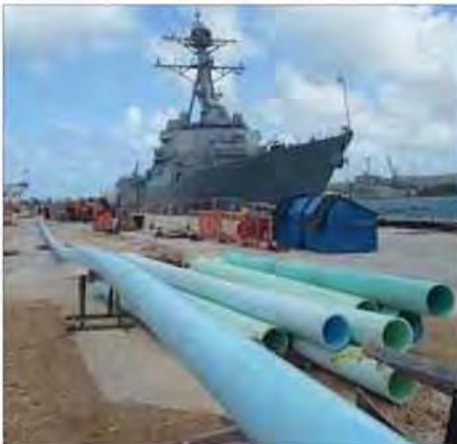
Fusible PVC pipe is now regularly designed and installed in Hawaii Department of Transportation (HDOT) right-of-ways (airports, harbors, and highways), under major roadways, including H3, Kamehameha Highway and beneath Dillingham Airfield.
