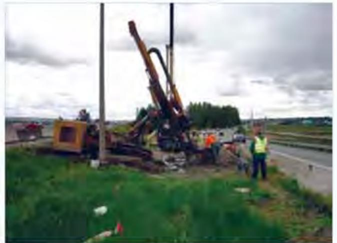
**Figure 2: Drilling and freeze pipe installation for the shaft bottom (looking south). I-5 is to the left and the off-ramp is located to the right.**
