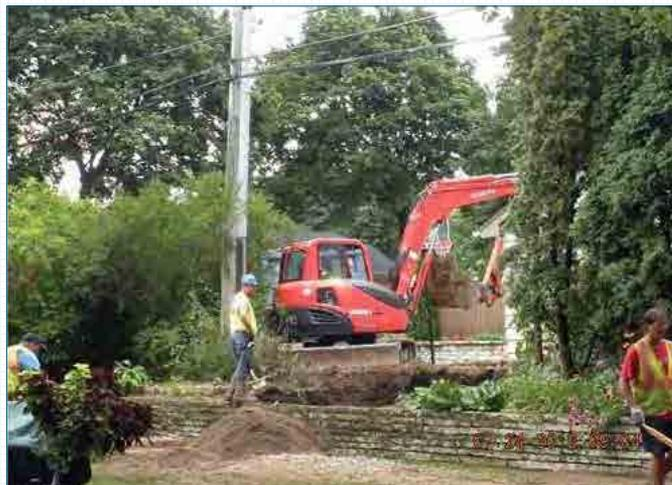
Figure 6 – Excavation in Wauwatosa after the Sept. 15, 2012 pipe break. The pipe runs parallel to, and behind, the retaining wall. Note the limited access along this pipe easement and the presence of overhead private utilities.
