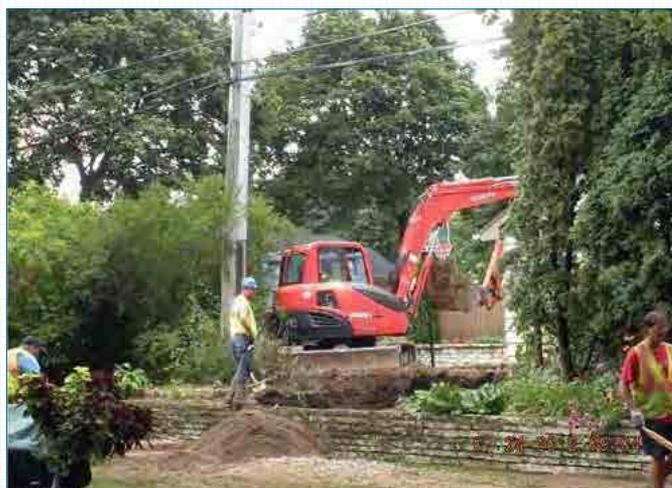
**Figure 6 – Excavation in Wauwatosa after the Sept. 15, 2012 pipe break. The pipe runs parallel to, and behind, the retaining wall. Note the limited access along this pipe easement and the presence of overhead private utilities.**
