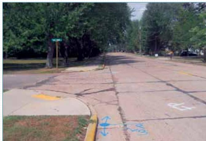
Figure 1 - Palmetto Avenue where it is intersected by Wallonnie Drive. The pipe varies in location from under the curb to near the middle of the lane in the foreground. Excavation would disturb much of the pavement.
