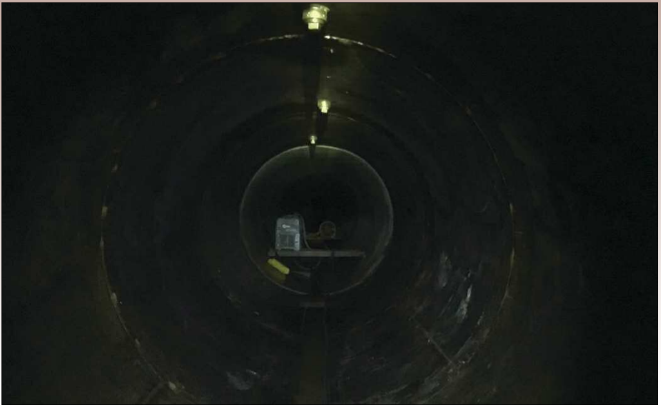
Figure 5. Repaired pipe section prior to mortar placement
