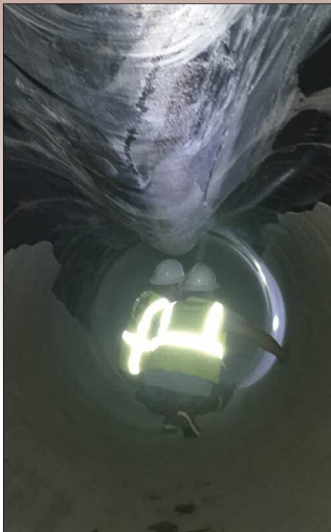
Figure 3. Initial buckled pipe damage
