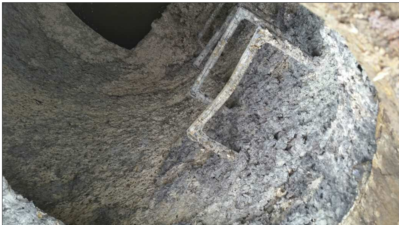
Figure 2. Manhole condition prior to rehabilitation
