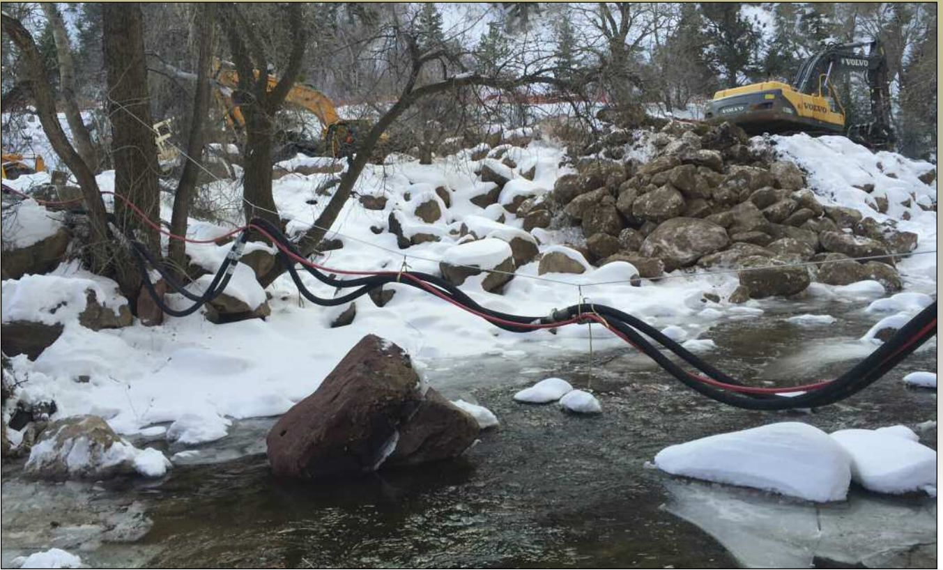
CIPP installation hoses suspended over creek
