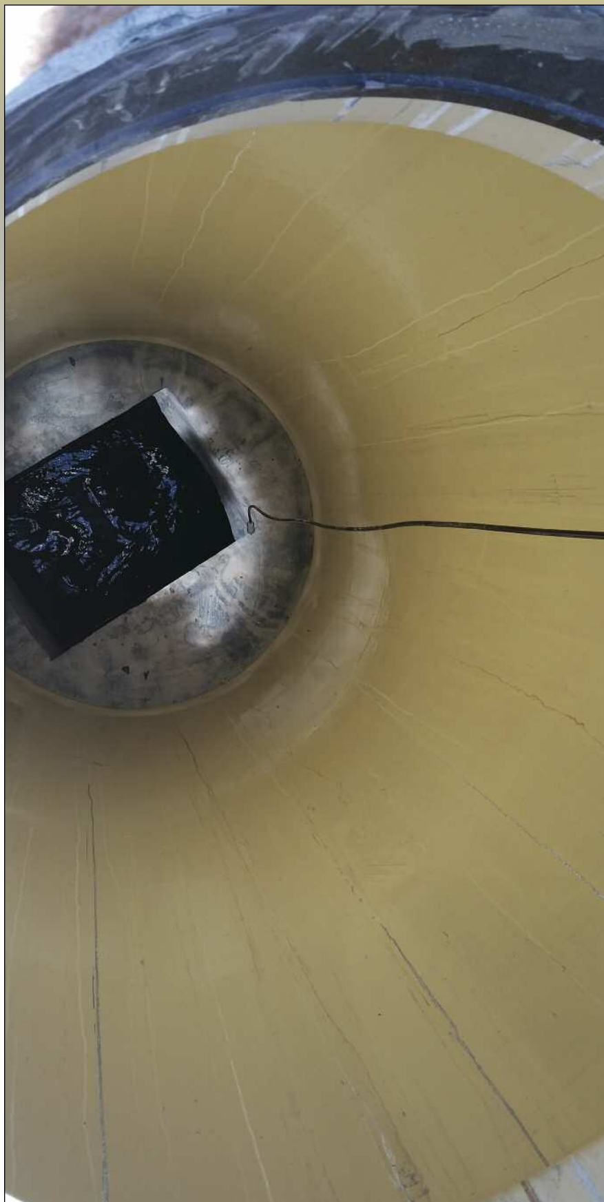
Figure 4. Completed composite manhole insert rehabilitation installation
