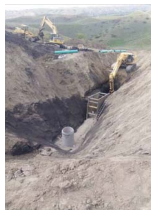
Figure 9. Second Manhole Installed
