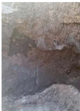
Figure 7. Corroded Manhole Barrel
