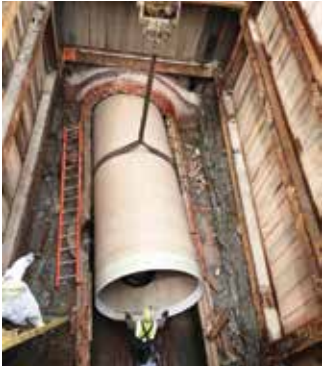
Figure 11 – Sliplining Pipe Placement
