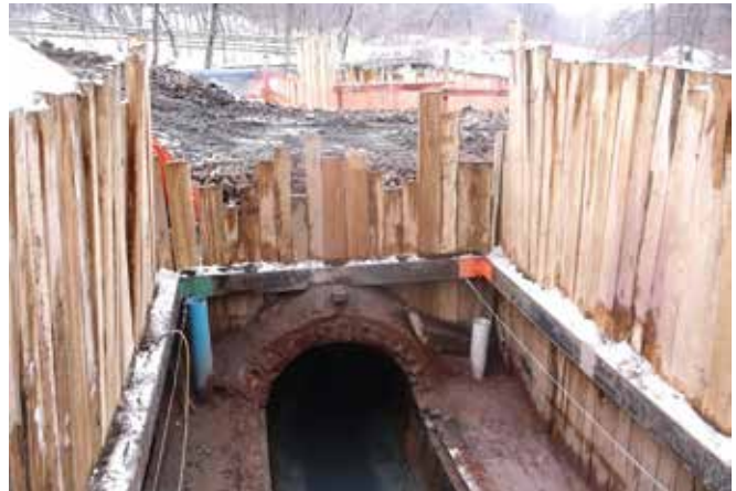
Figure 9 – Trench Shoring and Protection
