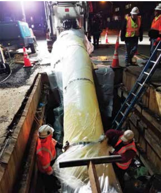
Starline® Cured in Place Liner coming off the drum guided as it enters the host pipe
