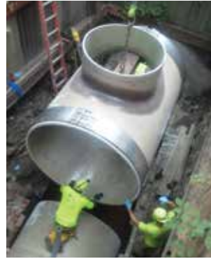
Figure 13 – Coupling to Sliplined Pipe After Annular Space Grouting
