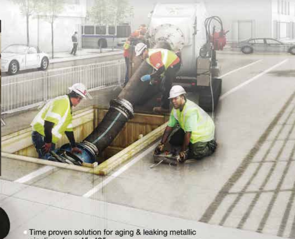
PPM / Starline holds the world record for the largest gas main ever lined. 36" Cast Iron Main, Seton Hall, NJ, November 2017
