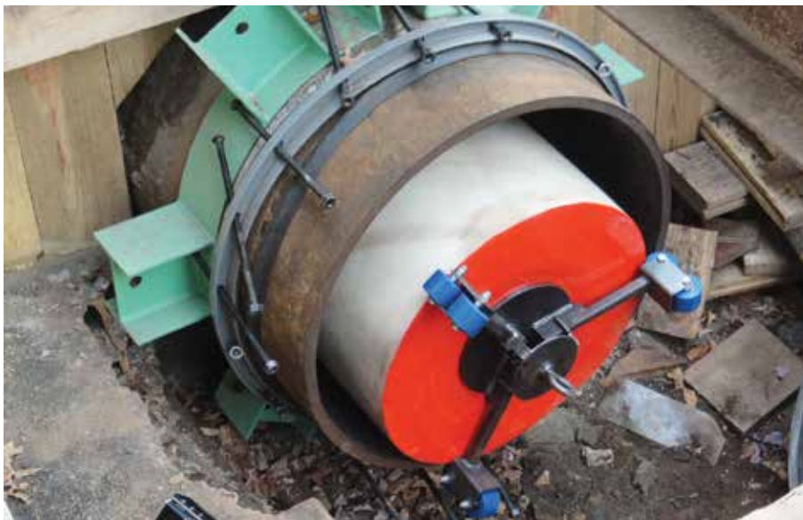
Custom pig fabricated to remove stranded grit
