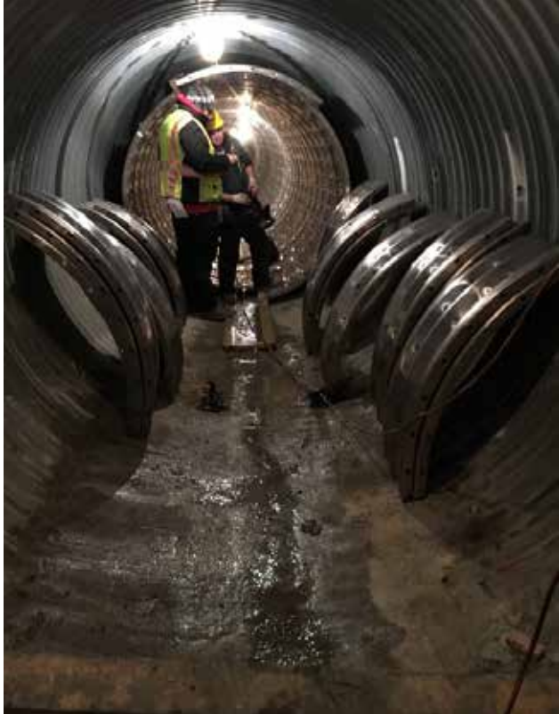
Individual sections were assembled inside the host pipe; 5 plates for each pipe ring
