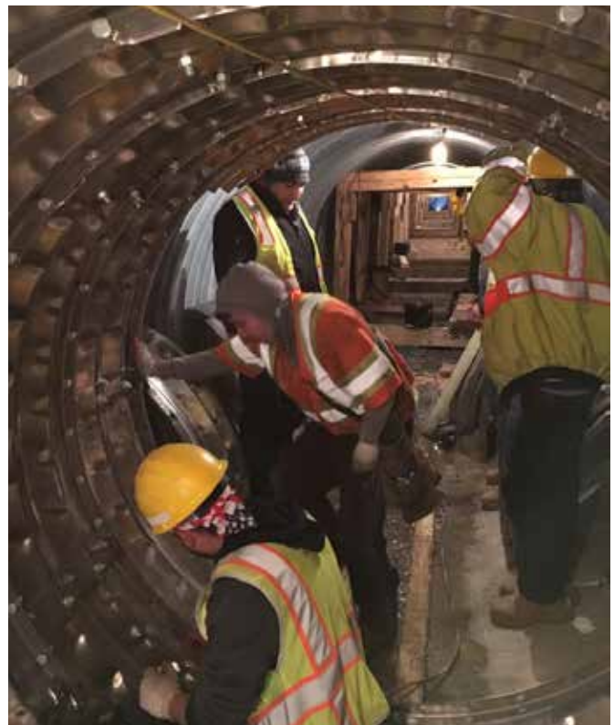
Tunnel Liner Plate provided a safe working environment as workers progressed through the length of the structure
