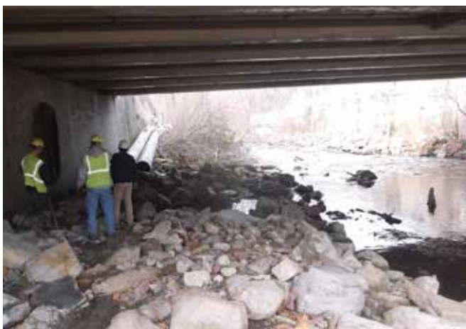
Figure 7 – Bypass Piping Crossing Under Howard Street Bridge
