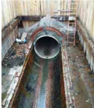
Figure 12 – Sliplining Pipe After Annular Space Grouting
