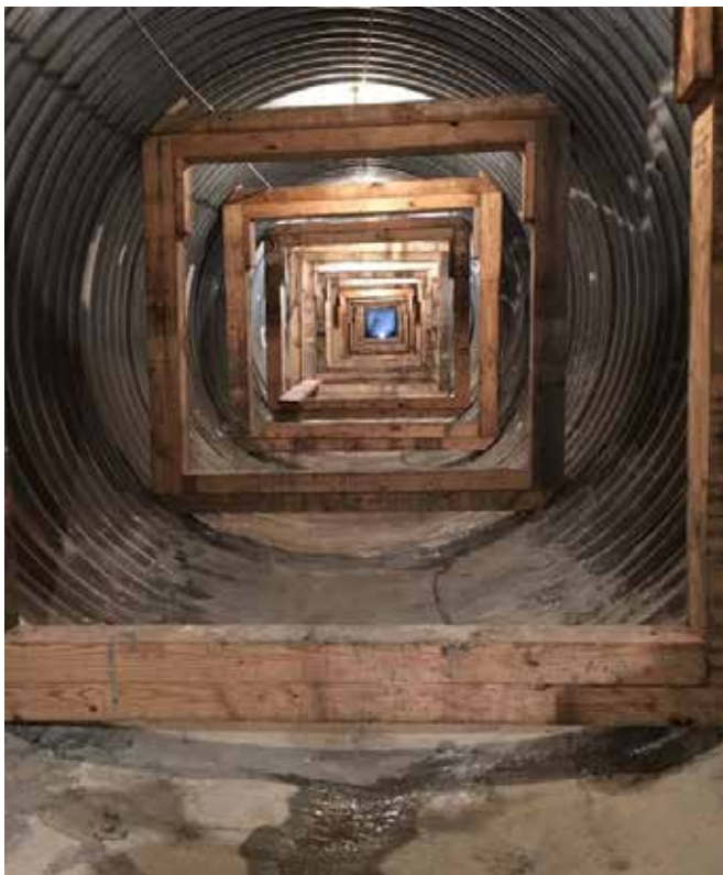
Host pipe stabilized with box beam frames to temporarily address structural concerns
