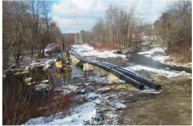
Figure 8 – Bypass Piping Crossing Ohio Canal near LCR
