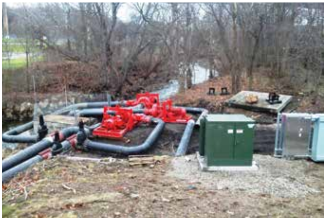
Figure 6 – Bypass Pump Setup
