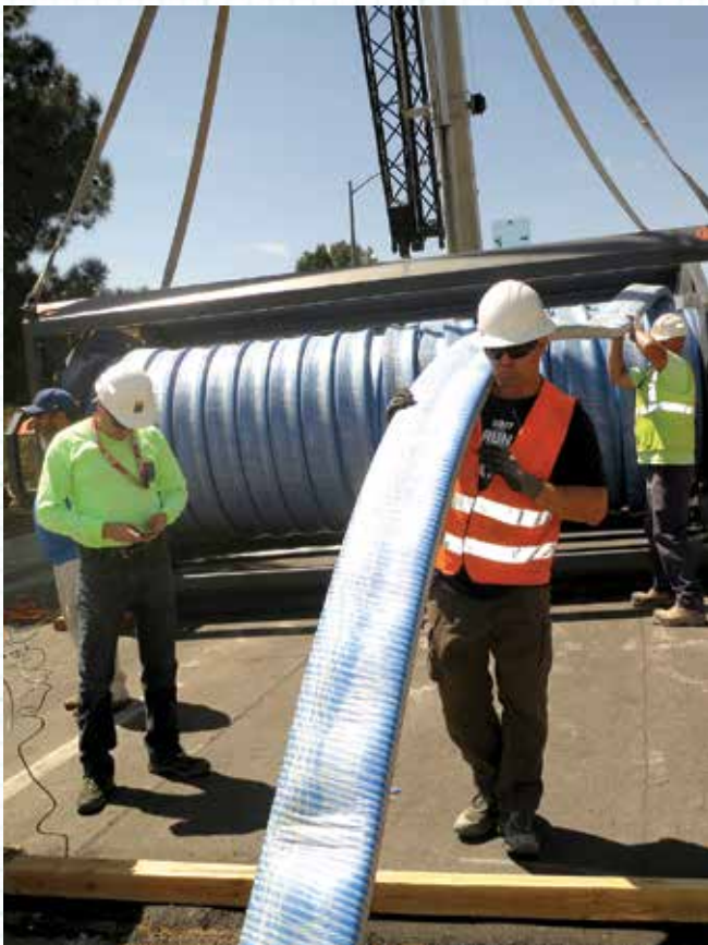
Crews Guide the Liner into Place for Installation on Reclaimed Line
