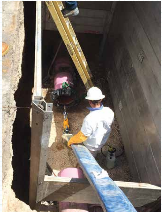
Reclaimed Pipe Liner Installation
