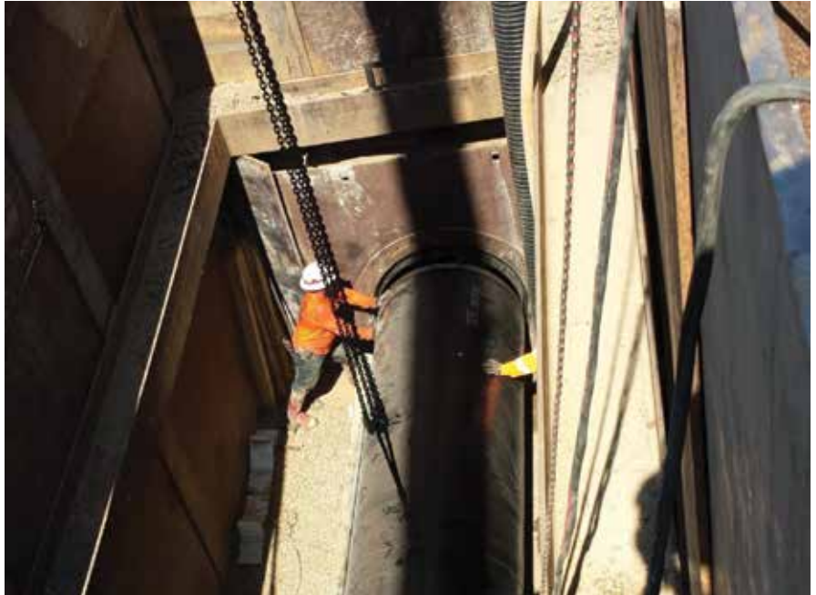
Figure 6. Pushing on a Joint for Casing Pipe in the Jacking Frame at Line A.
