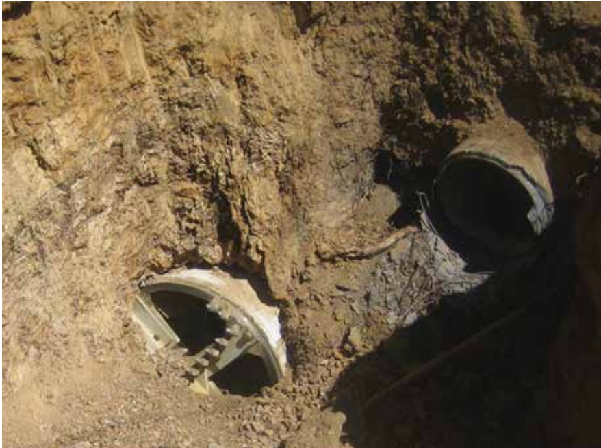
Figure 5. Line B TBM Shield and Cutterhead Being Retrieved From Excavation.
