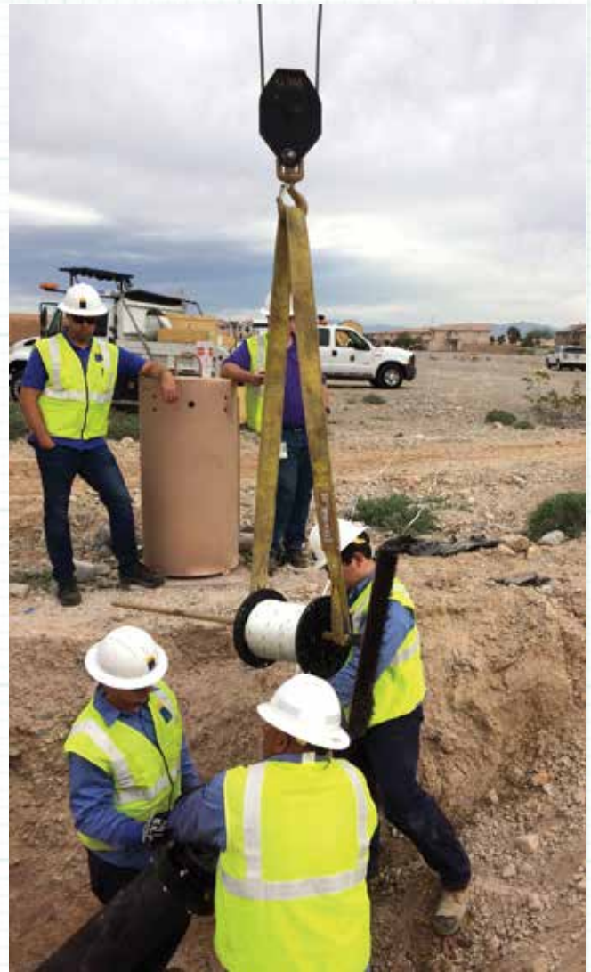
Crews Prep the Pipeline at Portal 1 for Liner Install at Highway Location
