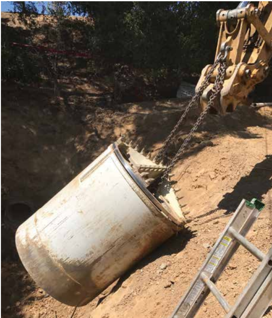
Figure 5. Line B TBM Shield and Cutterhead Being Retrieved From Excavation.
