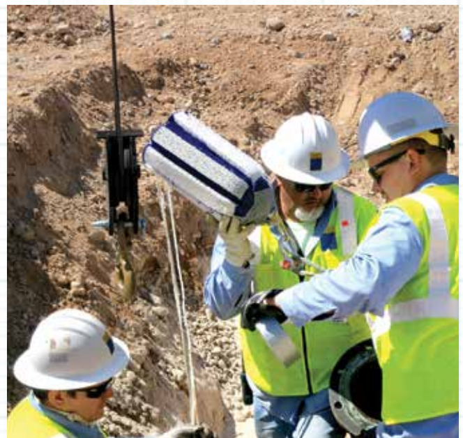
Crews Prepare to Pig the Pipeline for Line Installation at Highway Location
