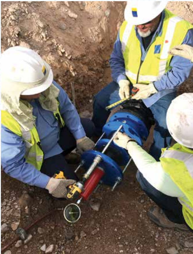
Crews Install 8-Inch Terminal Fitting at Portal 2 Highway
