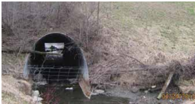
Figure 1. Upstream end of culvert, before construction.
