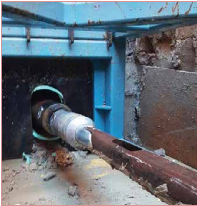
Figure 11. The low profile of the Quicklock bursting rods allowed Avertex to rod the existing PVC line, even though it had collapsed significantly.
