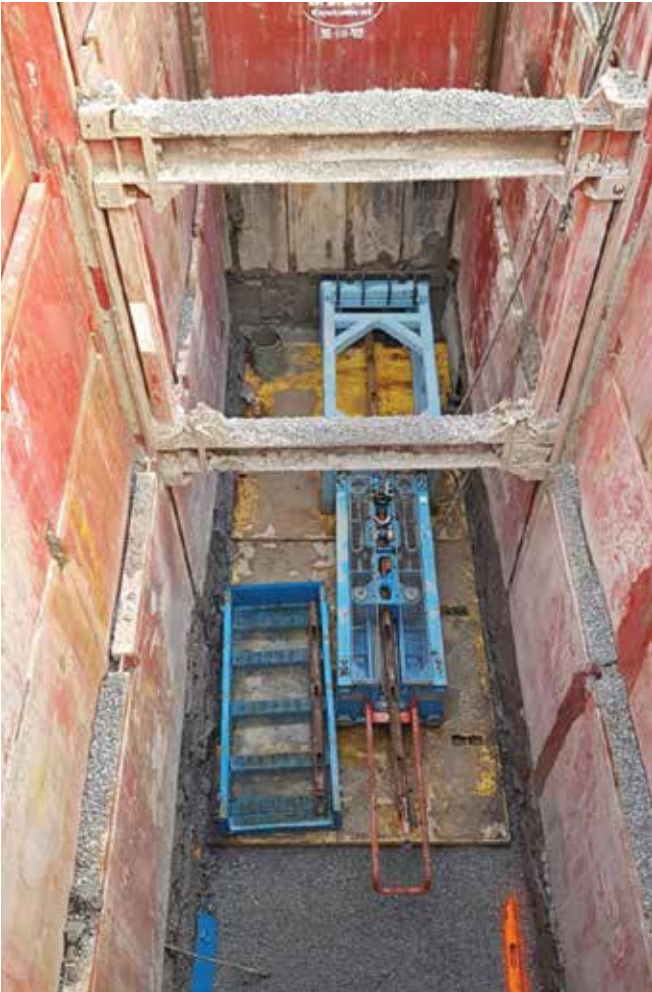
Figure 9. A static pipe bursting unit was used to burst and replace the collapsed PVC pipe.
