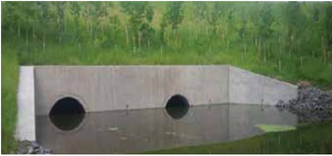
Figure 7. Upstream end of culvert, after construction.
