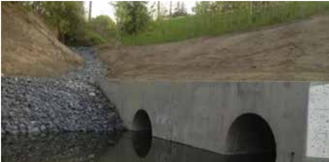
Figure 8. Downstream end of culvert, after construction.
