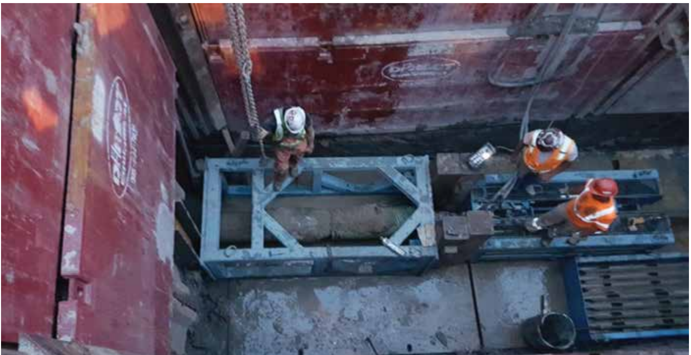
Figure 12. An extension frame on the pipe bursting unit provides the space between the wall of the shaft and the machine to facilitate the entry of the new pipe.
