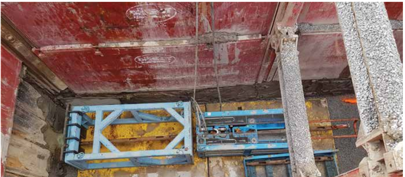
Figure 10. The static pipe bursting unit delivers 214 tons (427,137 bar) of pullback.
