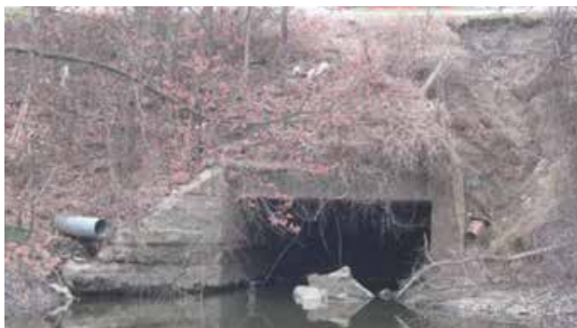
Figure 2. Downstream end of culvert, before construction.
