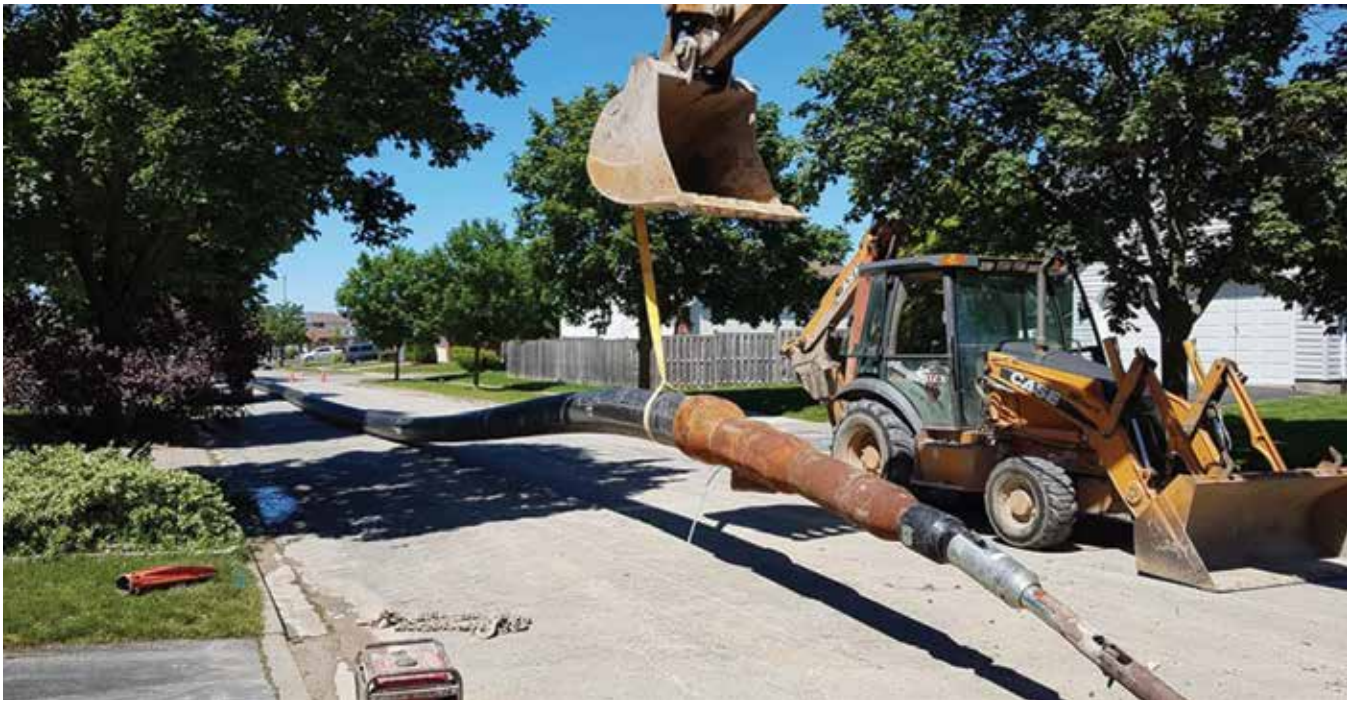
Figure 8. A directional drill was used to create a window down to the existing pipe on the launch side of the project. This allowed Avertex to limited street disruption and restoration.
