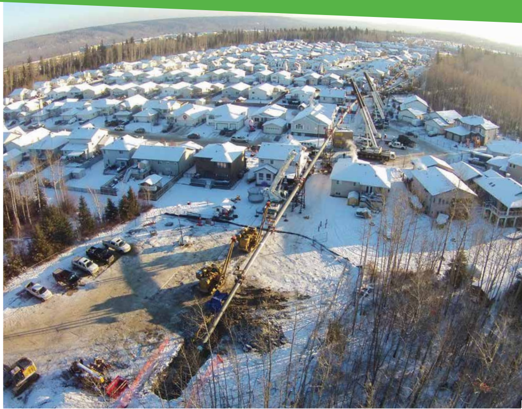
New pipeline provides Fort McMurray's south service area with a robust and resilient water supply network
