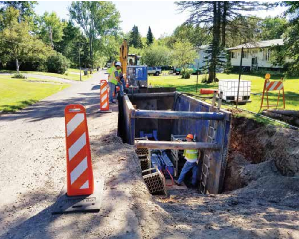
The city chose trenchless pipe bursting to limit disruption on its narrow streets and neighborhoods
