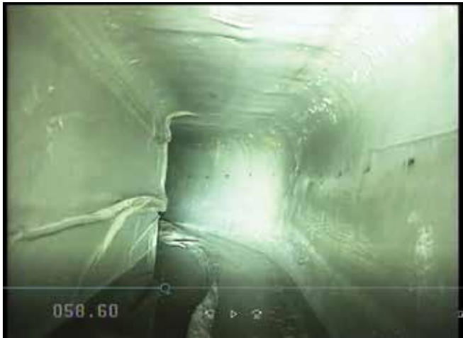
PST#1 post lining at a 45 degree bend
