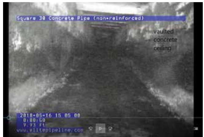
PST#1 conduit precast ceiling panels missing and vaulted
