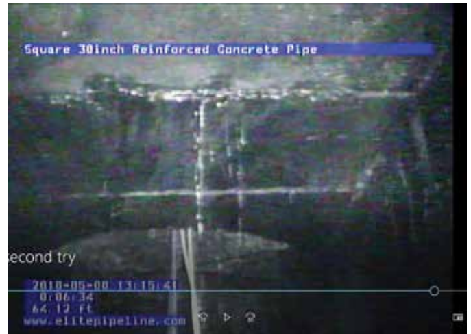
PST #4 influent tunnel televising existing conditions and the one point of infiltration/exfiltration
