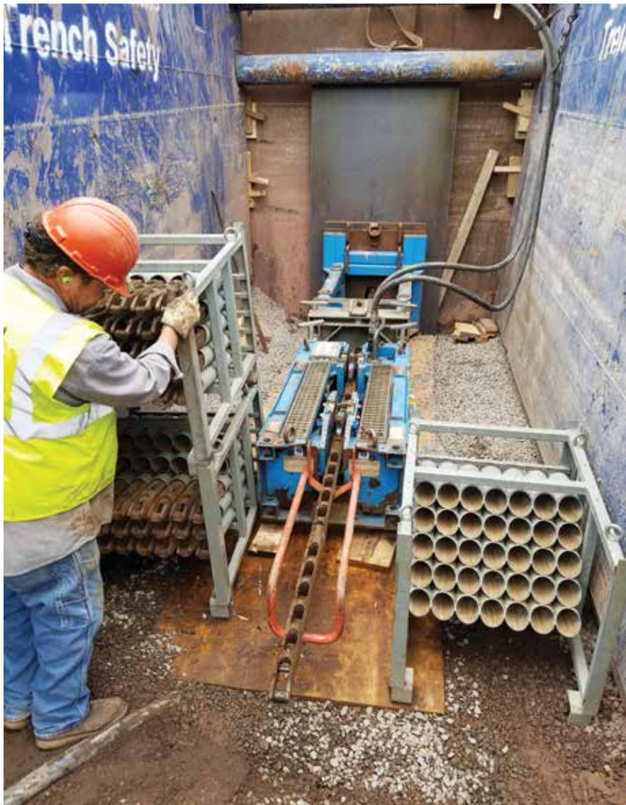
The City of Duluth developed an in-house pipe bursting program focused on replacing deteriorating cast iron water mains
