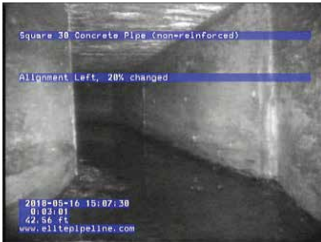
PST#4 influent conduit existing condition at 45 degree bend
