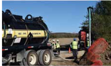
WATER MAIN CLEANING
