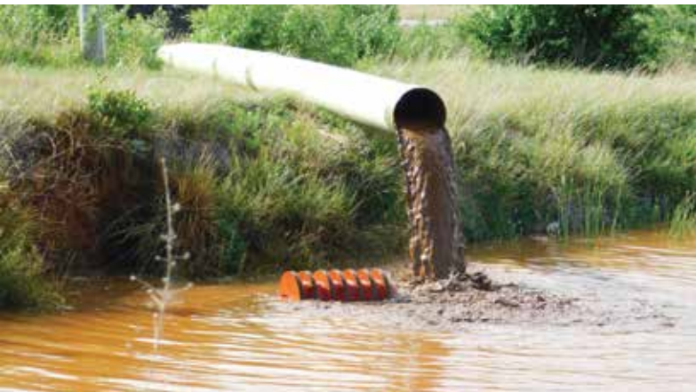
Replaced twin water mains after pigging was completed
