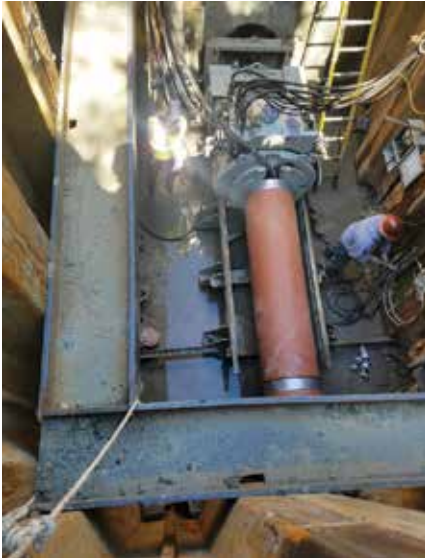
Pushing the product pipe into place
