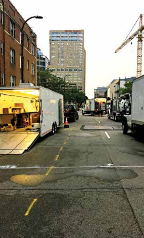
The sinkhole presented a major problem for the traveling public
