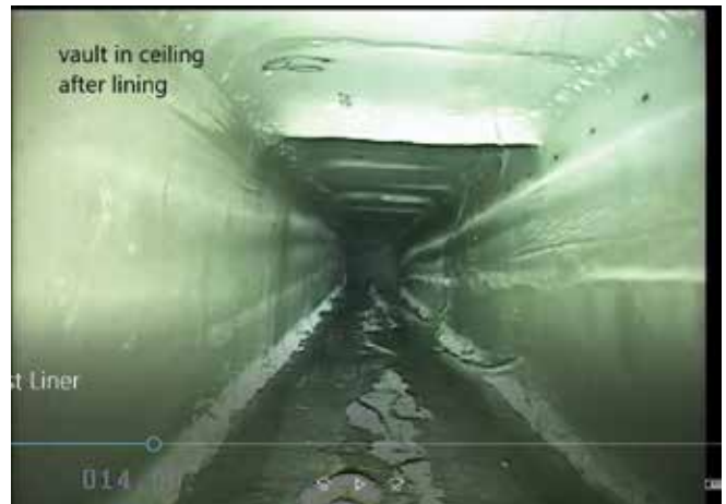
PST#1 conduit after lining
