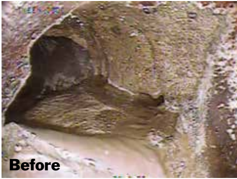
A unique CIPP rehabilitation of 18-inch oval main lateral connection
