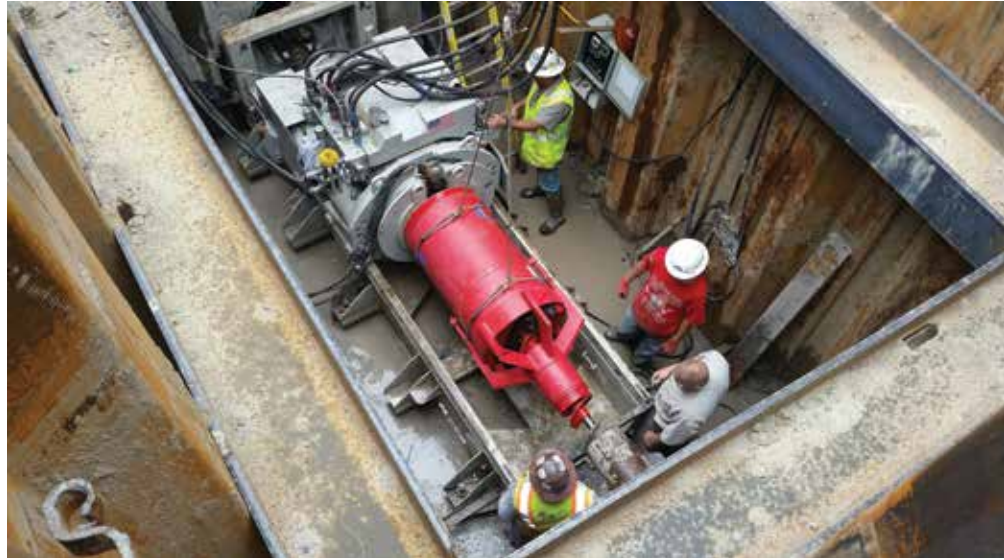
The Powered Reaming Head in place and ready to follow the path of the pilot tubes
