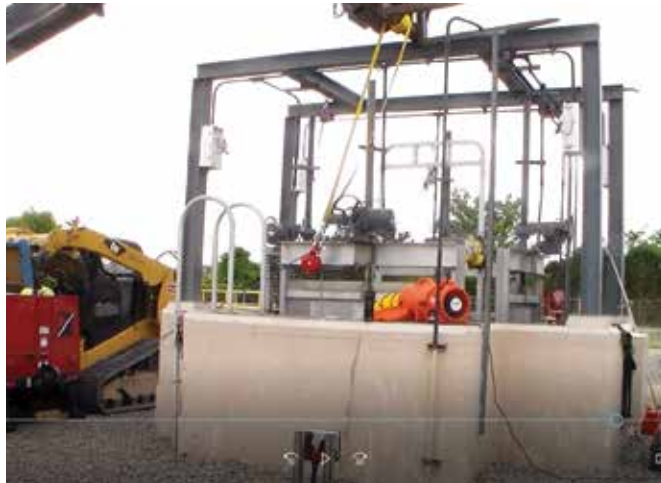
Winch set up at the distribution box to pull the liner into place
