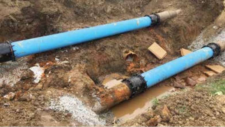
Disc Pig exiting the water main
