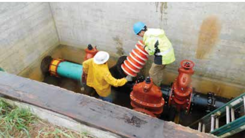
Disc Pig being inserted into one of the dual line water mains
