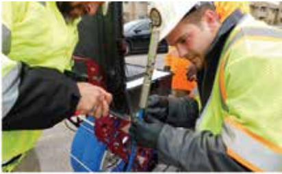
LIVE WATER MAIN INSPECTION & LEAK DETECTION
