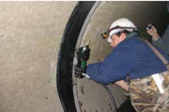
The system of installation requires technicians verify a proper sealing surface covering the joint, making repairs as necessary
