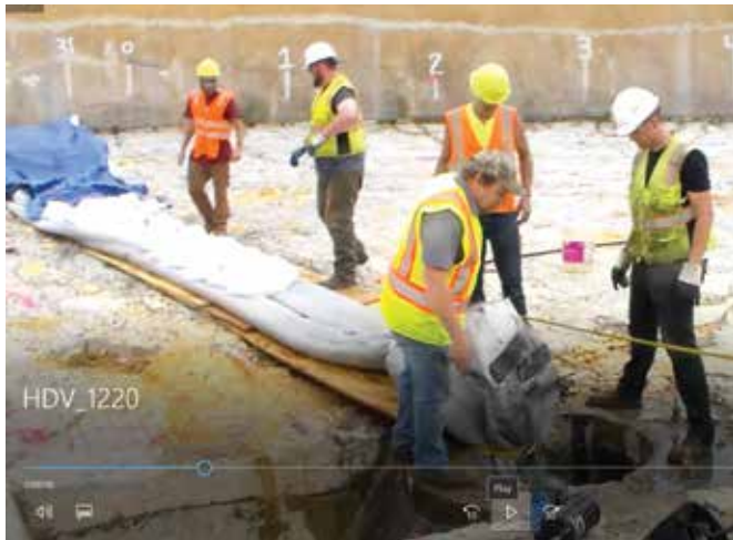
Liner being pulled into PST#1 Conduit
