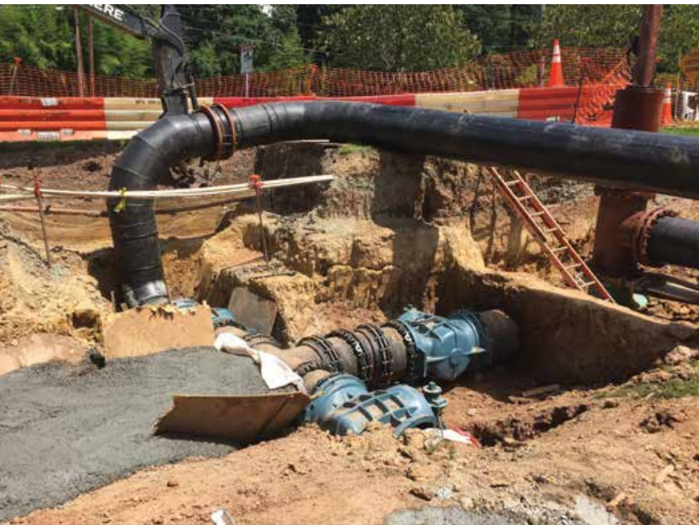
24-inch Tee and Plug Valves Installed Downstream of Line Stop
