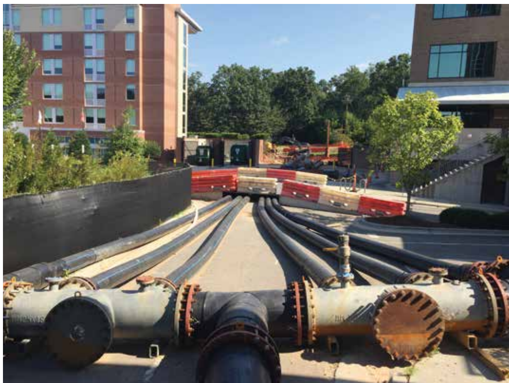
Concrete Road Ramp with six 12-inch HDPE Bypass Lines
