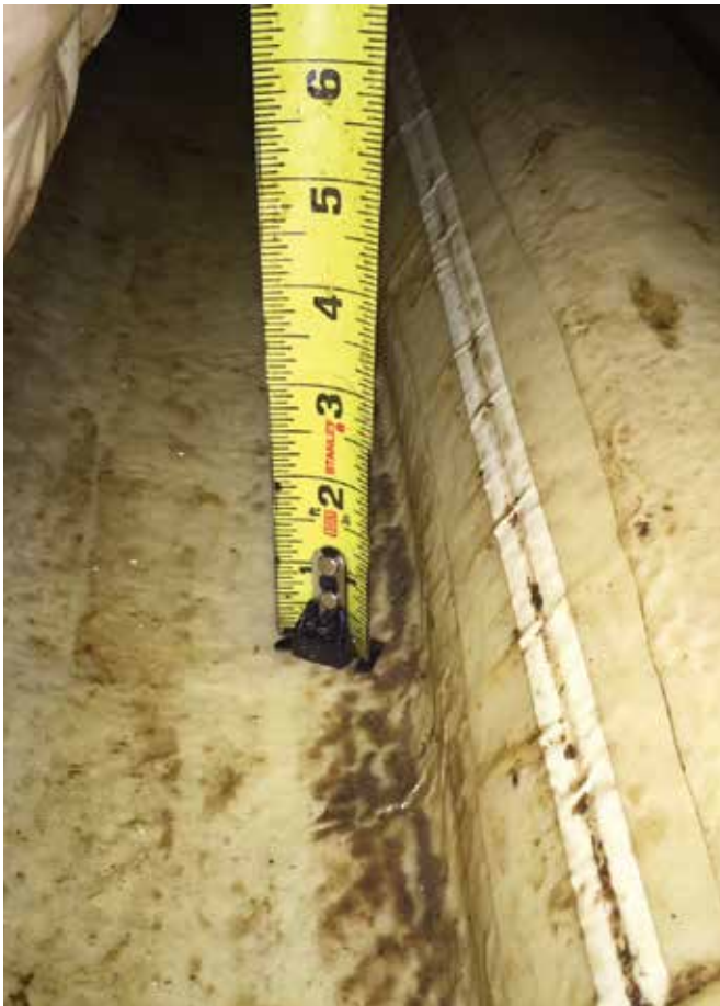
Trapped Water from Potential Infiltration in CIPP Liner
