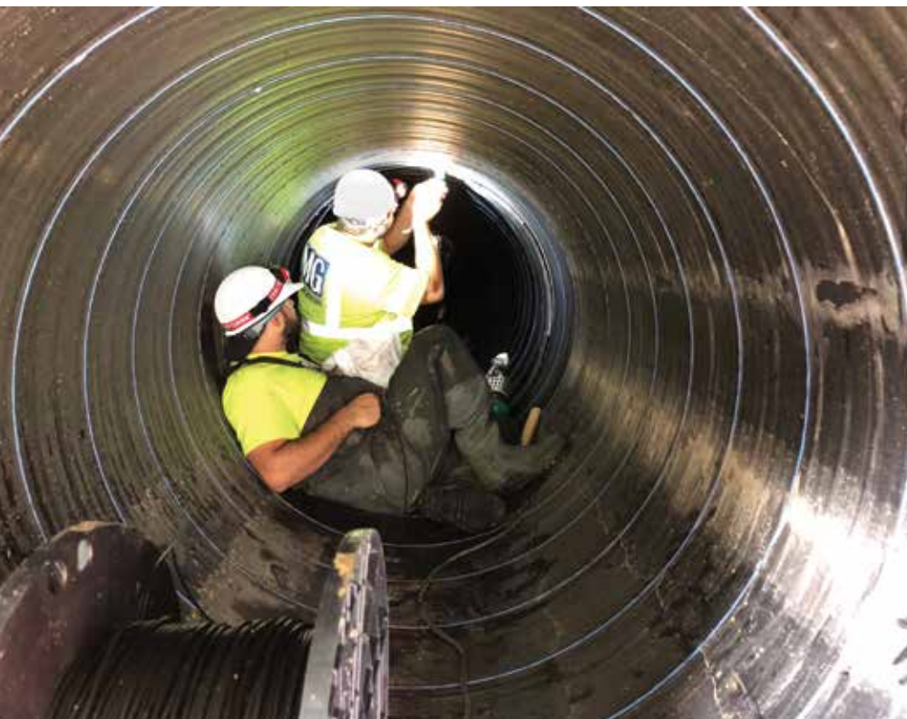
Welded Coupler (WC) joints were included in the design to provide a 30 psi, watertight joint
