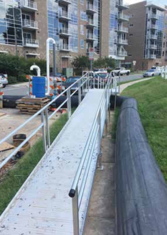
Pedestrian Ramp and Temporary Odor Control
