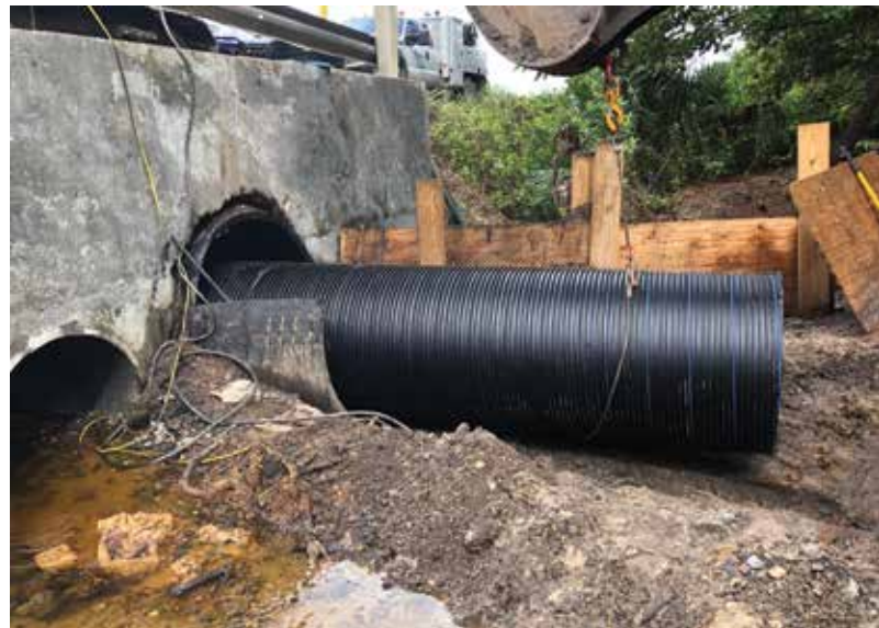
The DuroMaxx SRPE Liner Pipe offered a fully structural relining solution
