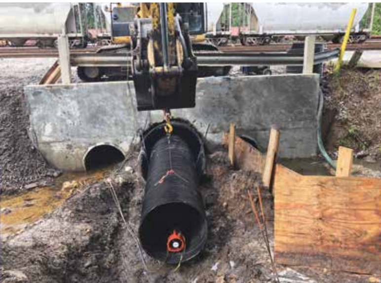
A push-pull method was incorporated to expedite the installation process
