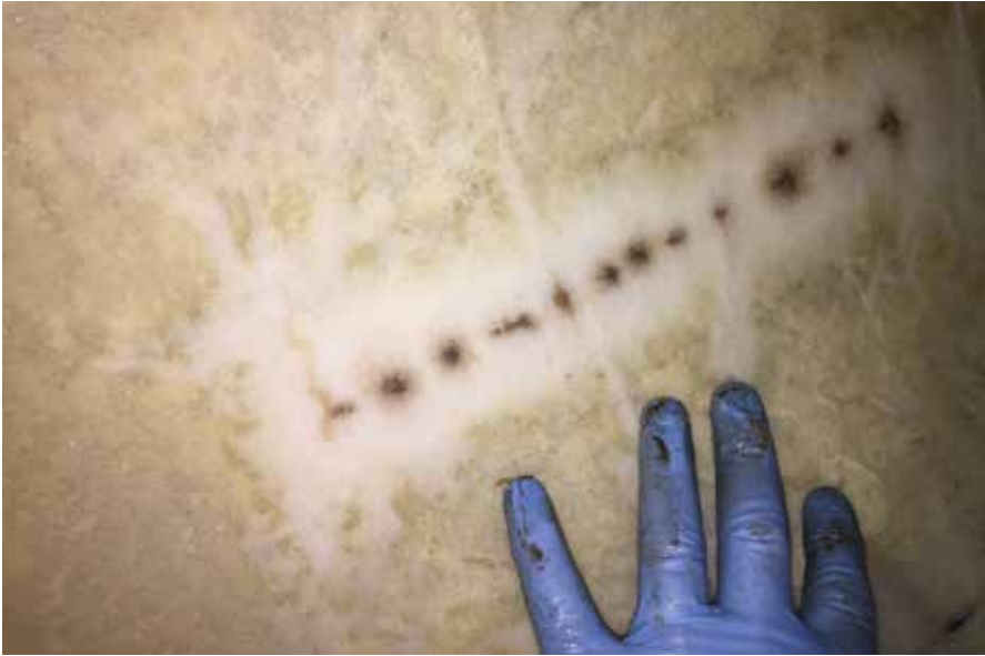
Holes in Second Partial Liner
