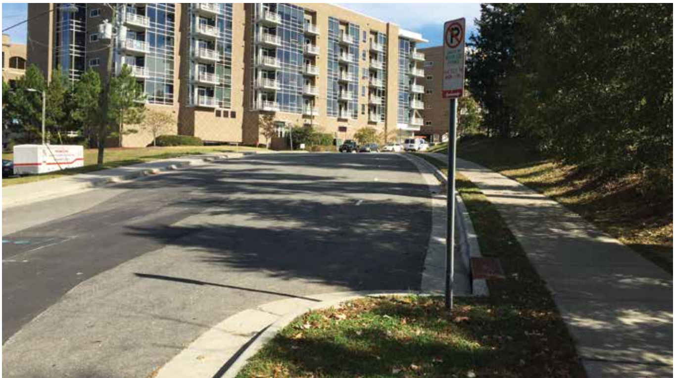
Area of Force Main Break in Secondary Street
