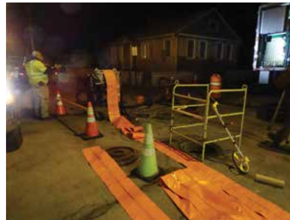
Using an epoxy CIPP liner was beneficial in 2017
