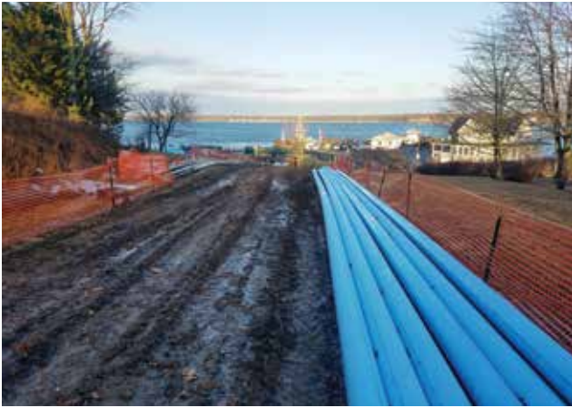
Work continues through winter to meet project schedule
