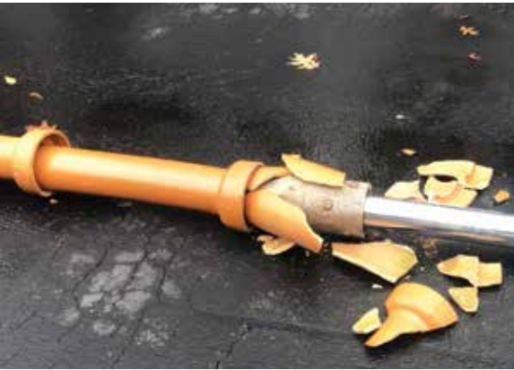
Figure 2: Pipe bursting live demo
