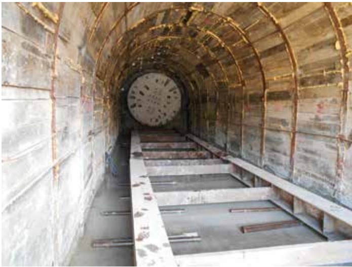
Figure 4: MTBM holed through into the hand-mined tunnel
