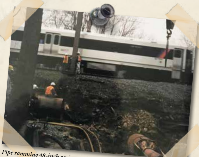
When directional drill is immobilized percussive power frees 2500 feet of 24-inch pipe with air hammer attached
