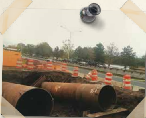
42-Inch Conductor Barrels - pipe rammer installs steel casings for clean bore start
