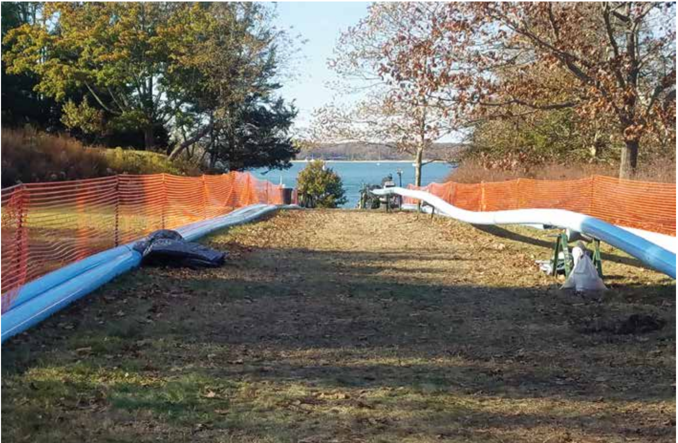
First of 3 conduits is pre-assembled for installation
