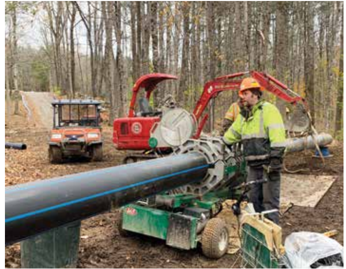
Fusing HDPE pipe string on site
