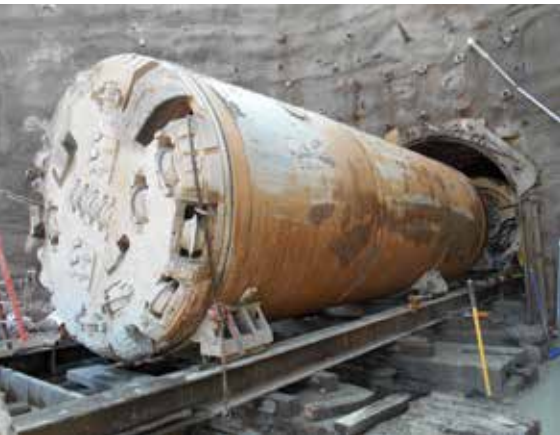
Figure 5: MTBM pushed through valve chamber portal
