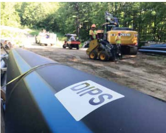
More than two miles of new 12-inch HDPE DIPS SDR11 pipe installed
