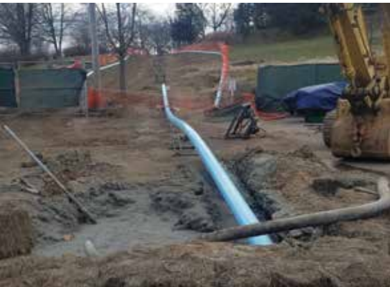
Insertion of first conduit is almost complete
