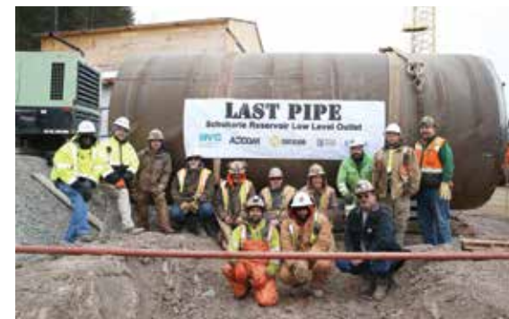
Figure 8: Commemorative last pipe to complete the LLO water leg tunnel
