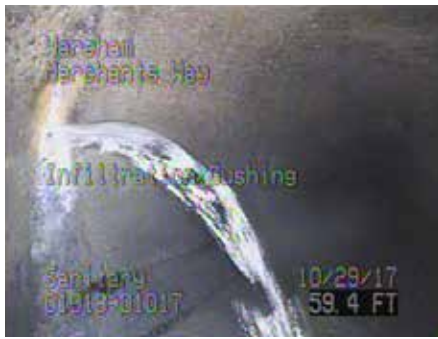
Infiltration at joint
