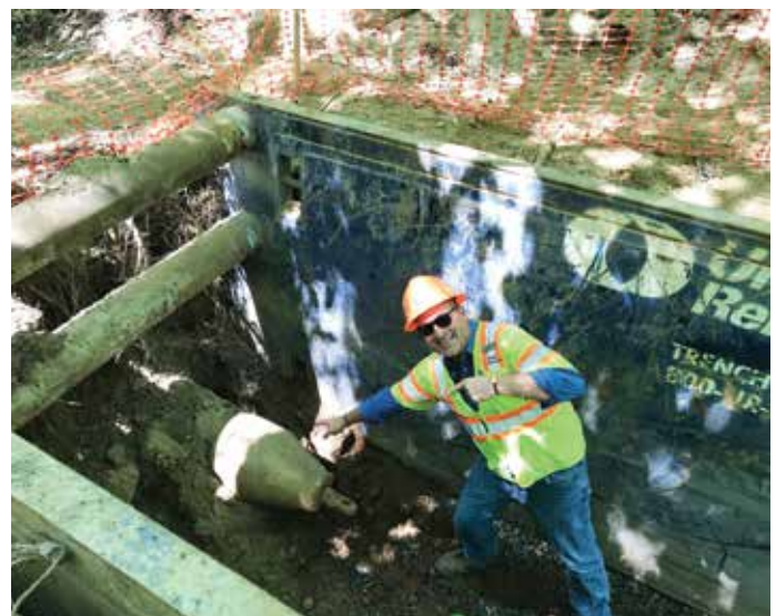
Ted Berry Company President Matt Timberlake at exit of another long pipe-bursting run
