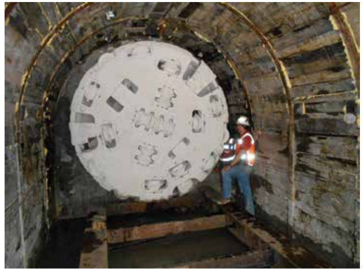
Figure 4: MTBM holed through into the hand-mined tunnel
