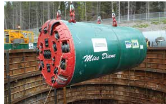
Figure 7: The Herrenknecht AVN2200B MTBM "Miss Diane" lowered to the land leg tunnel launching site
