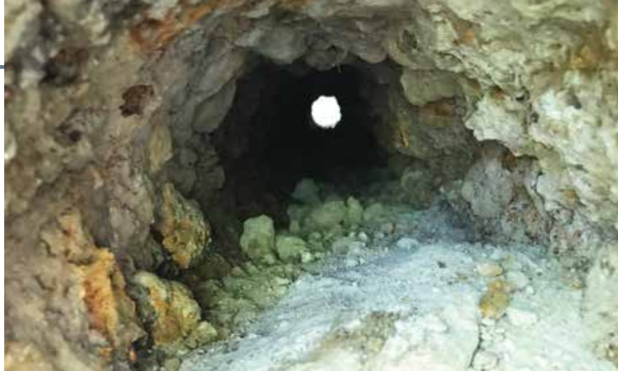
Original CI Main installed 120 years ago when McKinley was US President
