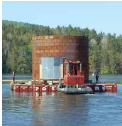
Figure 6: Water leg cofferdam structure with fiberglass soft eye
