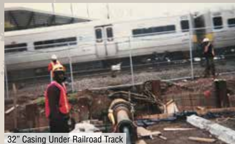
32" Casing Under Railroad Track
