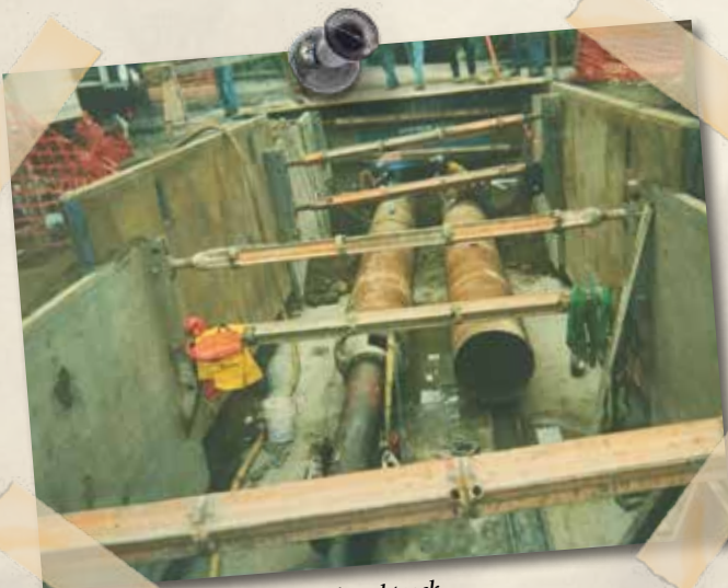
Two 30-inch casings under railroad track
