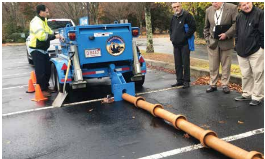
Figure 1: Pipe bursting crew and conference attendees witnessing the demo
