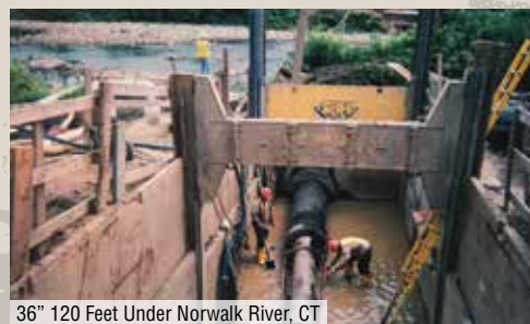
36" 120 Feet Under Norwalk River, CT
