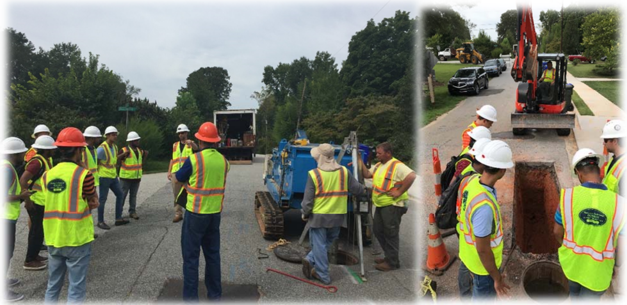
Pictures 6. (a) Jesse and his co-worker interacting with Clemson students at Pipe Bursting jobsite; (b) Students watching the existing pipe in the entry pit of pipe bursting
