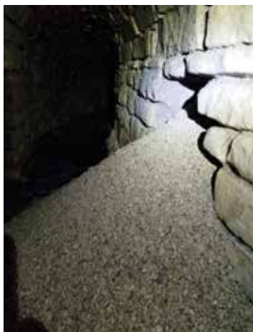
Figure 5. A cave-in during pipe plugging operations caused a void to form under the roadway
