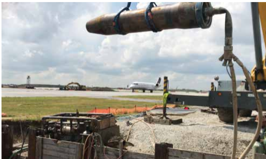
Extensive shoring was required
