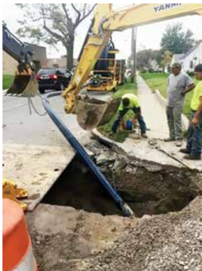
HDD used to install six-inch diameter water main from 500 foot reels. City crews have become skilled with electrofusion
