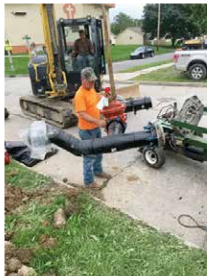
HDD used to install six-inch diameter water main from 500 foot reels. City crews have become skilled with electrofusion
