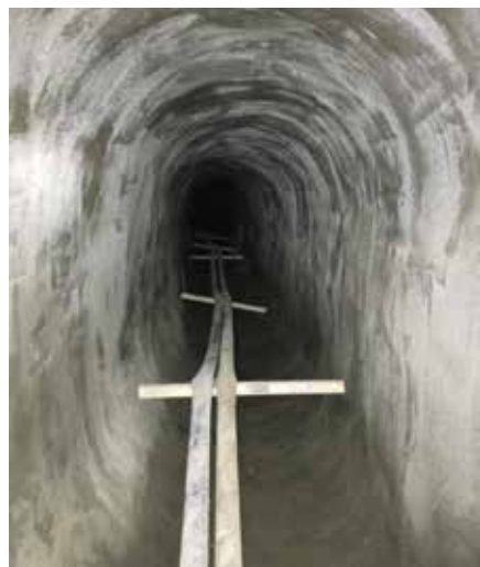
Figure 7. The archway sewer after the geopolymer coating was applied. Bypass pumping lines also shown
