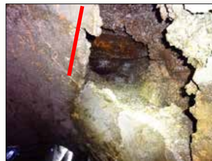
(d) Looking into void (downstream), approximately 10 feet deep.
