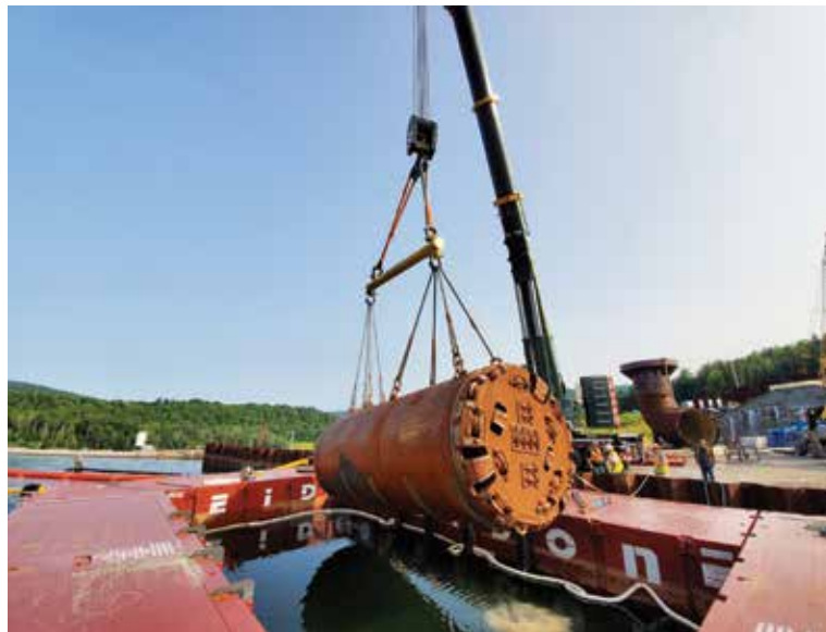
Figure 6: The MTBM unit was retrieved from a depth of approximately 153 feet on July 10, 2019
