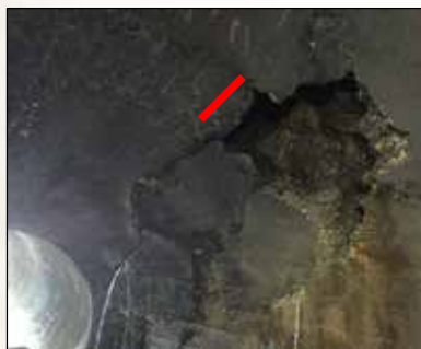
(c) Defect after dewatering and minor scaling for safety.
