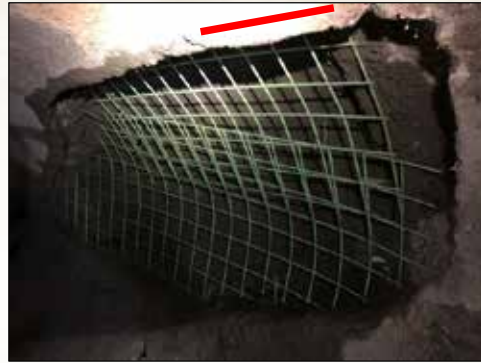
(f) Welded wire mesh in place during shotcrete repair.
