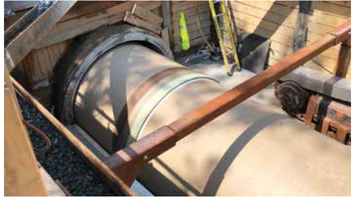
New pipe in-place
