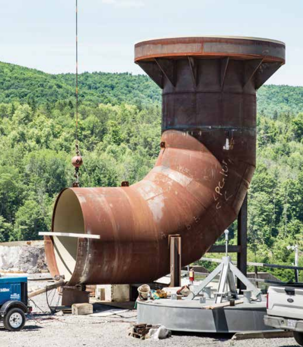
Figure 7: 108-inch elbow for the intake. In foreground is removable plug/bulkhead used for dewatering water leg tunnel
