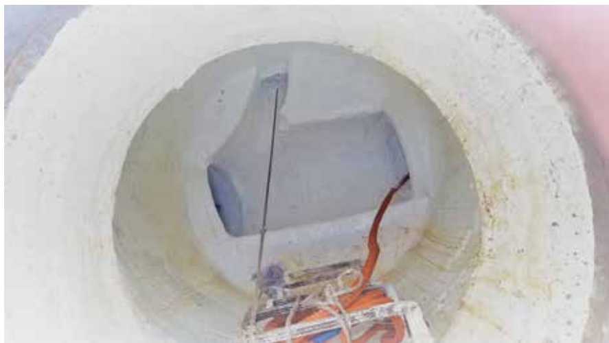
The 39 manholes along the 1.8 mile segment were coated with an aquatic-safe epoxy
