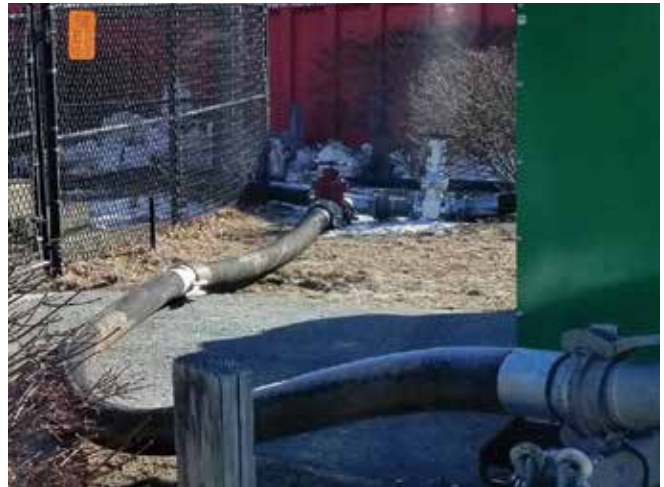
Bypass setup pumped over 110,000 gallons average daily flow
