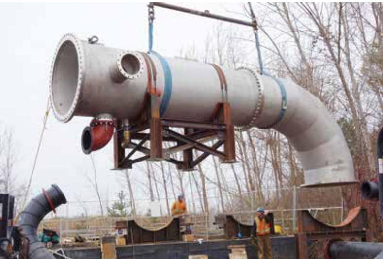
Figure 2.60-inch launcher being moved from one intake to another
