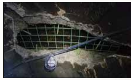
(c) Welded wire mesh in place for shotcrete repair.
