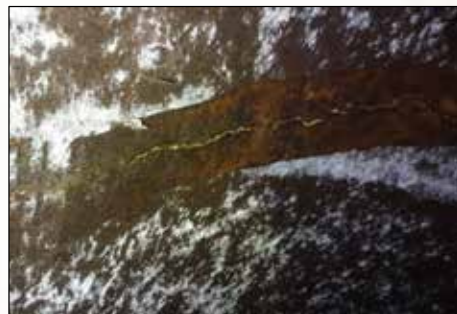
(b) Defect after dewatering.
