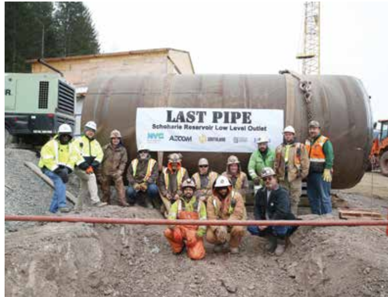
Figure 4: Commemorative last pipe to complete the LLO water leg tunnel
