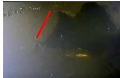
(b) Defect during 2017 Emergency ROV Inspection.
