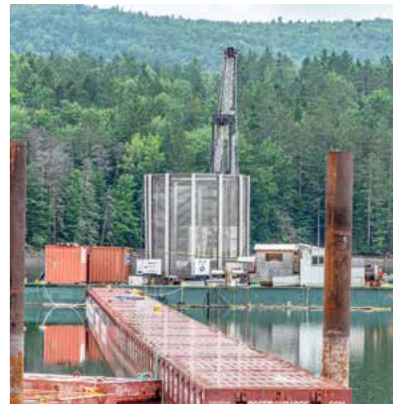
Figure 9: The stainless steel Intake Structure was lowered into place and tremie concreted
