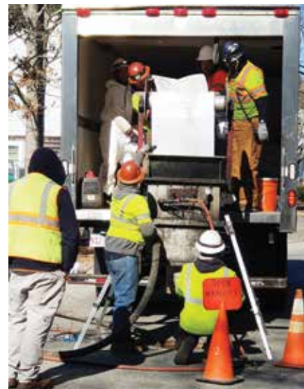
Compact site footprint during liner installation minimized impact on the community
