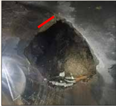
(e) Defect after sawcutting and chipping in preparation for repair.
