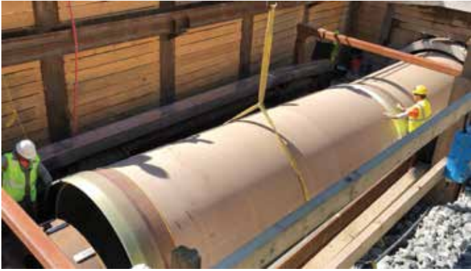
Installation of a slipliner into an excavated pit
