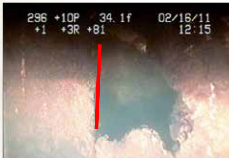
(a) Defect during 2011 ROV Inspection (SeaView, 2011).
