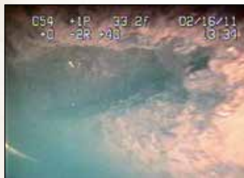
(a) Defect during 2011 ROV Inspection (SeaView, 2011).
