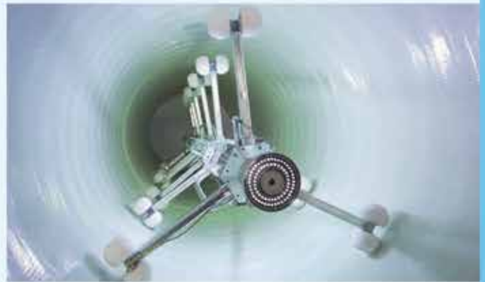
UV Mainline Lining
