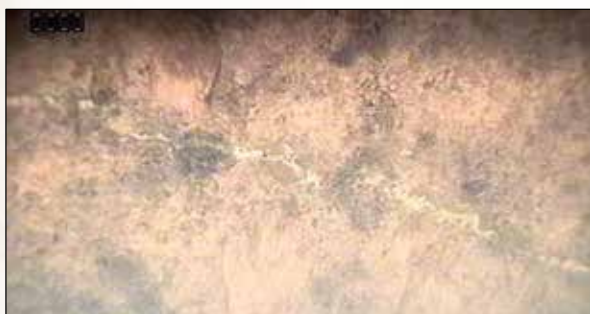
(a) Defect during 2011 ROV Inspection (SeaView, 2011).
