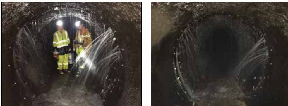
Figure 3. Before and after chemical grouting on the left arch.
