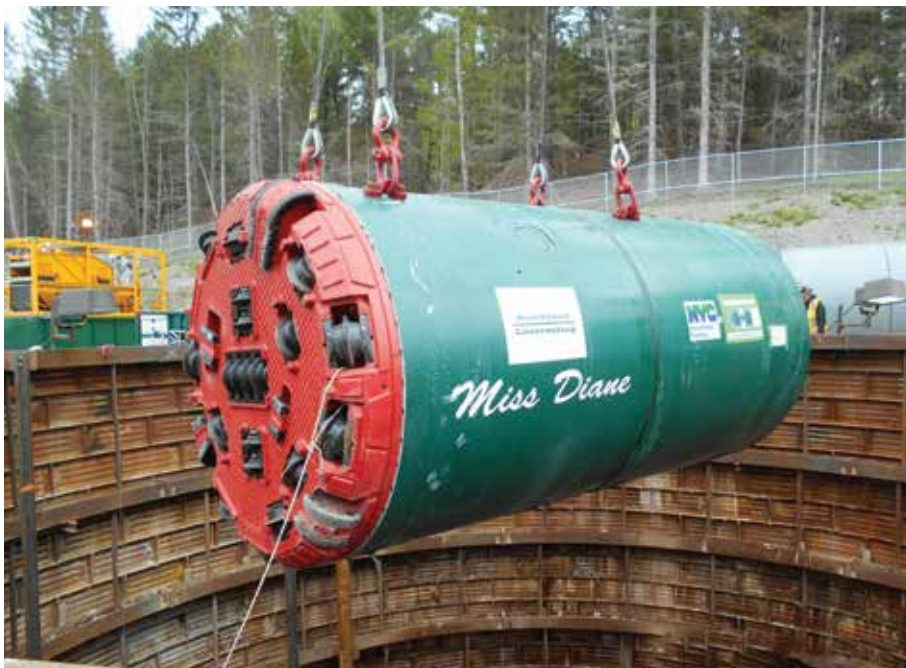
Figure 1: The Herrenknecht AVN2200B MTBM “Miss Diane” lowered to the land leg tunnel launching site. The first of its kind manufactured in accordance with OSHA Class I Division II classification
