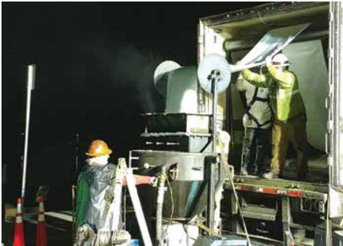
To reduce traffic disruption in downtown Wareham, CIPP liner was installed at night
