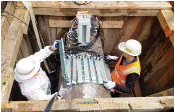
External NDT inspection of exposed CI pipe
