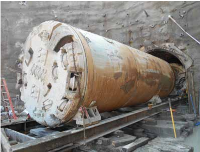
Figure 3: MTBM pushed through Valve Chamber portal to complete the land leg tunnel
