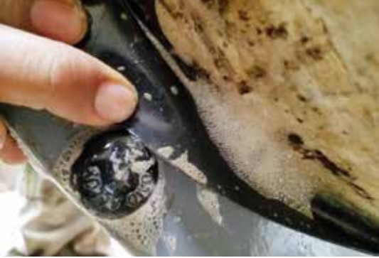
Leak at CI coupling
