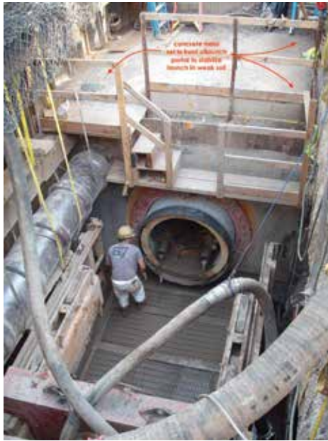
Figure 3- Photograph of MTBM launching shaft depicting the use of concrete mass ground stabilization in front of launch portal to stabilize weak soils.
