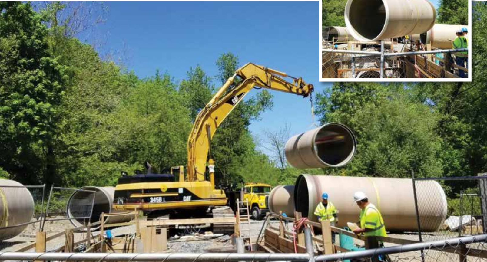
Lifting of a pipe section using an excavator onsite
