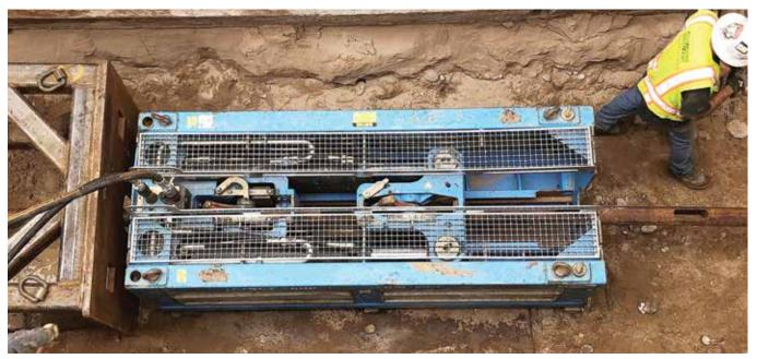
To complete the 100 percent upsize from 8-inch VCP to 16-inch FPVC, AUI used a Grundoburst static pipe bursting system from TT Technologies.
