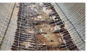
Figure 3. Nelson Stud and Wire Mesh Prior to Invert Concrete
