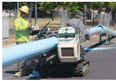
Figure 8: Fusing PVC Pipe and Sliplining the Casing Prior to Pullback
