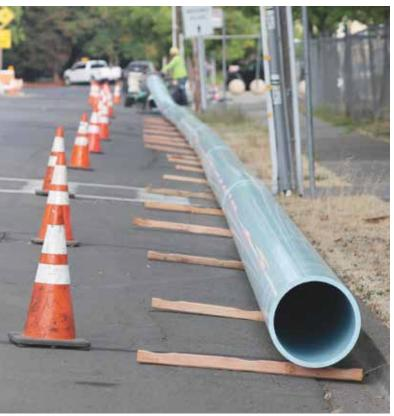
Figure 7: Pipe String in Temporarily closed parking lane
