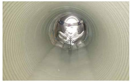
Figure 6. A first pass of mortar in a pipe section.
