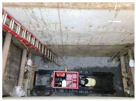
Shafts constructed using trench boxes due to low groundwater and stable ground conditions
