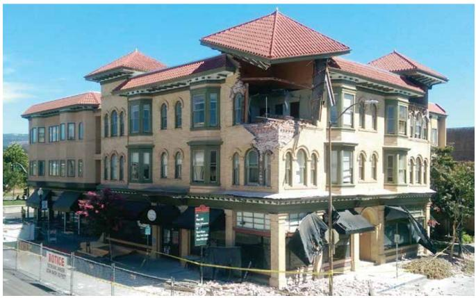
Figure 3: Damaged Alexandria Square building in Napa
