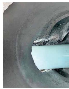
Bursting runs were determined by manhole location. Longer runs included bursting through a manhole and onto to the next.
