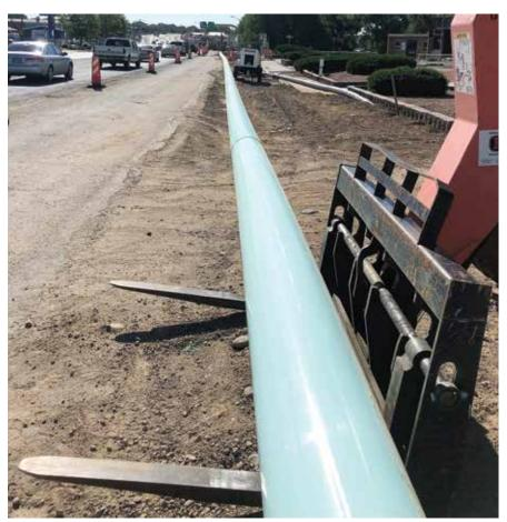
*Fusible PVC was chosen to replace the existing VCP sewer. The static pipe bursting process can accommodate a wide range of product pipes depending on the specific requirements of the job.*
