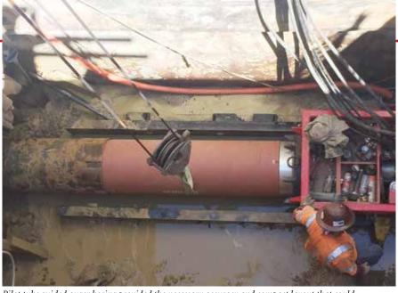
Pilot tube guided auger boring provided the necessary accuracy and compact layout that could accommodate the site constraints
