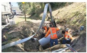
Winding creates a structural liner within the host pipe
