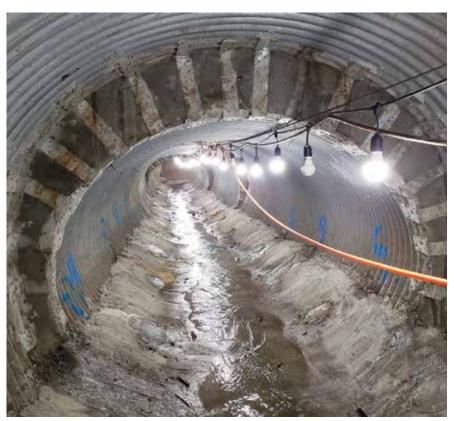
Figure 4. Significant groundwater infiltration
