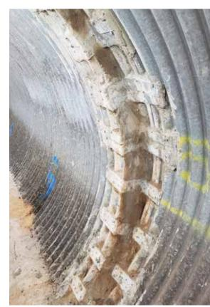
Figure 2. Stabilization of Offset Joints
