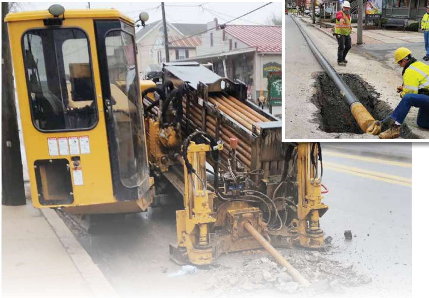
HDD was used to install new potable water pipeline for Intercourse, PA. Nearly 10 miles of HDPE pipe installed
