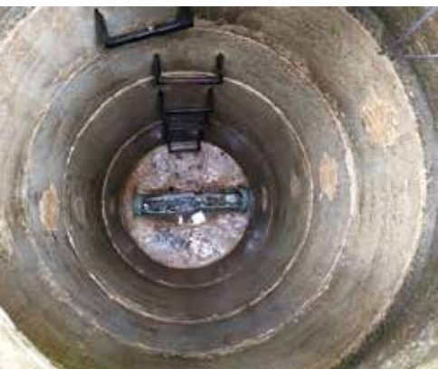
Manholes provide the main human and equipment access to maintain sanitary sewer pipelines
