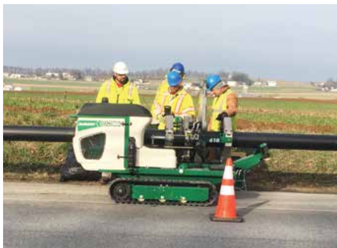
Sections of HDPE pipe were heat fused together to construct a monolithic pipeline nearly 10 miles long. Distributor Core & Main provided a 2-day training session for the crew
