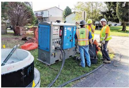
The township found renting the static pipe bursting equipment to be the most fiscally sound for their needs. Here crews connect the hydraulic power unit
