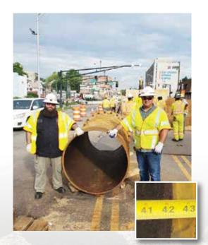
new world record diameter milestone set on July 19, 2019 lining 573 feet of 42-inch high pressure cast iron (CI) gas main crossing under the Garden State Parkway (GSP) at the Central Avenue Bridge in East Orange, New Jersey was due to meticulous planning and lessons learned on previous
