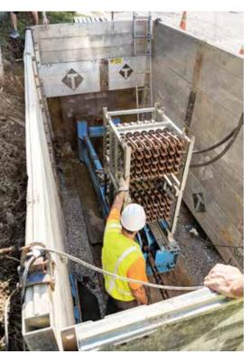
Typical bursting runs range between 270 and 300 feet in length and average 1.5 to 2 hours to complete
