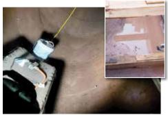
Grout pumped into soil through check valves stopped inflow from heavy rainfall
