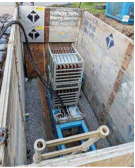
Penn Township has developed a comprehension in-house bursting program. Crews use a Grundoburst 800G static pipe bursting system from trenchless equipment manufacturer TT Technologies, Aurora, IL
