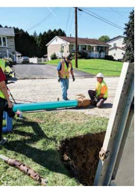
Static pipe burstings allows for the use of a variety of product pipes. Penn Township has been using Certa-Flo® PVC pipe on numerous bursting projects
