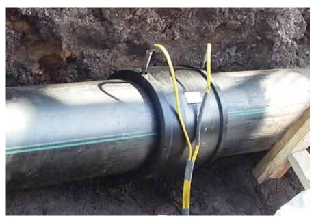
Electrofusion has proven to be an extremely reliable joining system
