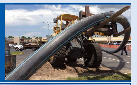
With 100-year design life, zero allowable leakage and the largest internal diameter, HDPE piping is superior for open cut and trenchless installations. It's even recognized by worldwide standards including AWWA C901 and C906, and in the new AWWA M55 Manual.
