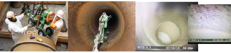
Self-propelled robotic sand blast unit, "The Beast" efficiently cleaned the metal to a NACE-2 finish
