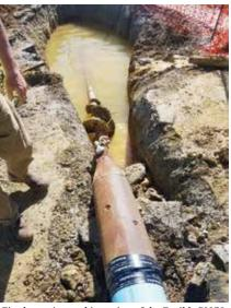
Final reaming and insertion of the Fusible PVC® pipe occurred simultaneously
