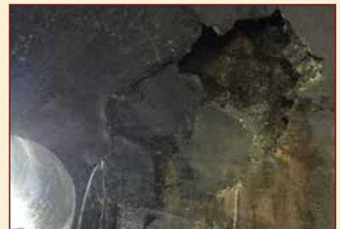
**4.c –Defect after dewatering and minor scaling for safety**
