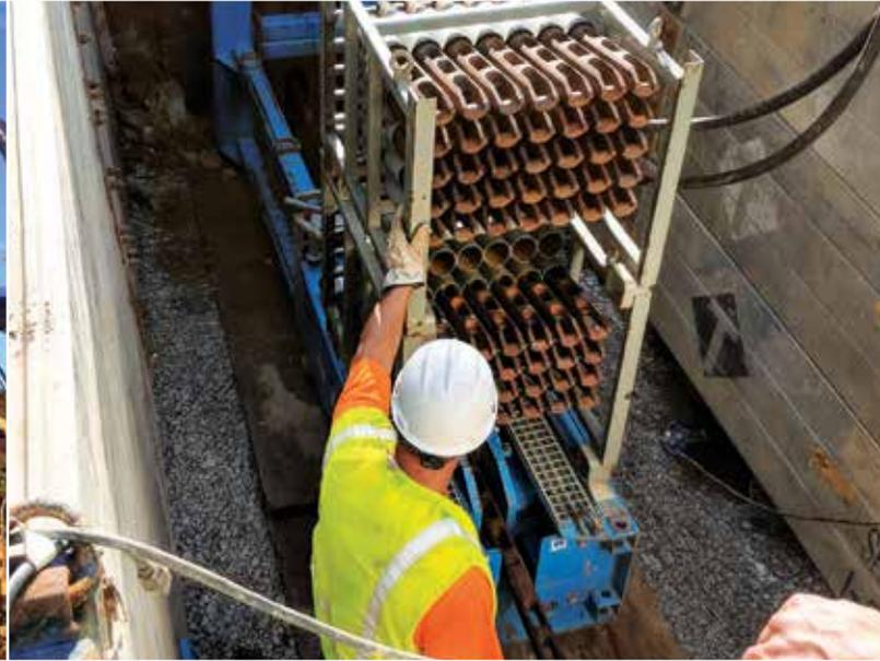
**Static Pipe Bursting: Burst & replace water, sewer and gas pipe with Grundoburst!**
