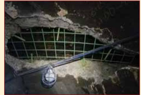
5.c –Welded wire mesh in place for shotcrete repair
