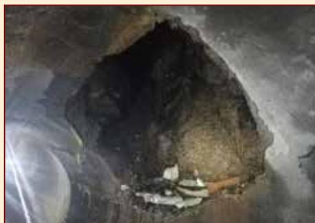
**4.e –Defect after saw-cutting and chipping in preparation for repair**
