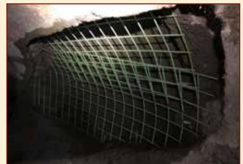
**4.f –Welded wire mesh in place during shotcrete repair**
