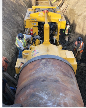
Weld on Reamer stage 4 - 48" to 84"
