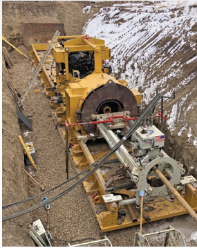
Pilot Bore Akkerman Pilot tube 190'
