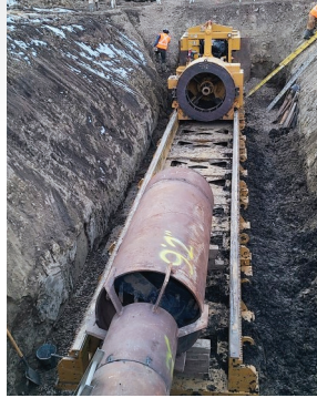
Weld on Reamer stage 2 - 30" to 48"
