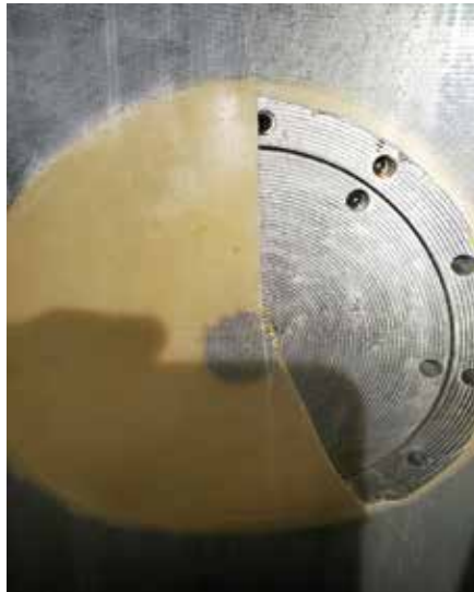
Liner was cut away, plug removed and 20-inch lateral restored after curing
