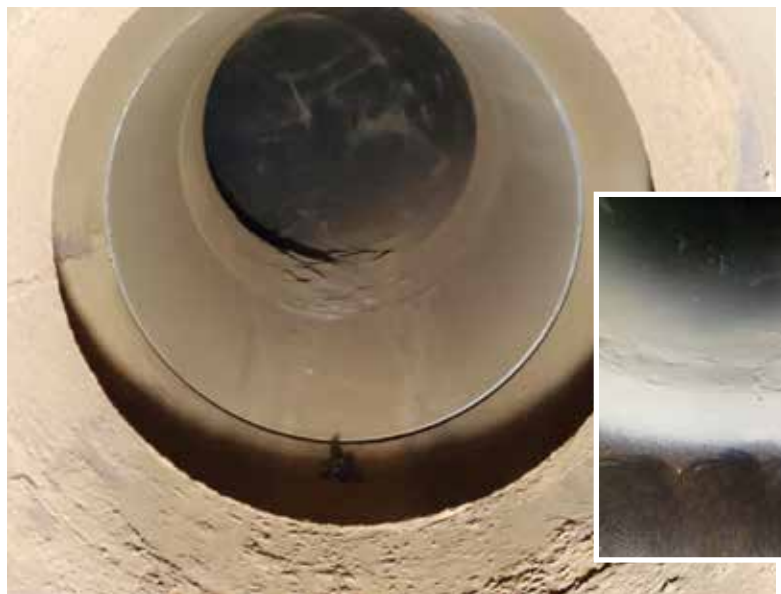
Use of aggregate and mastic epoxy to bridge 30-inch valve gate well was done for the first time ever
