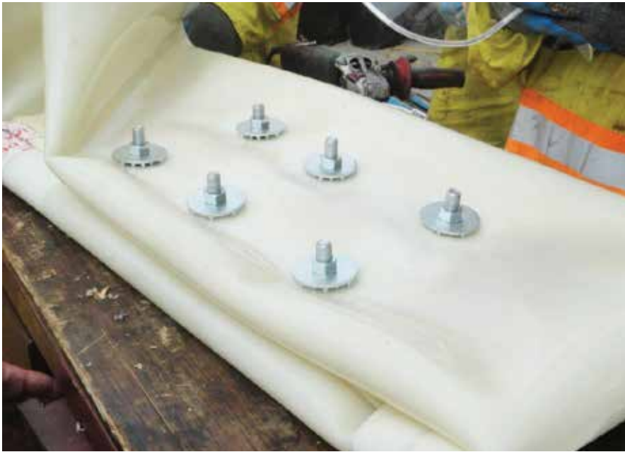
Liner with six tail bolts
