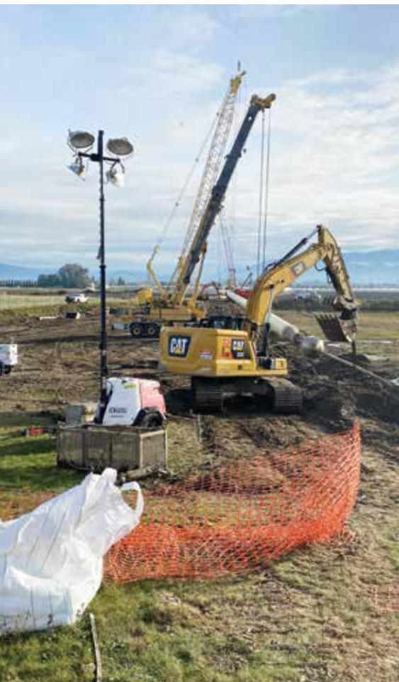
Figure 1. Maxi-Sized HDD Installation
