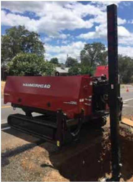
Cable winch being used to slit 4-inch plastic pipe. Pulling force for the operation is kept in-line with the bore axis by means of a self-deploying boom, which needs only a small pit to work from.
