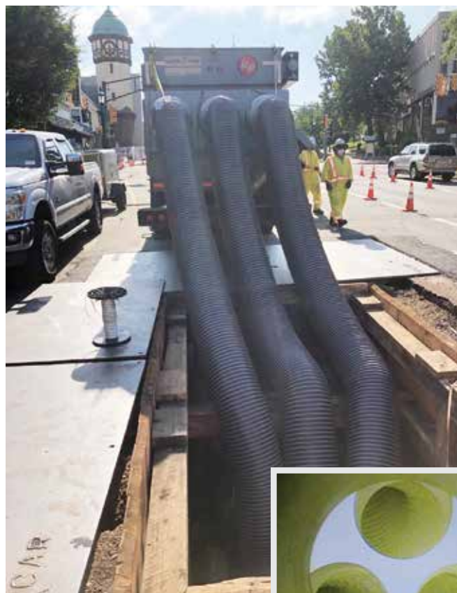
Dust collector with three 16-inch hoses was used to recover leftover cleaning grit
