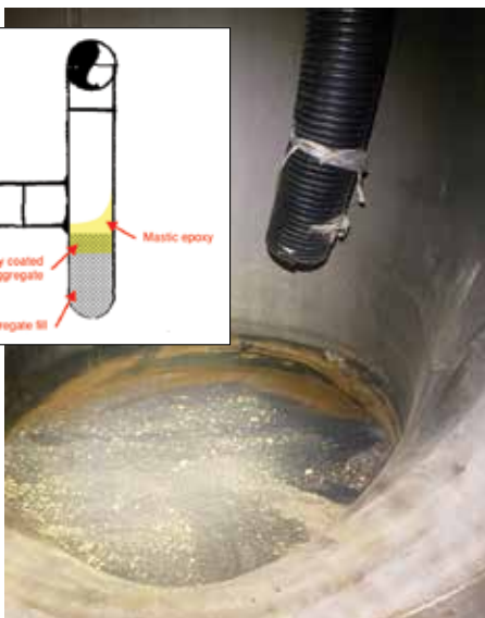
Stack was backfilled, then covered with mastic epoxy to form a 90-degree elbow from the 36x36-inch Tee
