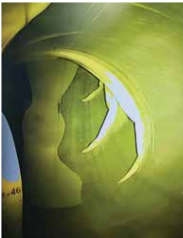
Elbow fabricated from high-strength epoxy was crucial in allowing liner to navigate compound curve with minimal wrinkling
