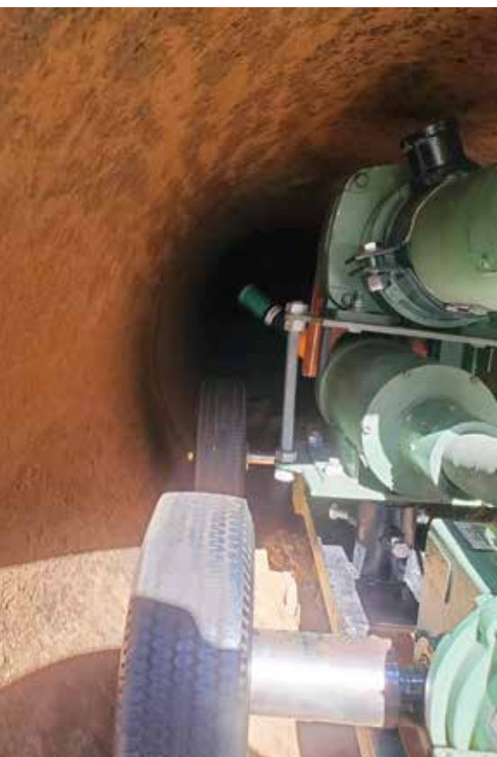
Self-propelled robotic sandblast unit nicknamed "The Beast" was again used to clean the pipe interior before lining
