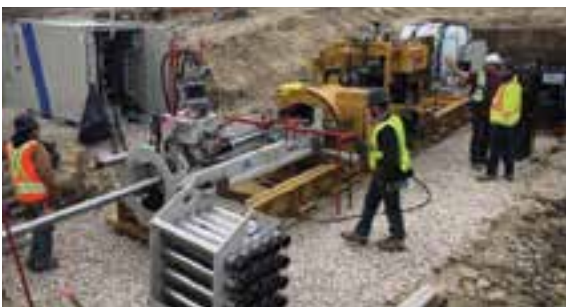
Figure 1: Total Trenchless of Calgary, AB installing pilot tubes for a guided auger boring project.
