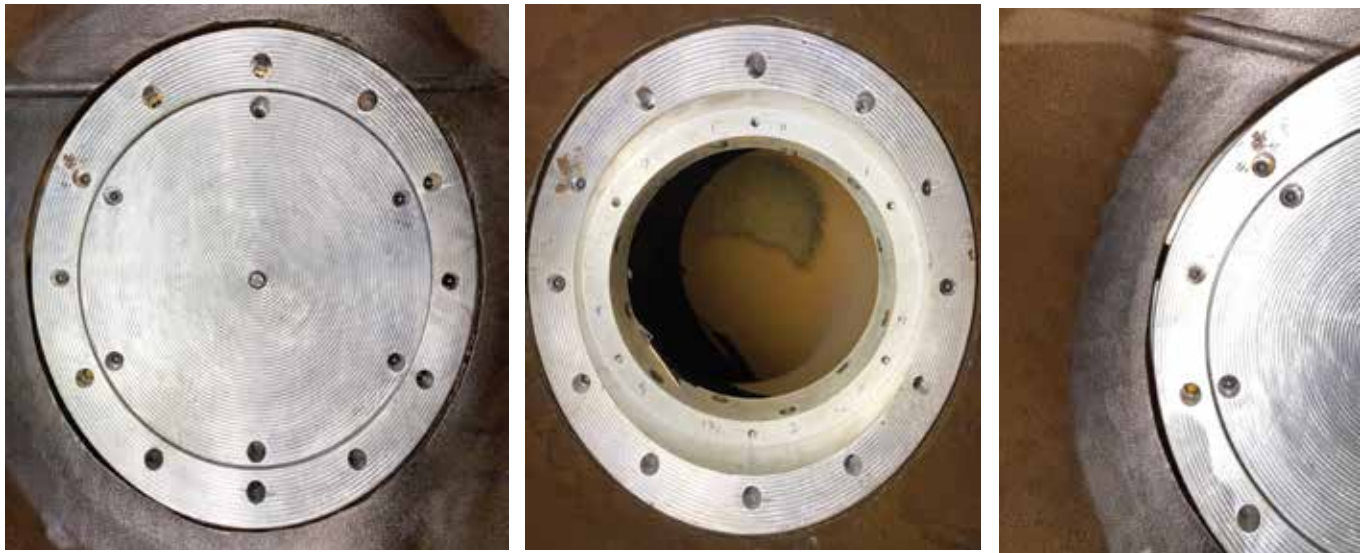
Design engineered prefabricated metal plug installed to cover a 20-inch lateral and provide bearing surface for liner inversion
