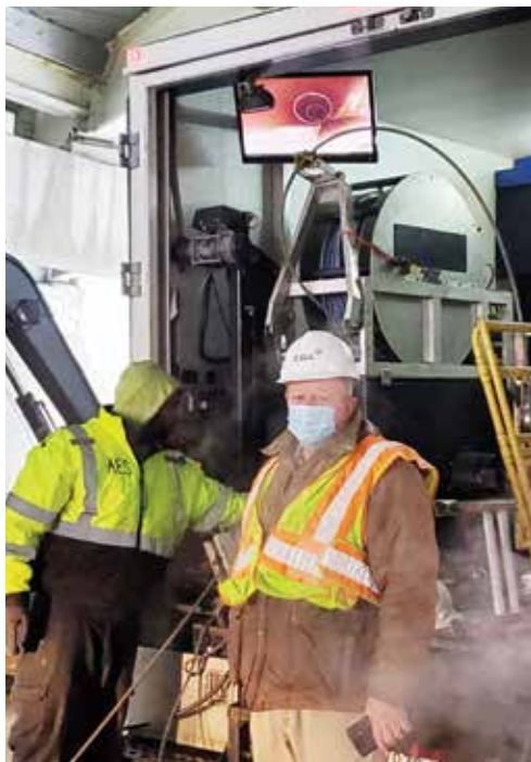
Figure 6. CCTV inspection of pipe in vicinity of the leak required installation of two entry ports
