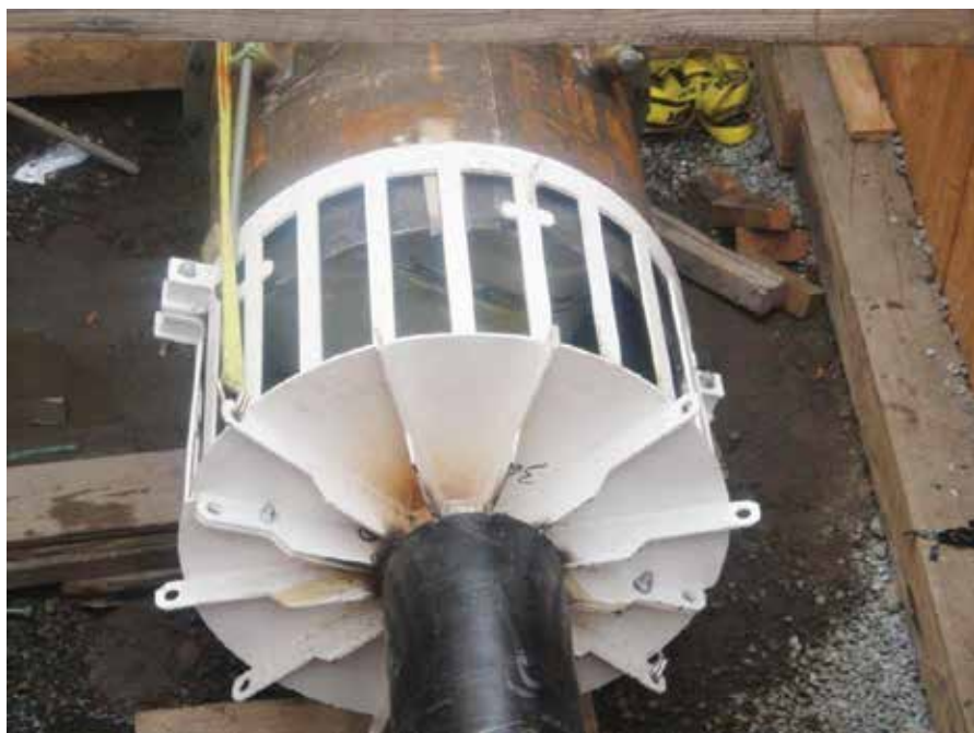
Inversion of the liner through "The Mess" took less than two hours
