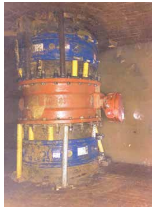
Figure 4. Temporary bracing was used to restrain the new 36-inch butterfly valve while the repair was underway
