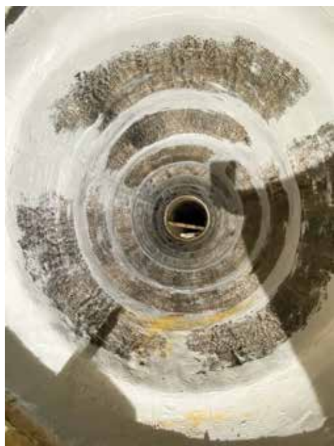
Figure 9. Completed CFR of the 48-inch pipe
