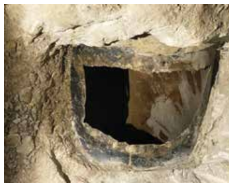
Figure 11. The steel plate was designed to fit the curvature of the pipe to ensure it fit to the cylinder
