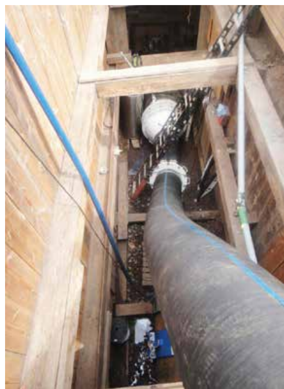
Transport hose used to convey inverting liner down into 10-foot deep pit. This innovation eliminates chafing during liner entry and is referenced as the “US Method”
