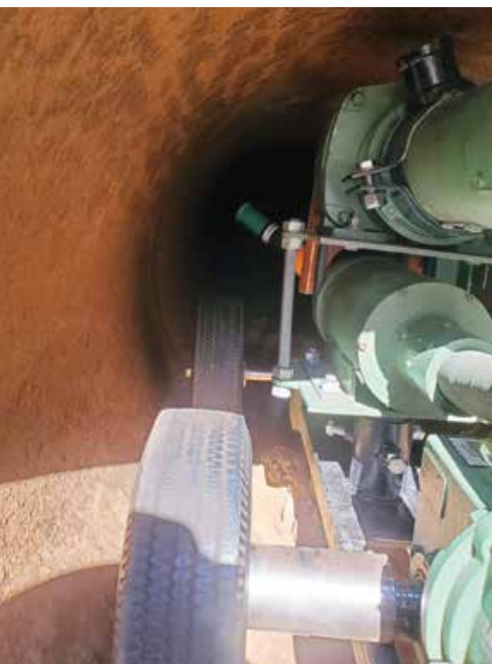
Self-propelled robotic sandblast unit nicknamed "The Beast" was again used to clean the pipe interior before lining
