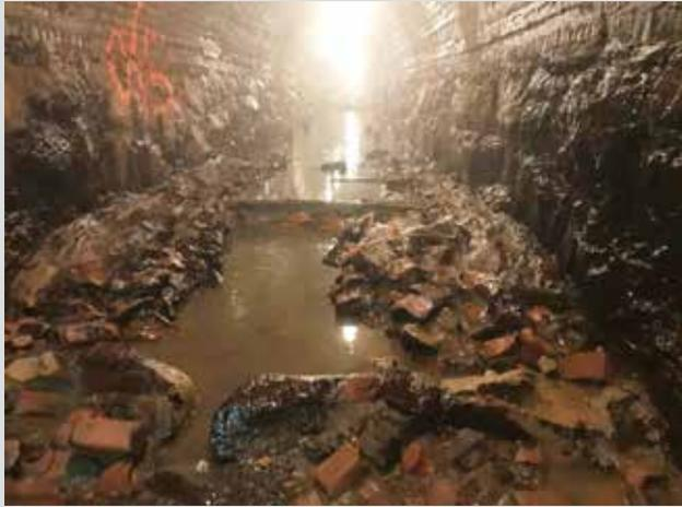
Figure 6. Existing conveyance tunnel invert with significant erosion of brick and granite
