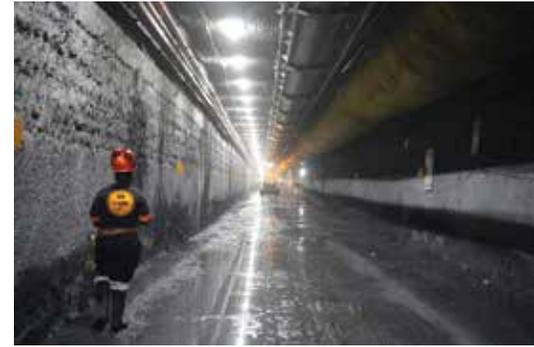
The MDM5000 is particularly useful wherever a rectangular profile is needed, such as train tunnels requiring a flat invert. The rectangular profile requires 30% less rock to be removed as compared with a circular cross section. PHOTO CREDIT: FRESNILLO PLC
