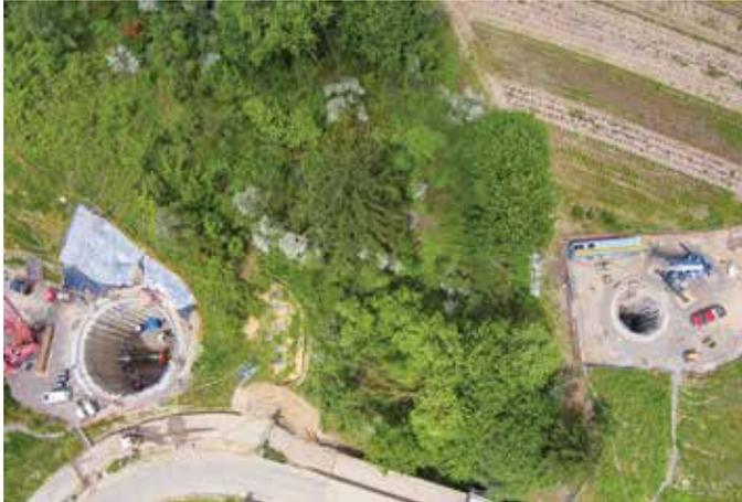
Photo 2 - Watertight secant pile shafts were used for launch and reception of the pipe ram (PHOTO COURTESY OF WILLAMETTE WATER SUPPLY PROGRAM)
