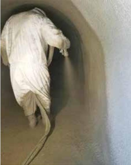
Figure 9. Hand spray application of the geopolymer lining
