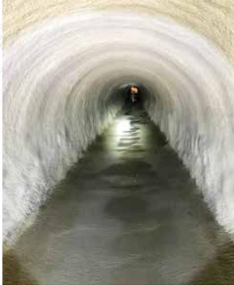
Figure 10. Completed lining of the original 96 x 96-inch brick/granite arch tunnel
