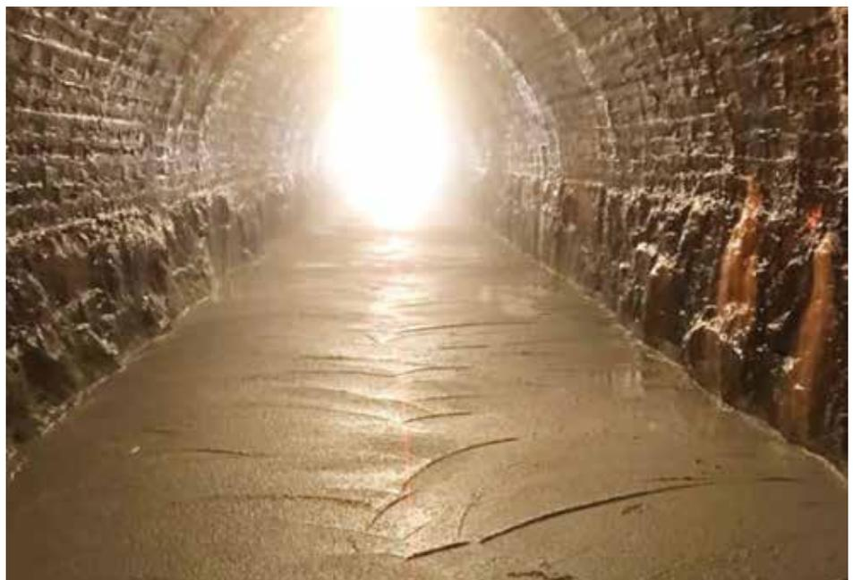
Figure 8. Completed 24-inch thick poured concrete floor to stabilize the flow and smooth the floor
