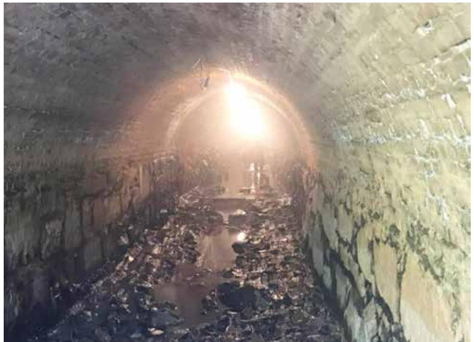
Figure 1. Internal view of the existing granite and brick tunnel prior to rehabilitation
