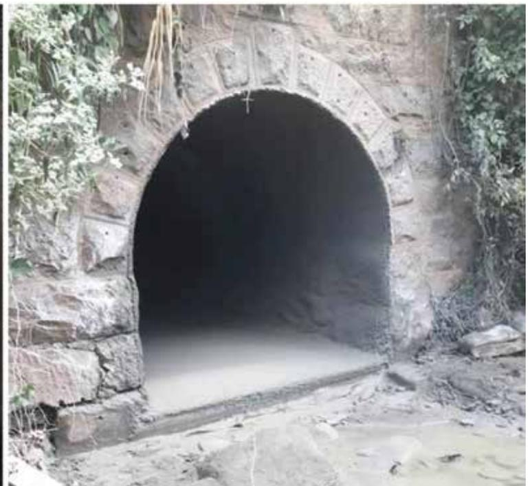
Figure 11. View of the completed lining at the outlet of the tunnel at the Broad River
