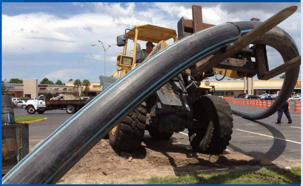
With 100-year design life, zero allowable leakage and the largest internal diameter, HDPE piping is superior for open cut and trenchless installations. It's even recognized by worldwide standards including AWWA C901 and C906, and in the new AWWA M55 Manual.
