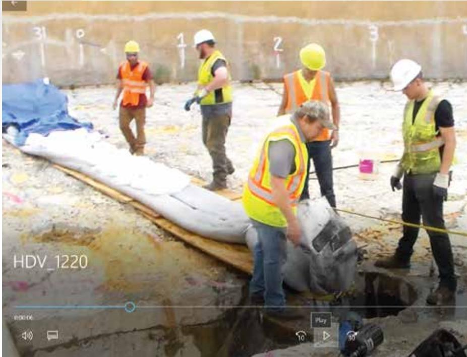
Figure 5. Preparing to load liner into tunnel in PST #1
