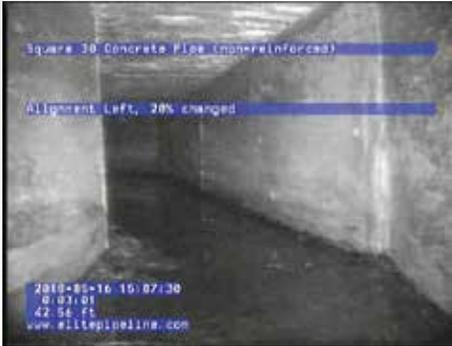
Figure 3. Example of bends in the tunnels and existing conditions after cleaning
