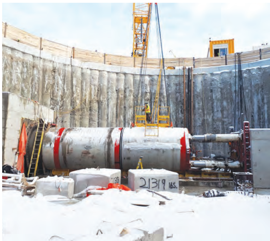
Figure 10. Microtunnel Setup for the HLI Extension in the Screen Building Shaft.
