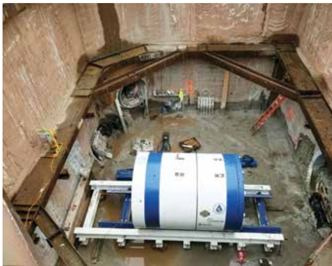
Figure 6 – 96-inch MTBM awaiting the start of tunneling
