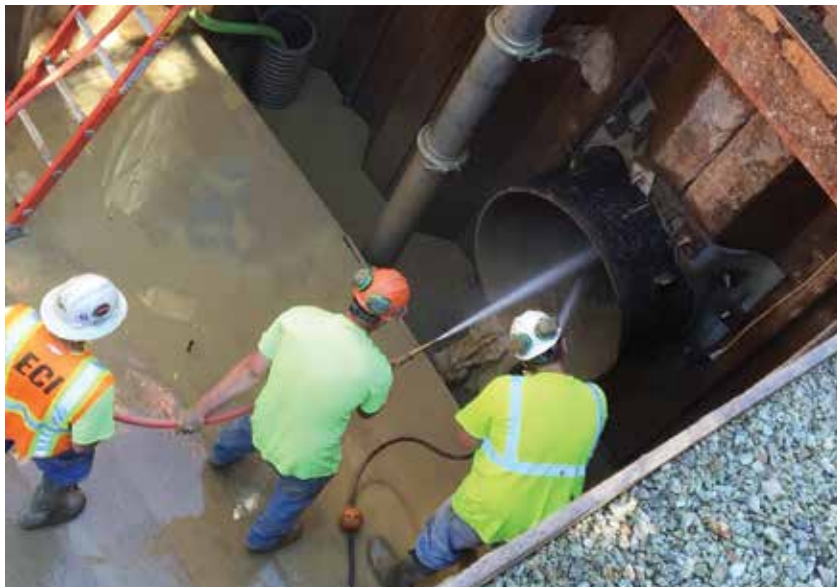
Cleaning the 42-inch casing
