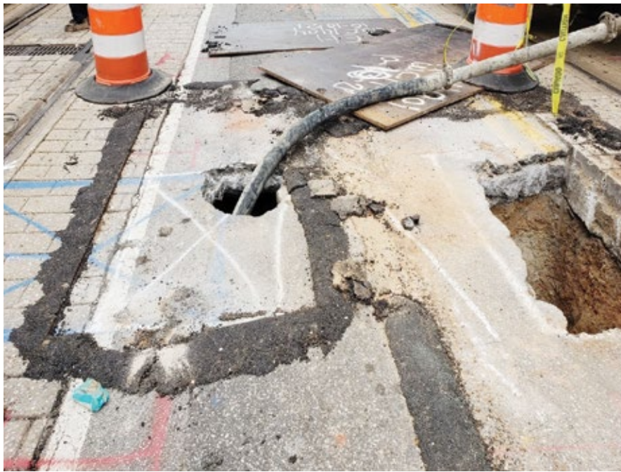
Figure 8: Grouting of major void with flowable fill, with access just outside of light rail slab
