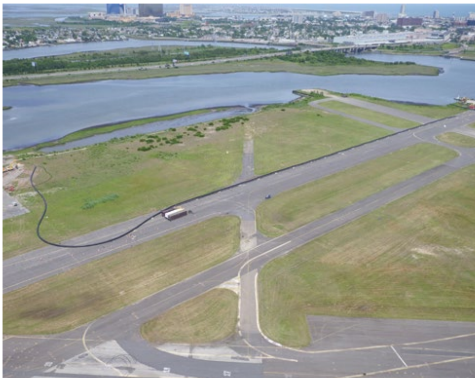
Heat fusing the sections of HDPE pipe was done and the resulting monolithic pipeline was staged along a runway at the former Bader airfield, ready for the 1,500-foot HDD pull 80 feet under the Beach Thorofare waterway. (PHOTO COURTESY OF ACUA)
