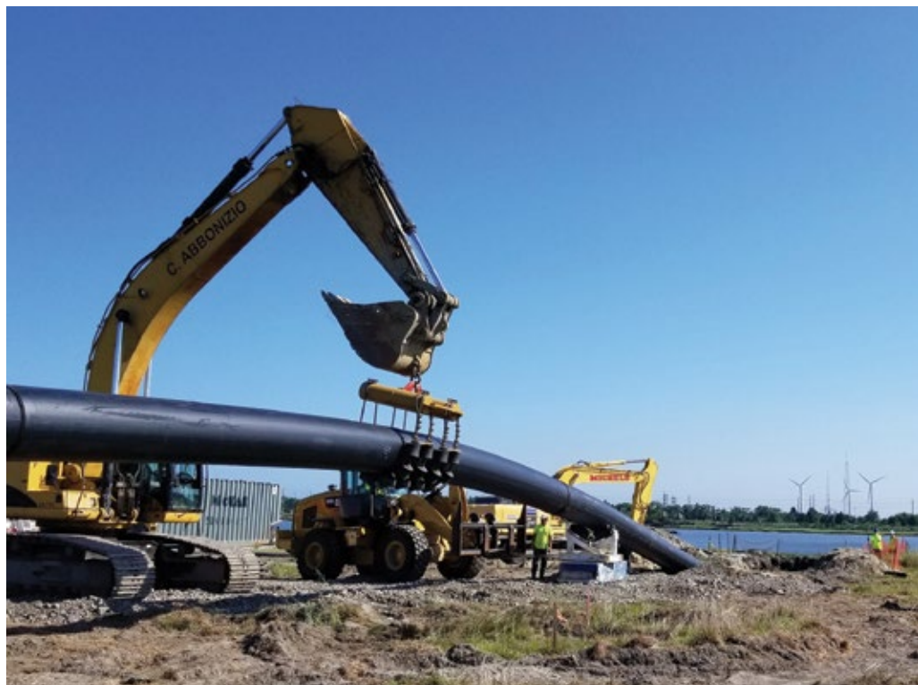
The 30-inch diameter HDPE PE 4710 pipe being pulled backward in the HDD process. (PHOTO COURTESY OF ACUA)
