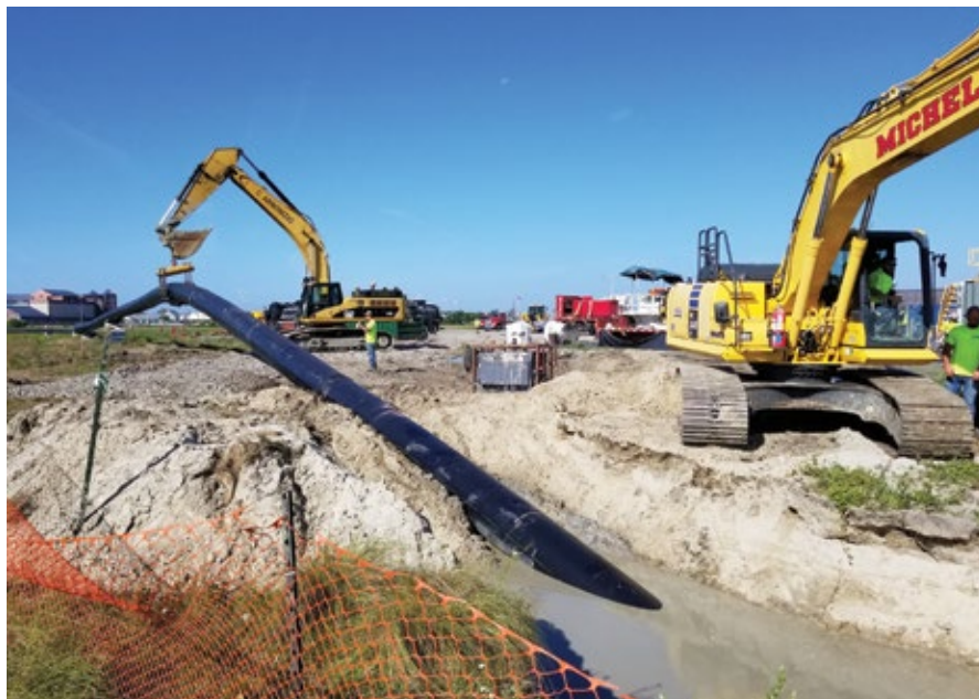
The 30-inch diameter HDPE PE 4710 pipe enters the HDD path to go under the Beach Thorofare waterway. (PHOTO COURTESY OF ACUA)
