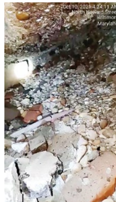
Figure 7: One of the largest voids discovered under the light rail slab
