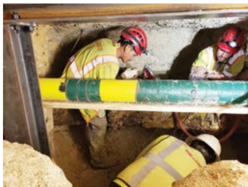
Figure 12: When tunneling towards the valve, a large gas line was encountered
