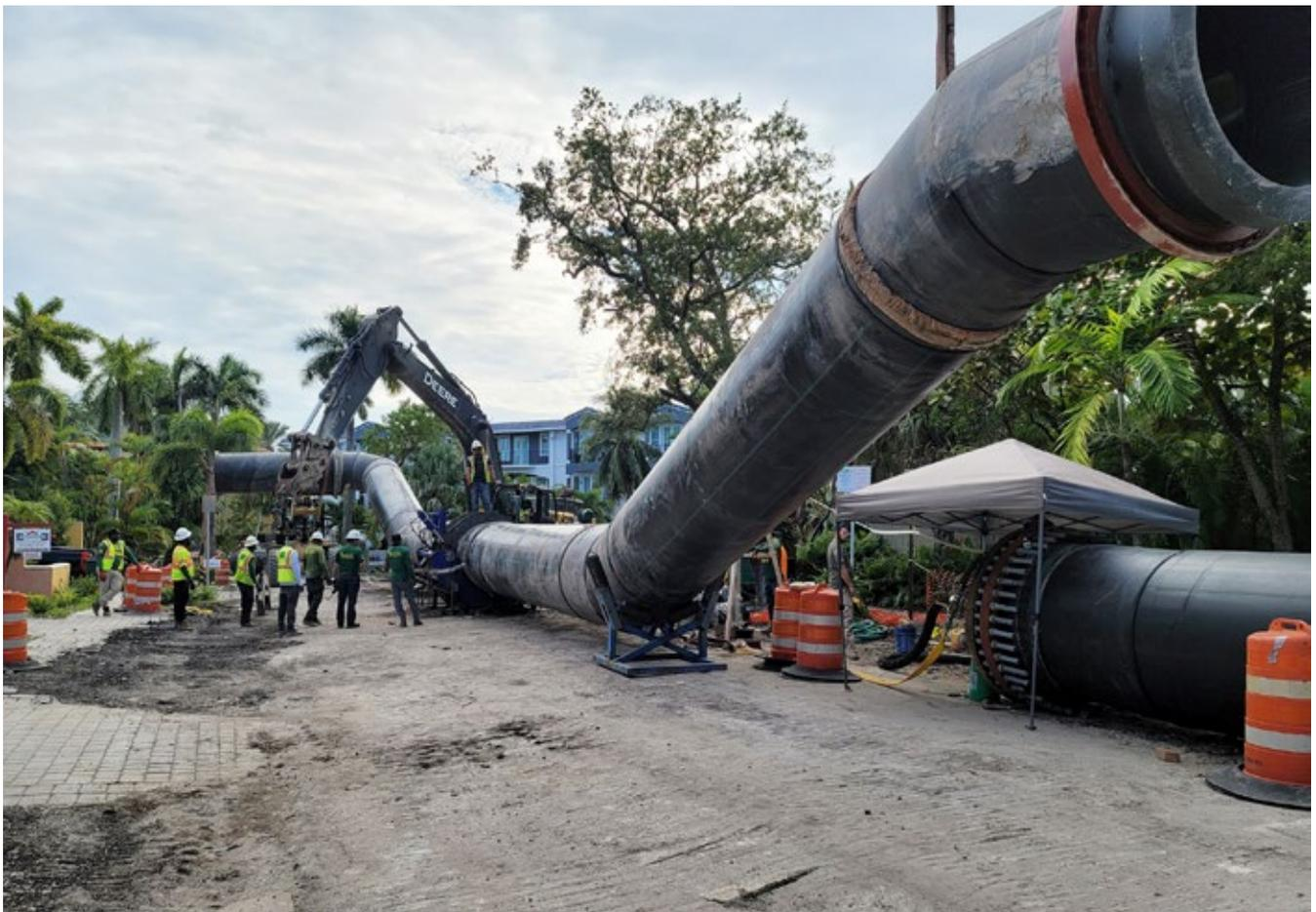
*Four of the HDD segments required unique compound curves due to roadway geometry and field conditions*
