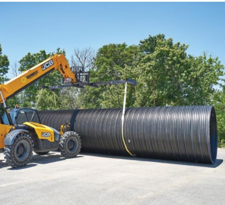
Liner pipe was shipped directly to the site in 41-foot and 45-foot sections
