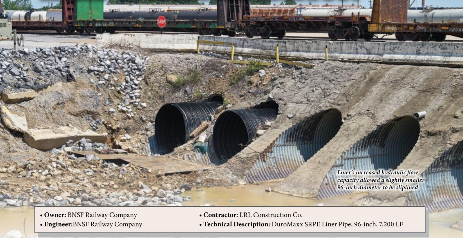
*Liner's increased hydraulic flow capacity allowed a slightly smaller 96-inch diameter to be sliplined*
