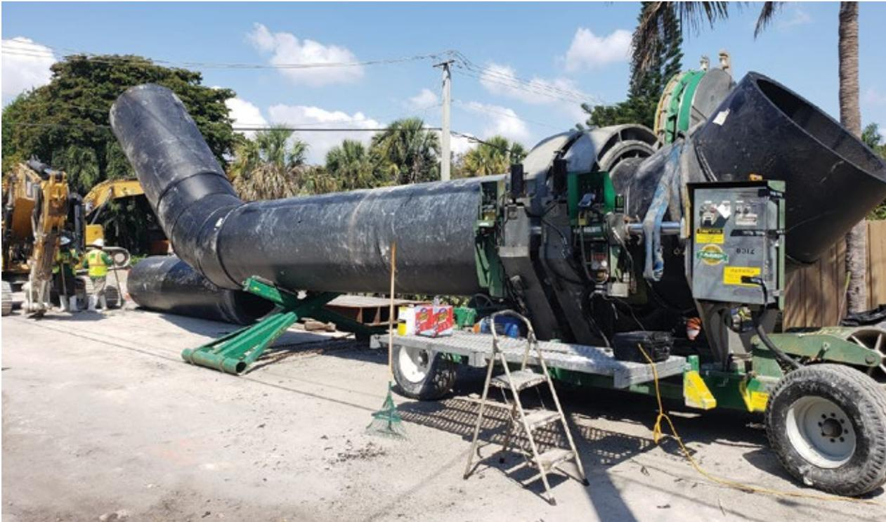
Fused joints eliminate infiltration and exfiltration
