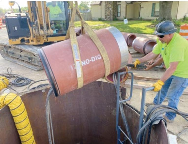
Short (1-meter) VCP-J pipe lengths make the 8-foot shafts functional
