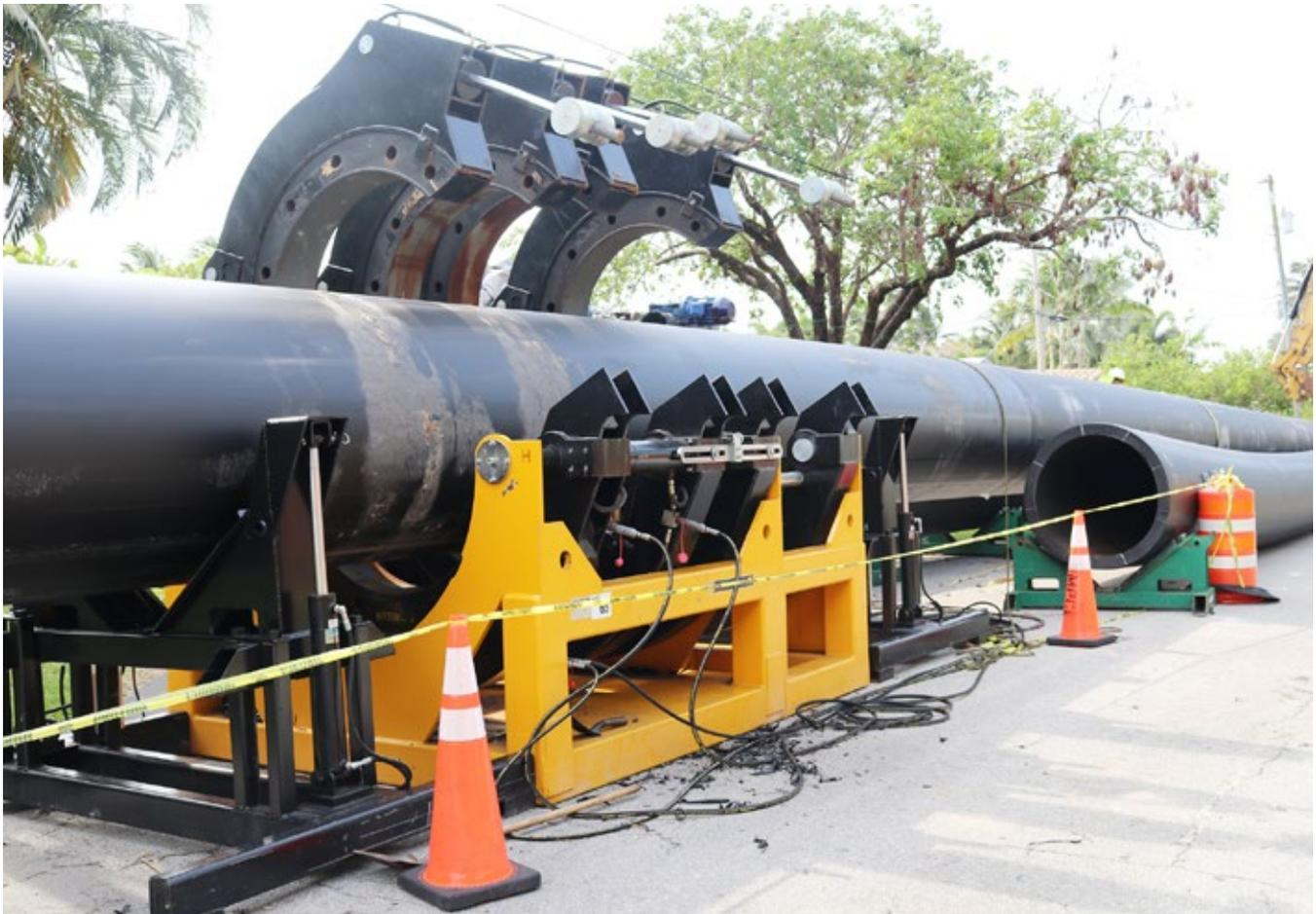
*HDPE's heat-fused joints create a leak free, self-restraint, monolithic piping system*
