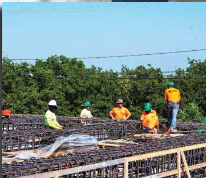
Left: Crew members lay rebar for the FKA's new generator building. Each piling is more than 3 feet in diameter to anchor the foundation in place if a catastrophic hurricane hits.
