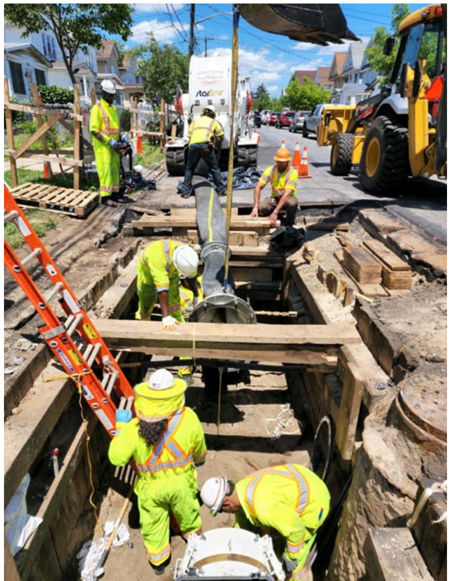
PPM crew prepare the transfer hose for lining the 24" cast iron natural gas pipeline on 134th Street
