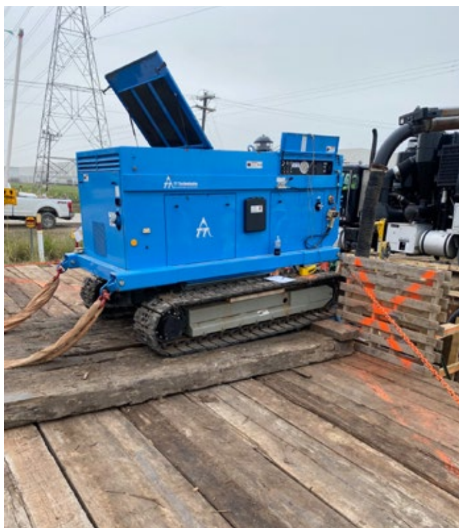
MAXX HDD used a 20-ton Grundowinch from TT Technologies to pullback a carrier pipe in a tight location where a traditional directional drilling pullback wasn't feasible
