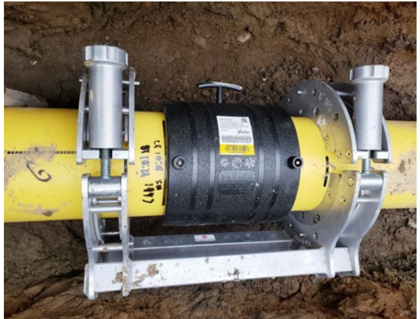
A properly prepared EF Coupling with Clamp
