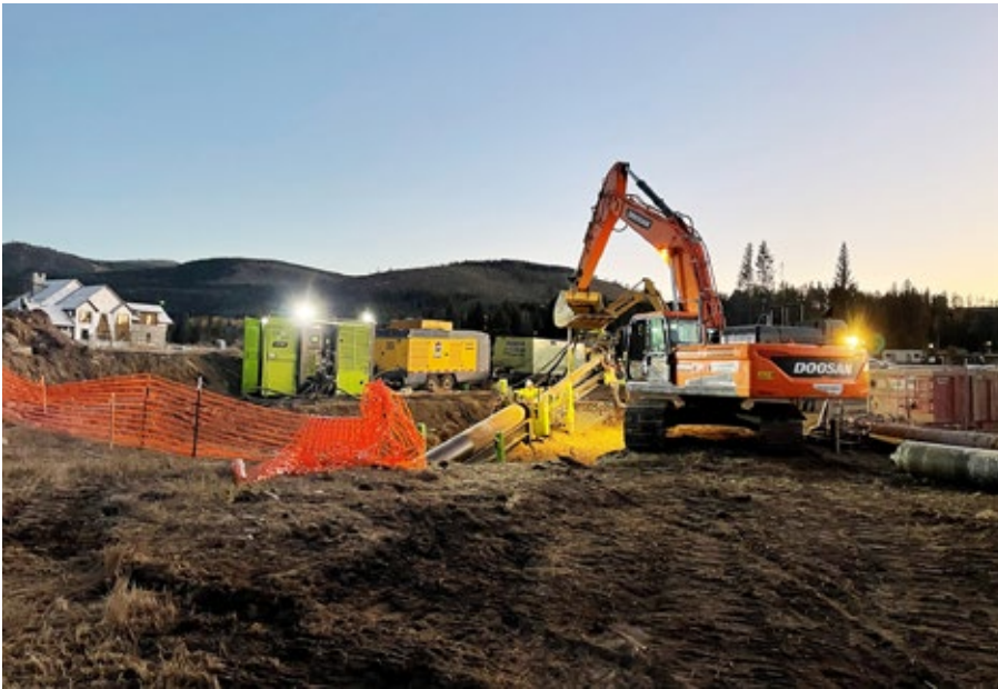
System does not require the use of drilling fluids
