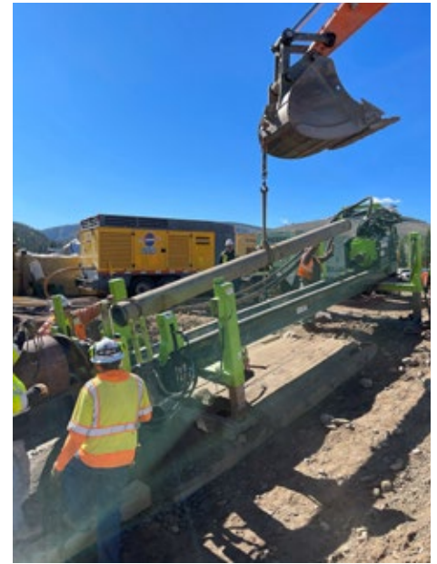
Desired 12 degree entry angle was met by adjusting independent hydraulic legs
