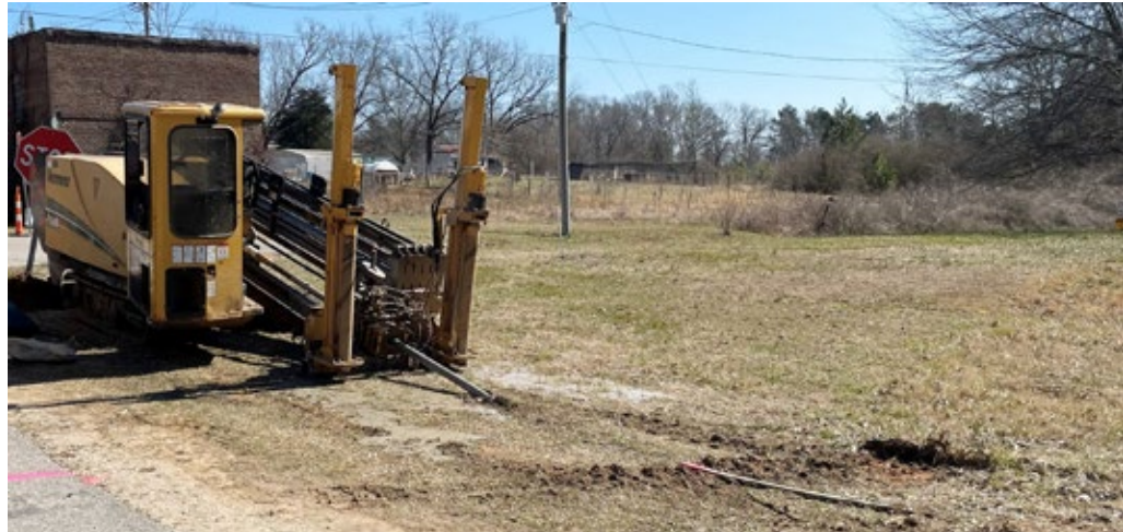
HDD Machine starting bore hole
