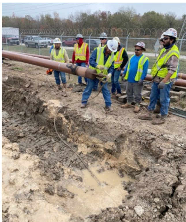
The 450 feet of 8-inch diameter steel carrier pipe was installed as part of storage facility development
