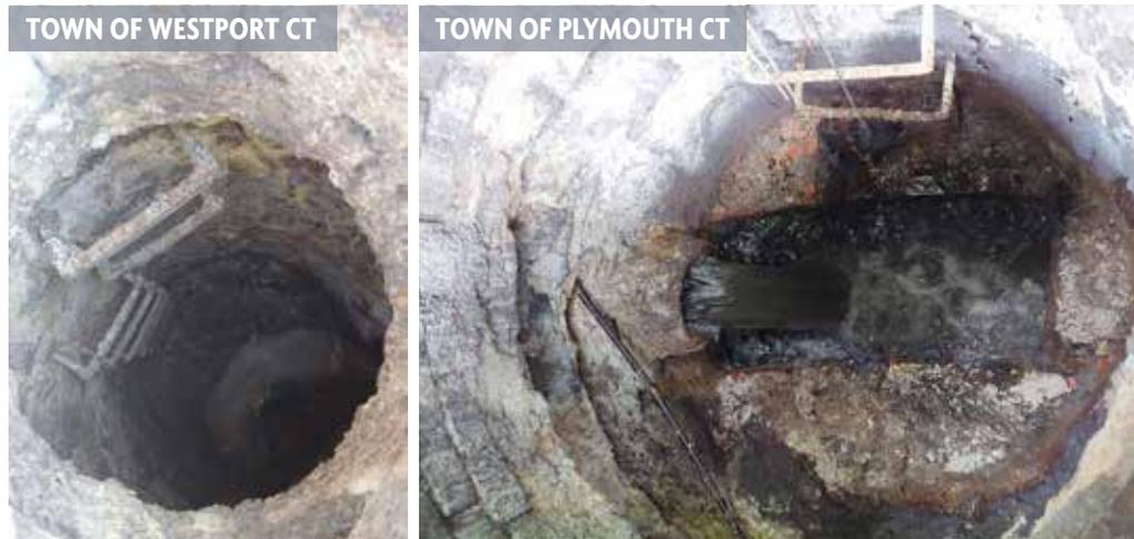
Figure 1. Over time corrosion in a manhole can be significant, creating unsafe conditions
