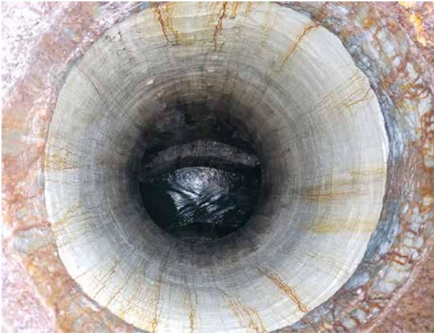
Figure 4: Rehabilitation on this manhole was done 14 years ago using the same composite system
