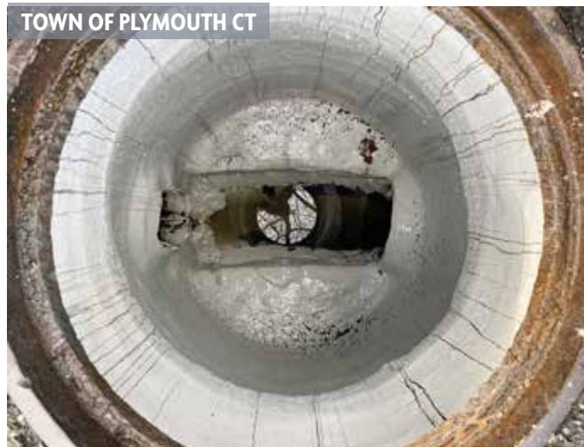
Figure 3. Completed rehabilitated manholes
