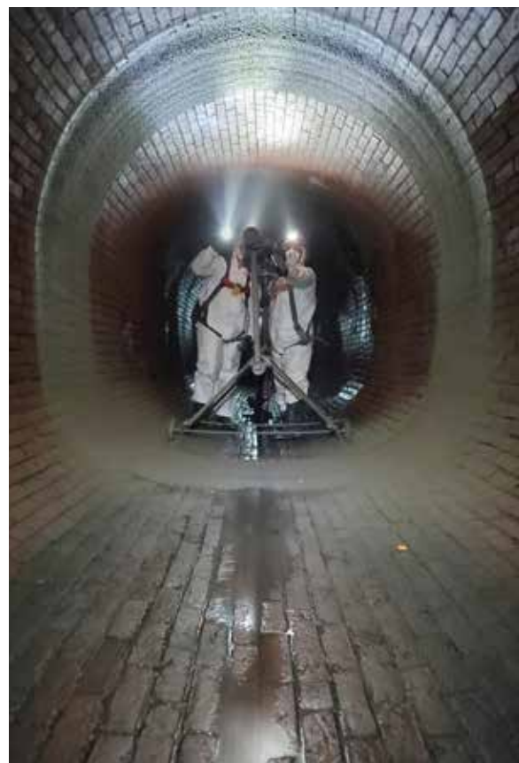
Spraying the first 0.5-inch layer of liner in the interceptor
