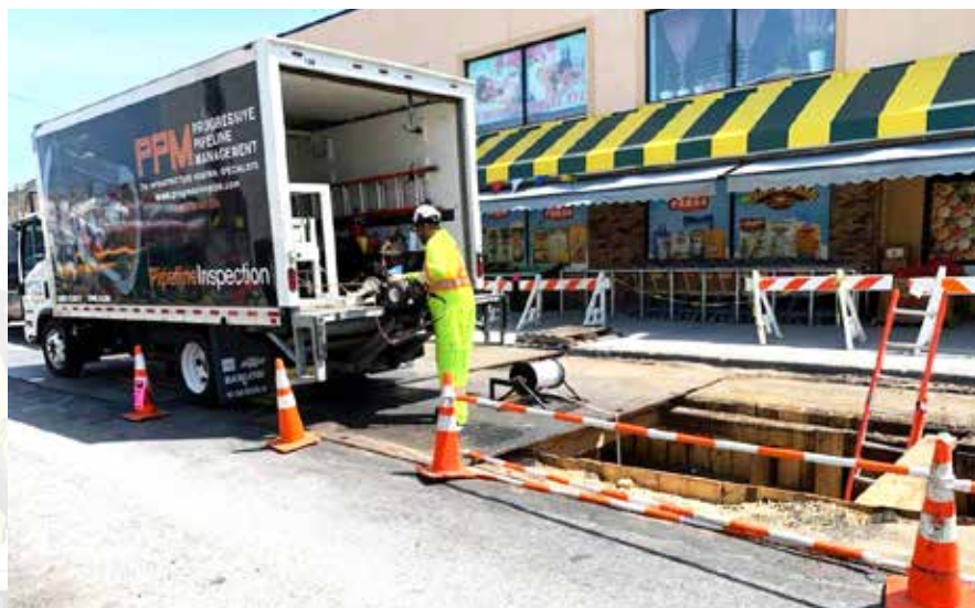
PPM crew with ARIES LETS CCTV camera used to inspect the pipeline prior to lining
