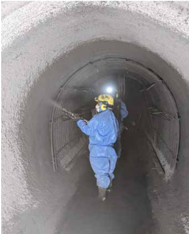
Spraying liner over basalt reinforcing bar (left) and completed manhole rehabilitation (right)
