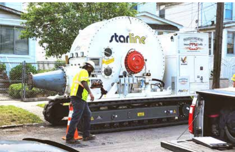
The Starline® Cured-in-Place-Lining Inversion Drum on 134th Street
