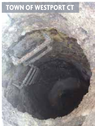
Figure 1. Over time corrosion in a manhole can be significant, creating unsafe conditions
