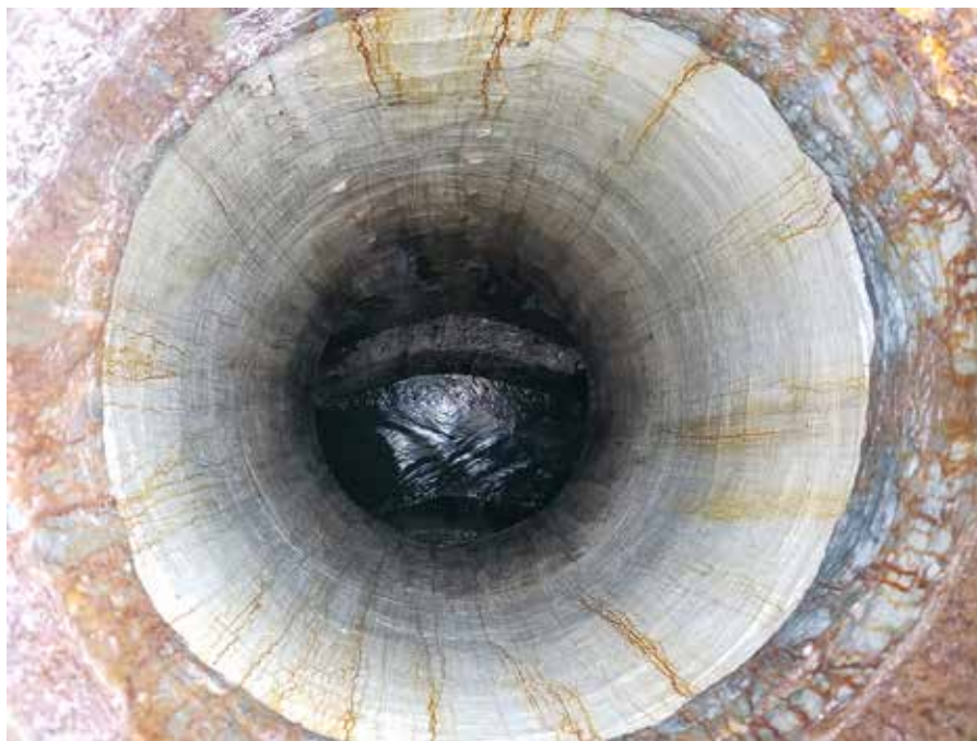
Figure 4: Rehabilitation on this manhole was done 14 years ago using the same composite system
