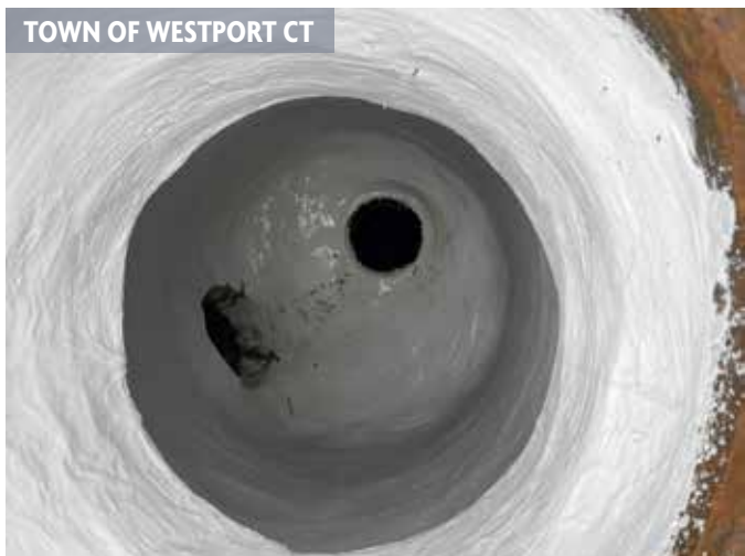
Figure 3. Completed rehabilitated manholes
