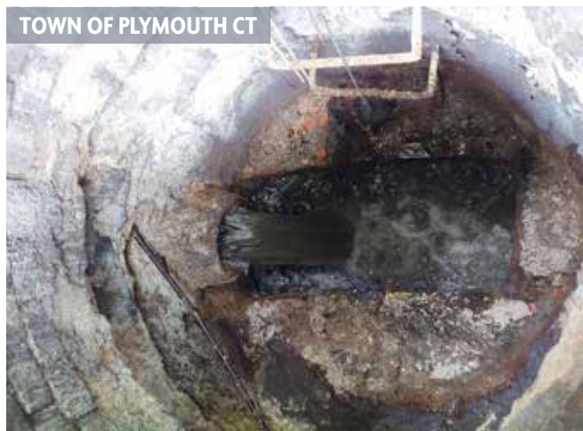
Figure 1. Over time corrosion in a manhole can be significant, creating unsafe conditions
