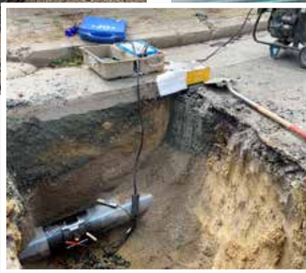
Electrofusion in Pit
