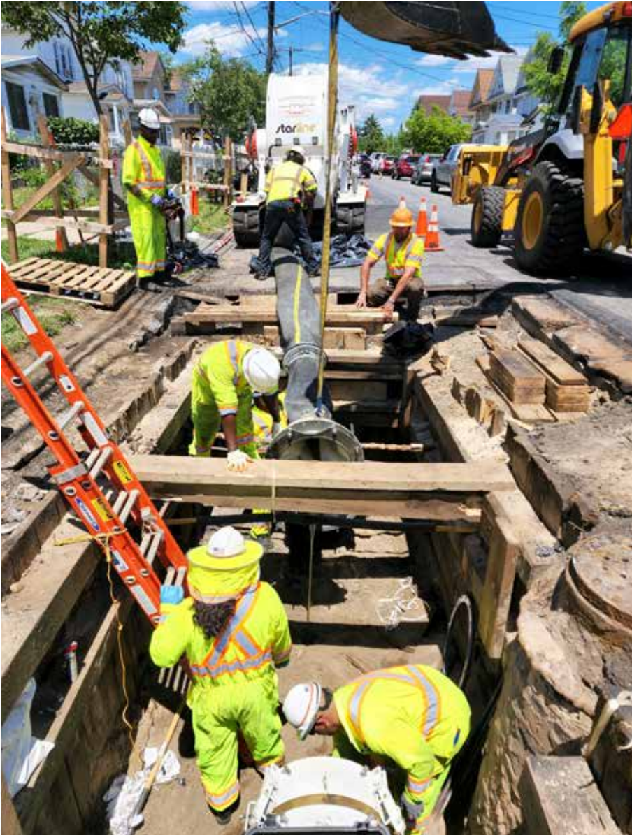
PPM crew prepare the transfer hose for lining the 24" cast iron natural gas pipeline on 134th Street
