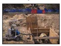
A pipeline construction project replacing a deteriorating 42-in. pipeline more than 20 ft below the surface of a small river met with trouble as unstable shores prevented directional drilling. Rain also brought constantly changing river levels,
