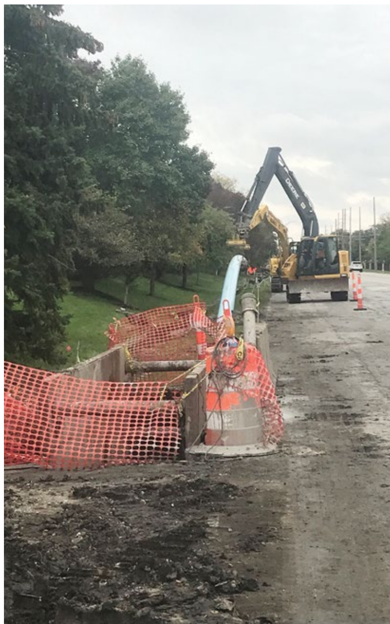
New main followed the same path as the existing main. Over 11,000 LF of Fusible PVC Pipe® was installed
