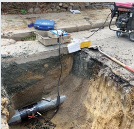
Electrofusion in Pit
