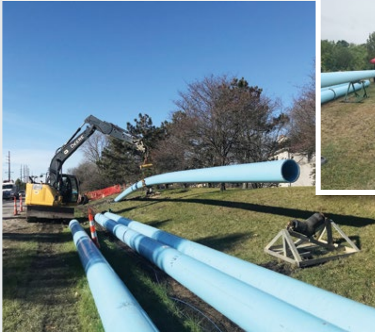
"The Fusion operation required additional forethought for layout but once installed the pressure test held like a drum" - AUSTIN RIDGE, ENGINEER, NIES ENGINEERING
