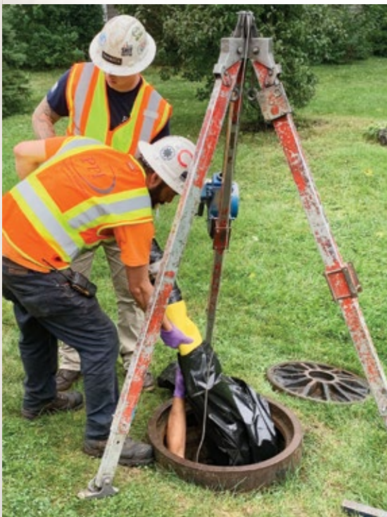
Figure 7. T-liner, wrapped in a UV proof bag
