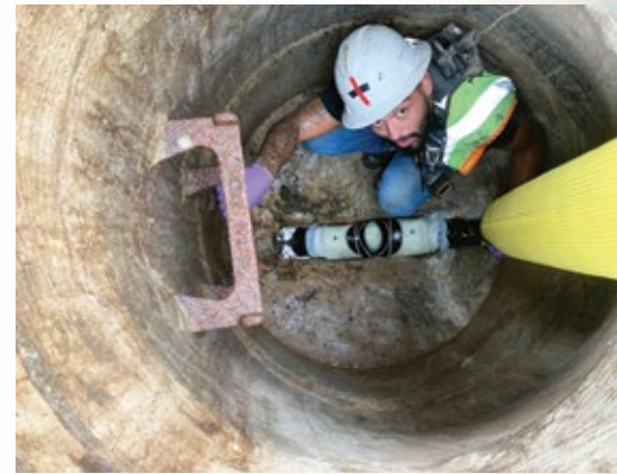
Figure 8. Sending the T-Liner in (from the manhole)
