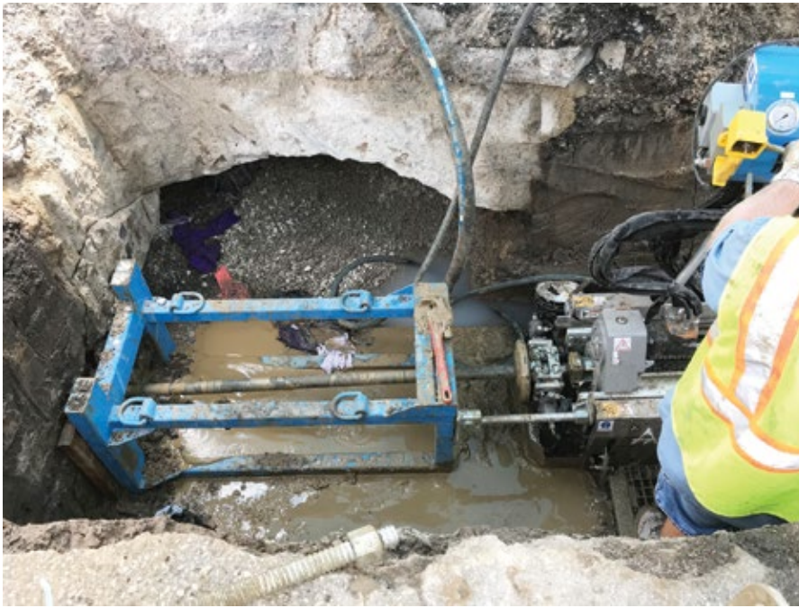
The Grundopit pit launch directional drill from trenchless equipment manufacturer TT Technologies is just 54 inches long, 43 inches wide and 57 inches tall, making it ideal for the difficult St. Paul neighborhoods
