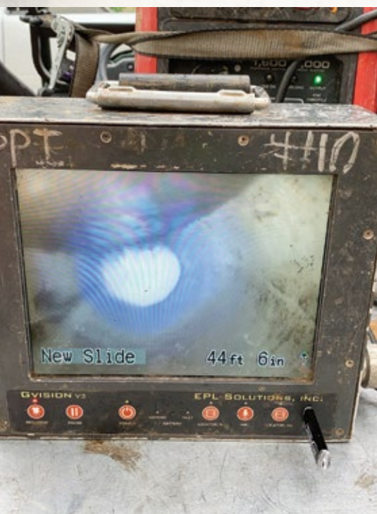
Figure 9. UV curing process (View from the cleanout)
