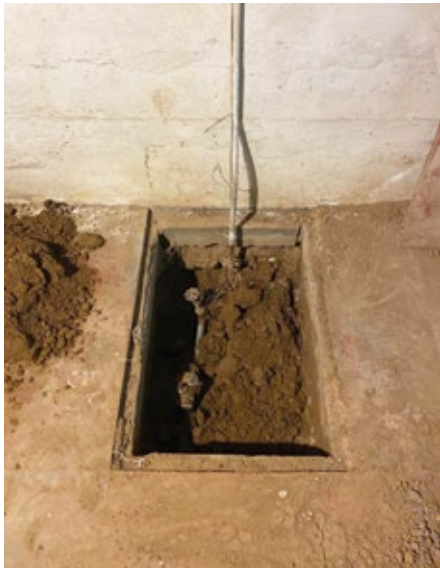
Triple E crews are boring into customers basements and pulling back new copper services
