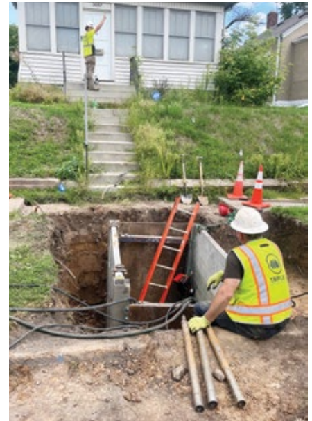
Triple E Water and Sewer is utilizing pit launched HDD technology to replace lead water service lines in St. Paul, MN
