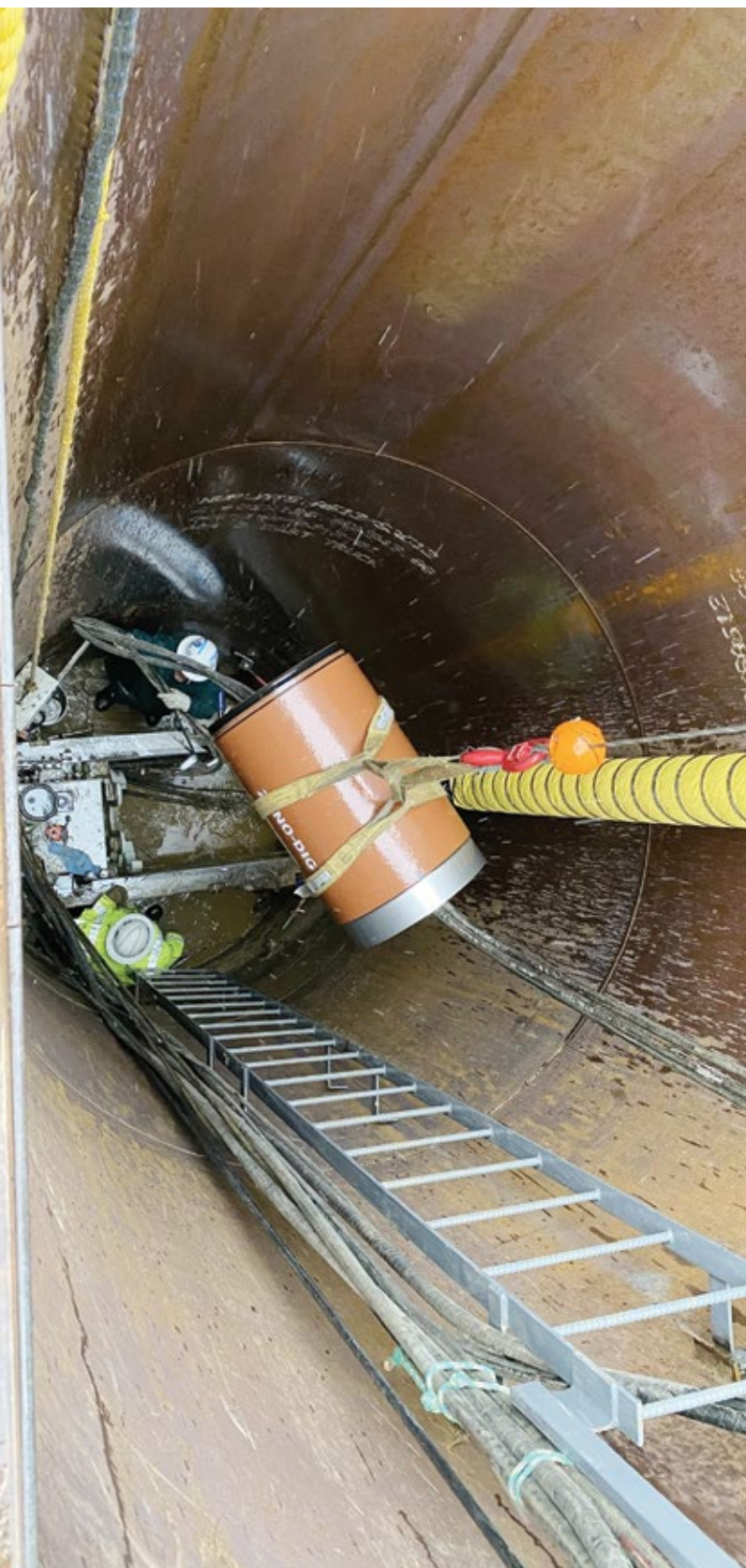
The depth needed to tie in to the existing sewer was one of the challenges that made the Pilot Tube Method of guided boring the right choice for this project
