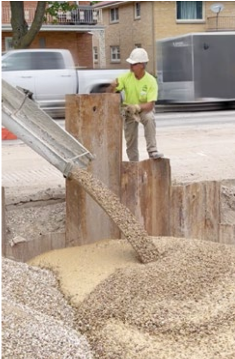
Given the high-traffic surroundings and the need for quick restoration, the backfill method of choice for the shafts consisted of a sand/gravel slurry mix
