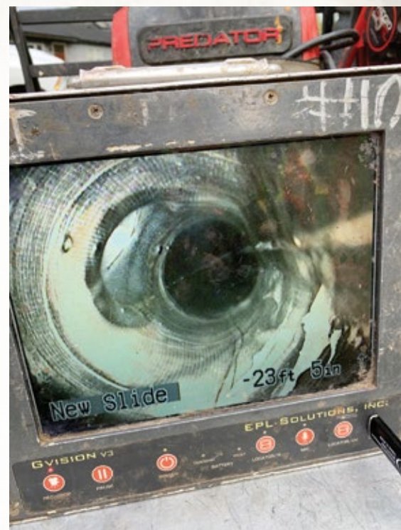
Figure 10. UV cured T-Liner (Installed)
