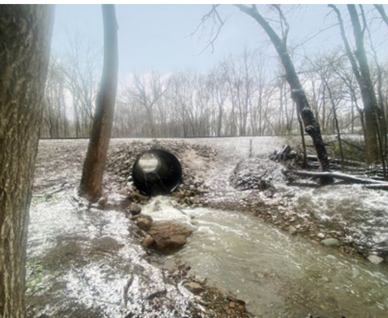
Converting the original trestle to a buried DuroMaxx® SRPE culvert brought even greater efficiencies to the railway including minimal maintenance
