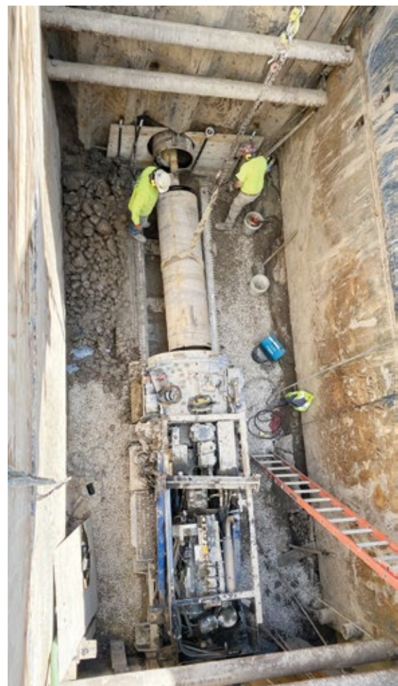
The American Augers 36-600 auger boring rig installing the 25-inch diameter by 10ft length temporary steel casings in the second step
