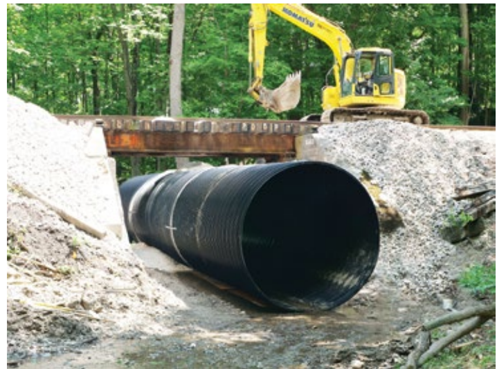
Three 20 LF segments of 120-inch DuroMaxx were needed to reline the existing train trestle
