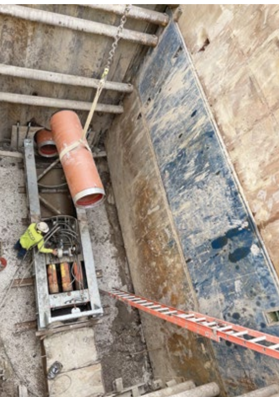
An installation depth of 25 feet was another reason that PTM was the best option for this job
