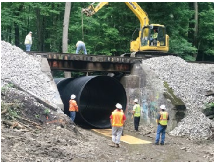
Each segment was properly aligned and honed for a tight fit prior to backfilling
