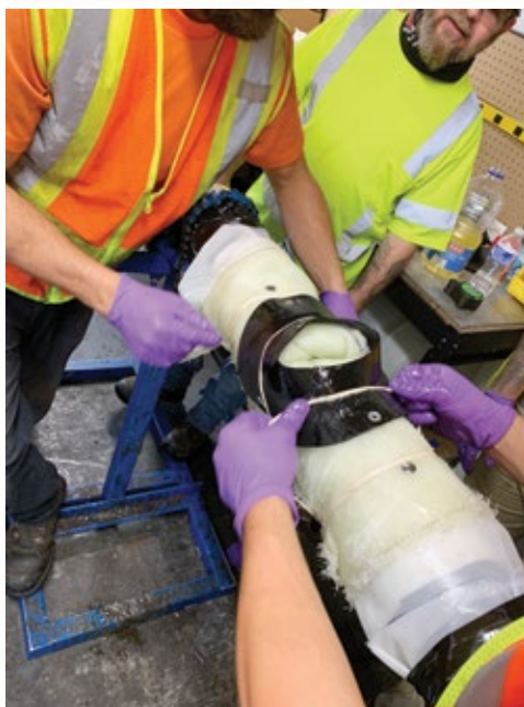
Figure 4. UV T-Liner & hydro-hat being setup
