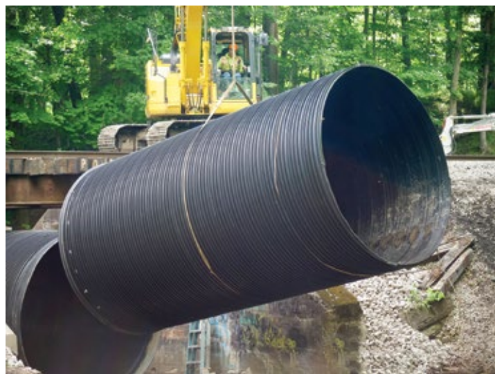
The DuroMaxx® SRPE Liner Pipe is set in place beneath the existing train trestle
