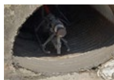
Cement Pipe Rehab
