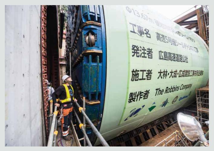
The 13.7 m (44.87 ft) diameter Robbins Slurry machine launched on September 18, 2018 in Hiroshima, Japan.
