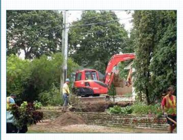
Figure 6 – Excavation in Wauwatosa after the Sept. 15, 2012 pipe break. The pipe runs parallel to, and behind, the retaining wall. Note the limited access along this pipe easement and the presence of overhead private utilities.
