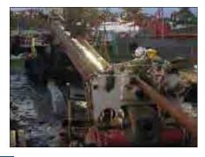
Staheli Trenchless Consultants was part of the design team for the South Magnolia CSO project for King County, Wash. The project included construction of an on-grade 3,074-ft pipeline beneath Magnolia Hill to convey excess flows to a 1.5 million gallon storage tank near Smith Cove Park in Seattle. The intersect method of horizontal directional drilling was used to install the 32-in. fusible PVC pipe at a slope of 1.8 percent beneath the hill, with a maximum depth of cover of over 150 ft.
