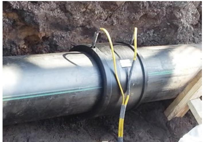
*Information about electrofusing polyethylene pipe procedures can be found in the updated MAB Generic Electrofusion Procedure for Field Joining of 12 Inch and Smaller Polyethylene (PE) Pipe (MAB-01-2022), one of two electrofusion documents available for free on the PPI MAB website: [www.plasticpipe.org/municipaladvisoryboard](http://www.plasticpipe.org/municipaladvisoryboard).*
