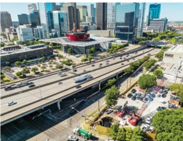
*The view of the breakthrough shaft from overhead: The Mill Creek tunnel is a designated critical infrastructure project for the City of Dallas, providing 100-year flood protection for areas of East Dallas that have experienced severe flooding in the past*
