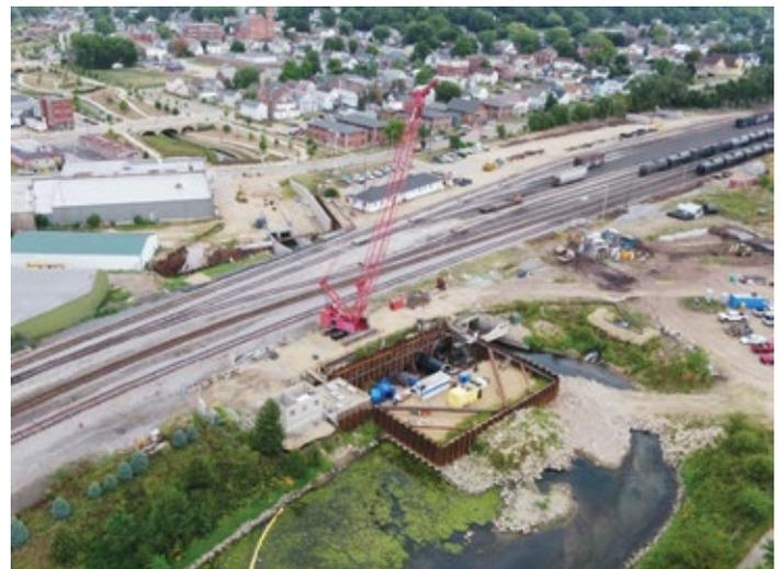
Figure 3. Aerial view of project site, looking SE across jacking shaft toward CP tracks and reception shaft. Note separation plant in upper right portion of photo, and existing storm drain culvert to right of jacking shaft
