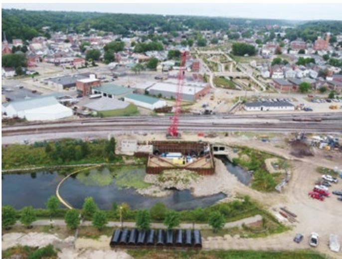
Figure 2. Aerial (drone) view of Bee Branch project site, looking east with Permalok jacking pipes in foreground, jacking shaft near center of photo, CP tracks and reception shaft in upper background
