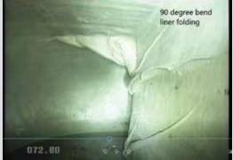
Figure 9. Post lining photos of 45- and 90-degree bend showing folds in the liner
