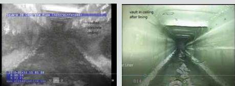
Figure 8. Before and after lining of the vaulted precast ceiling in tunnel from PST #1 to the box
