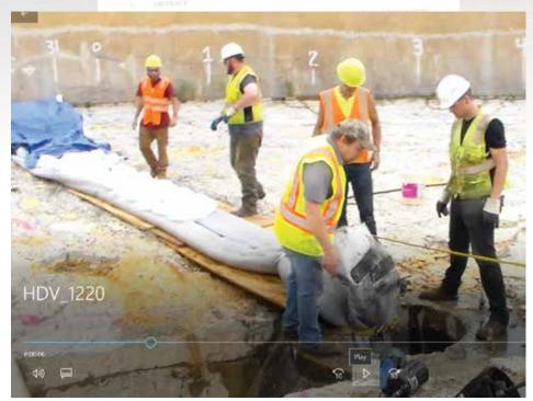
Figure 5. Preparing to load liner into tunnel in PST #1
