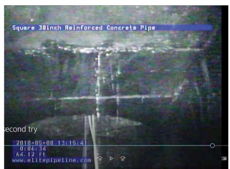
Figure 2. CCTV showing point of infiltration in effluent tunnel from PST #4 to distribution box
