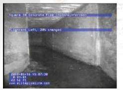
*Figure 3. Example of bends in the tunnels and existing conditions after cleaning*
