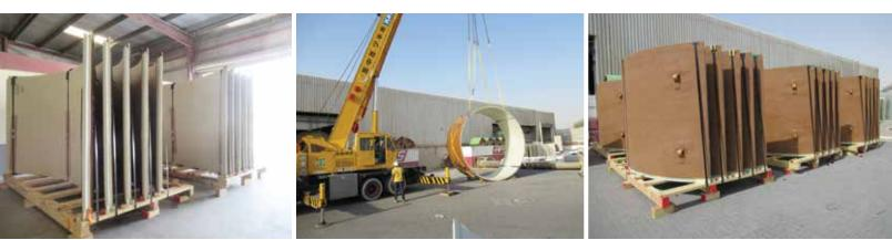
Proprietary system offered a way to break the geometrically complex pipe liners down into multiple component segments to dramatically reduce shipping costs, while still maintaining structural integrity and load capacity
