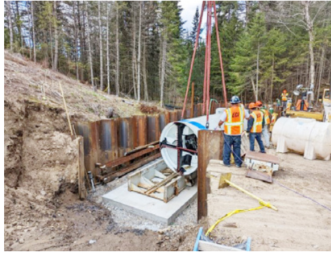
TBM lowered into launch pit. ECI crews maintain a high standard of safety
