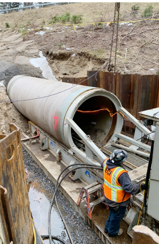
84-inch HOBAS pipe was jacked in 20-foot segments
