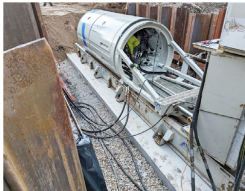
Akkerman Model 5000 Series II Pump System delivers up to 400 tons of jacking force
