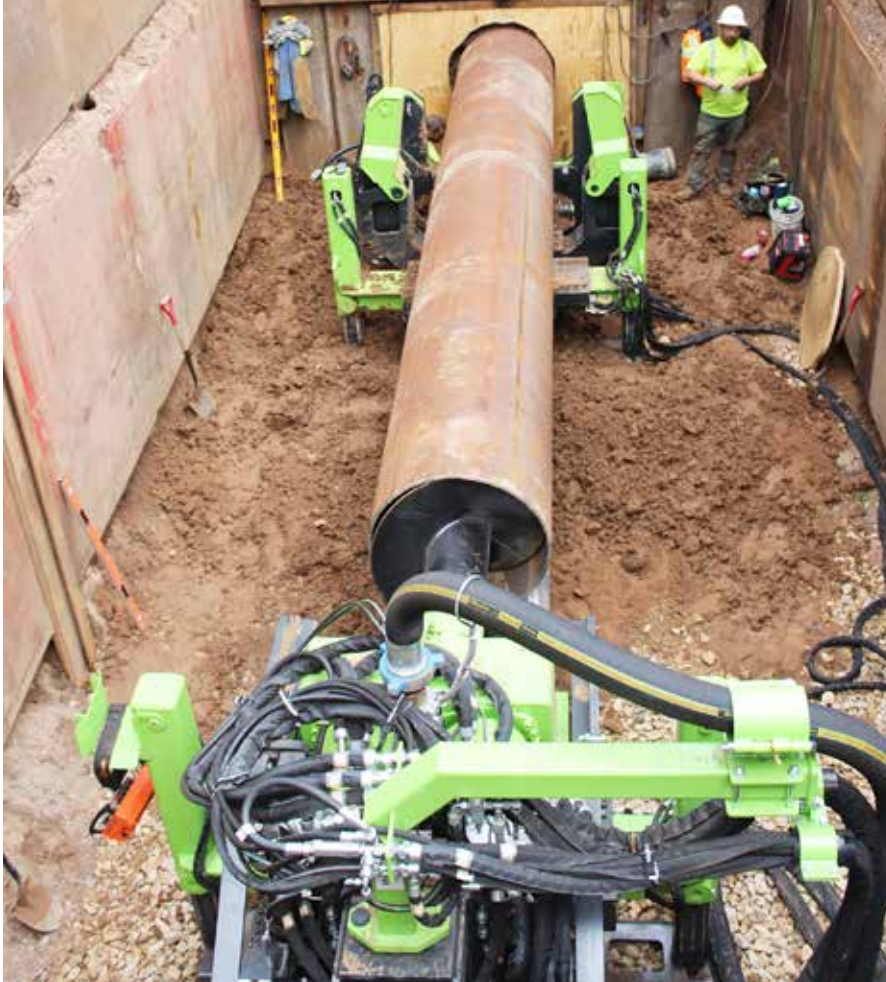
The casing advances with each cycle of the hammer
