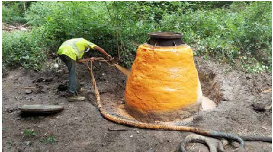
The OBIC Armor system reinforced and secured the structure of the exposed manholes
