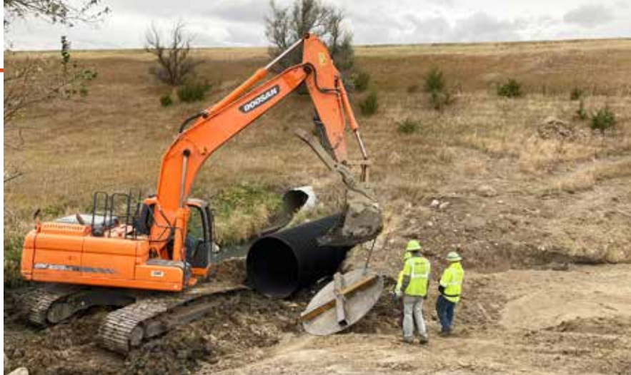
DuroMaxx® SRPE Liner Pipe being pushed into place
