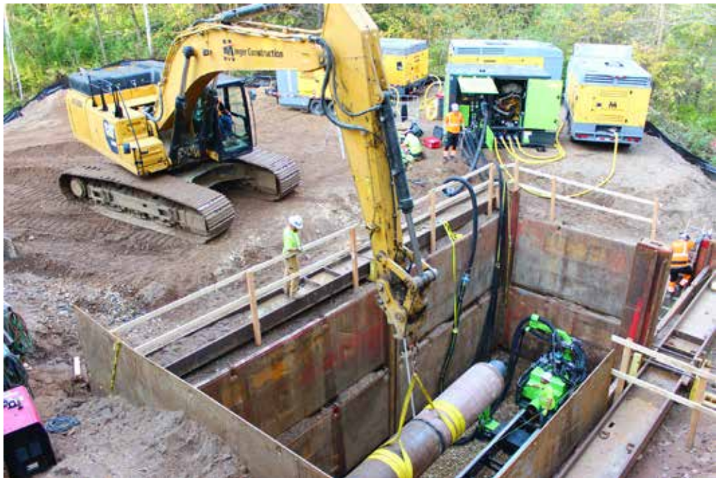
Minger Construction Crews lower the first piece of Casing to be installed with their new GEONEX HZR1200 Boring equipment in Scandia MN
