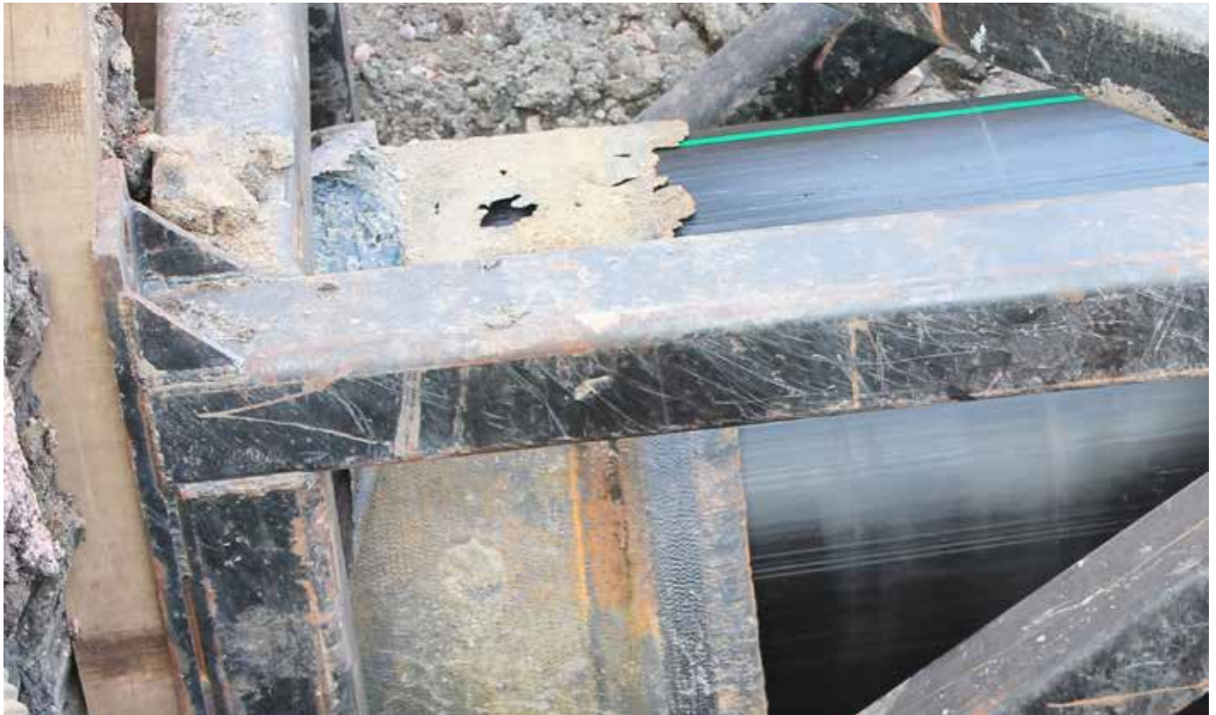
Replacing the Sioux Falls corroded ductile iron pipe that had been eaten away by sulfuric acid caused by sewage, the HDPE pipe is inserted into the destroyed pipe using the CompressionFit method from Murphy Pipeline (PHOTO CREDIT: MURPHY PIPELINE)
