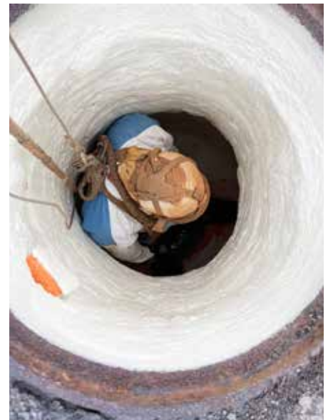
Material provides a monolithic lining system
