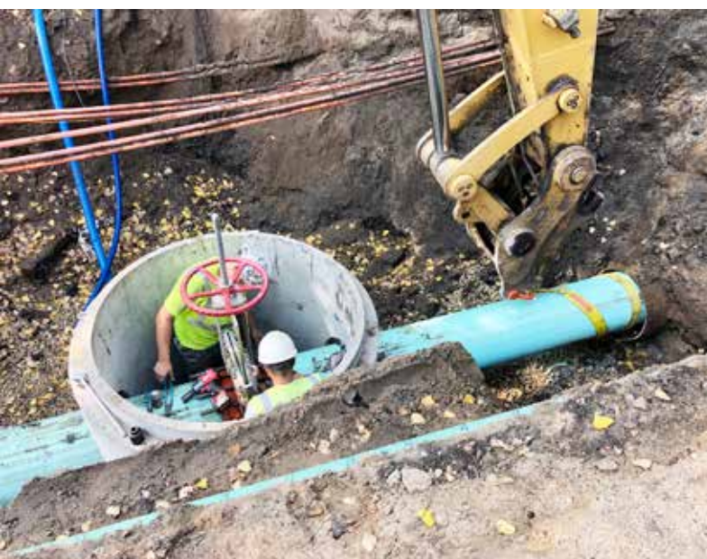
Fitting locations were used as insertion or receiving pits
