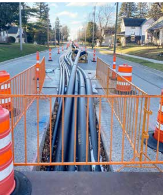
Pipe bundle string was set out down the middle of a heavily trafficked local road
