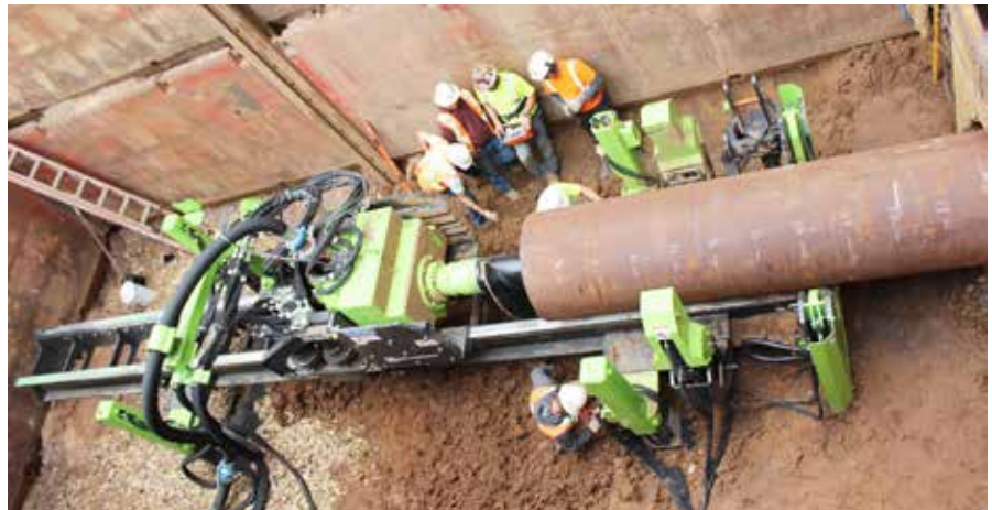
Though Down Hole HHB is a non-guided method, accuracy was achieved with help from GEONEX technicians onsite
