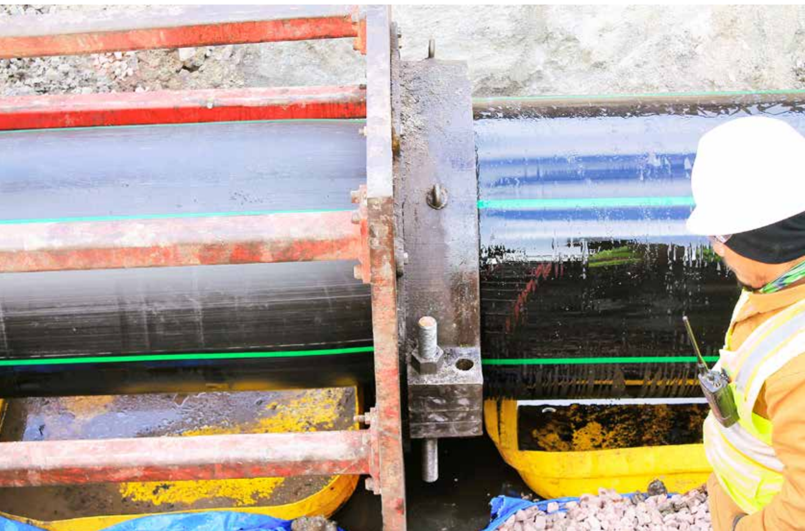
The new 36-inch HDPE pipe replaces the corroded ductile iron pipe in the Sioux Falls, SD sewer system (PHOTO CREDIT: MURPHY PIPELINE)
