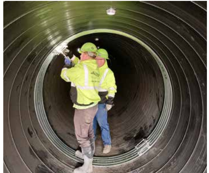
Using internal expanding bands allowed for optimized OD/ID of the liner pipe to meet hydraulic requirements
