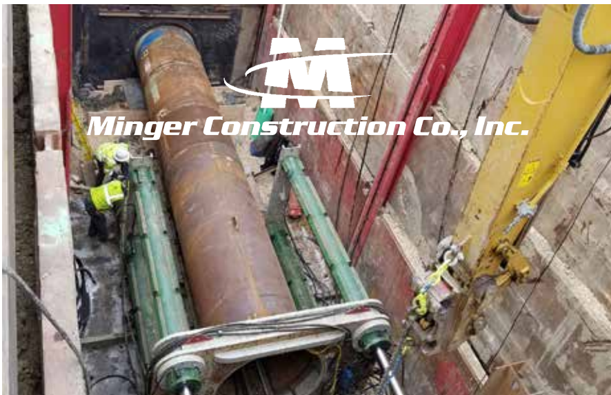
The casing advances with each cycle of the hammer
