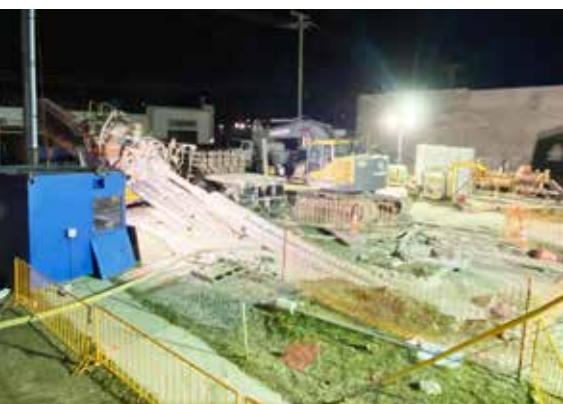
Pullback was completed with no damage to any conduits
