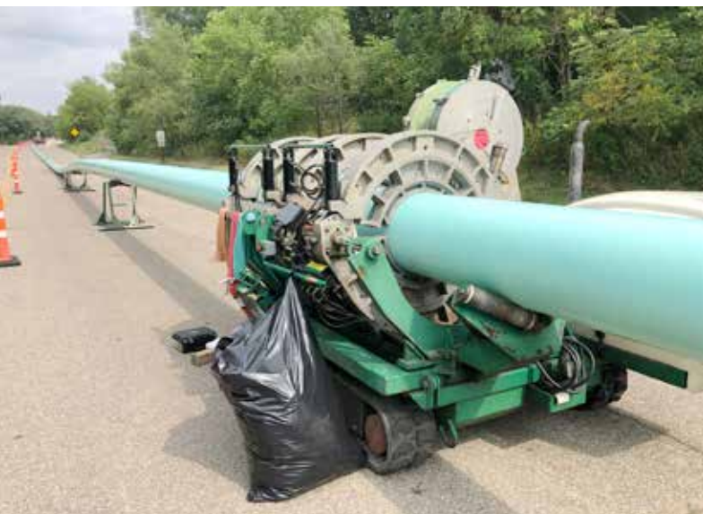
The 18-inch Fusible PVC was installed in 500 to 1250-foot lengths
