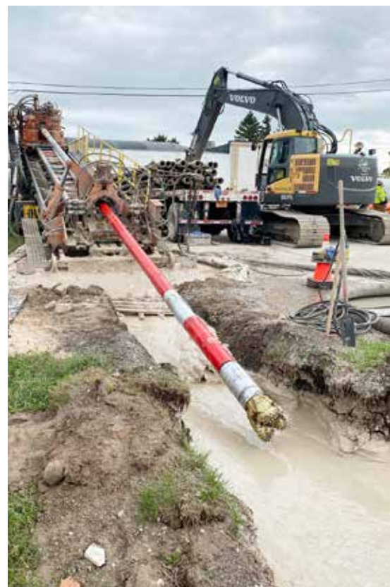
Extremely hard rock required hard formation tooling
