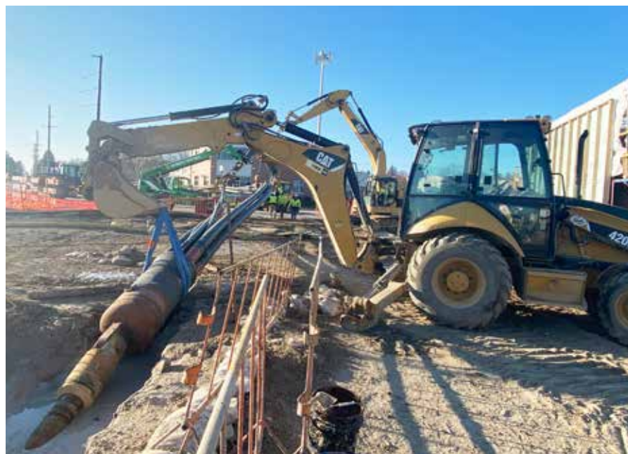
Buoyancy modification was not used during pullback
