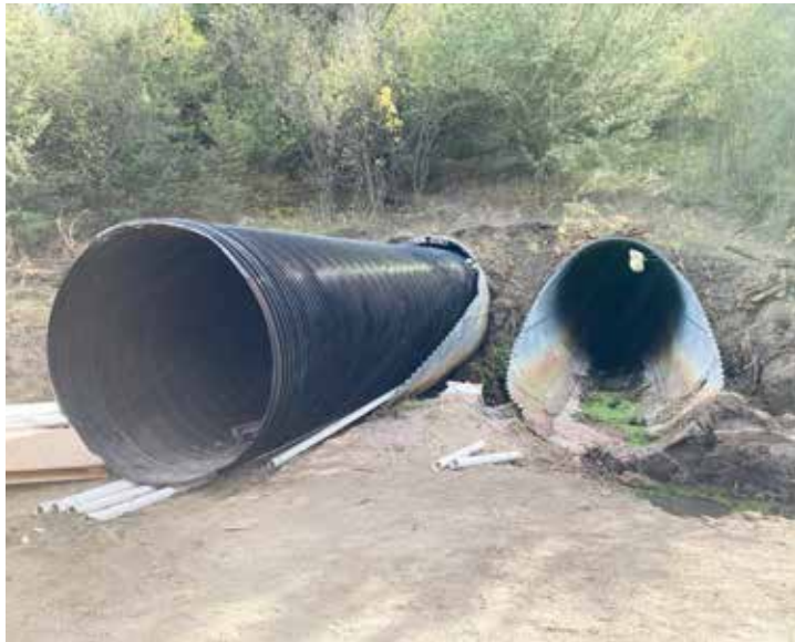
Use of "guide rails" ensures proper placement of liner pipe into the existing host pipe
