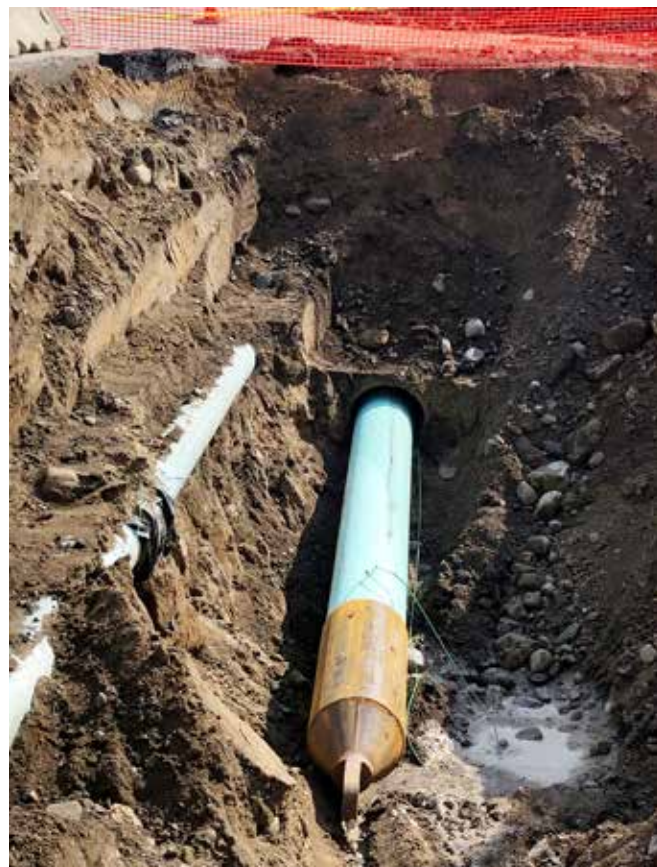
Existing ductile iron force main used as casing for sliplining new force main
