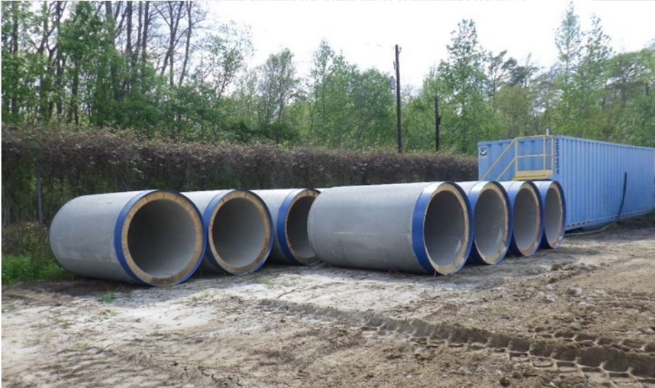
Figure 6. RCP Jacking Pipe
