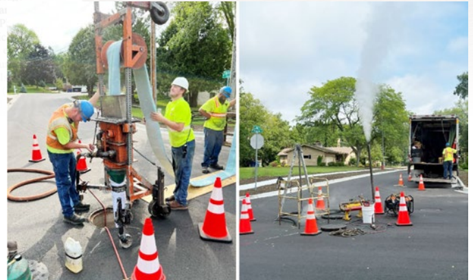
CIPP shooter (left) and the emission stack (right)
