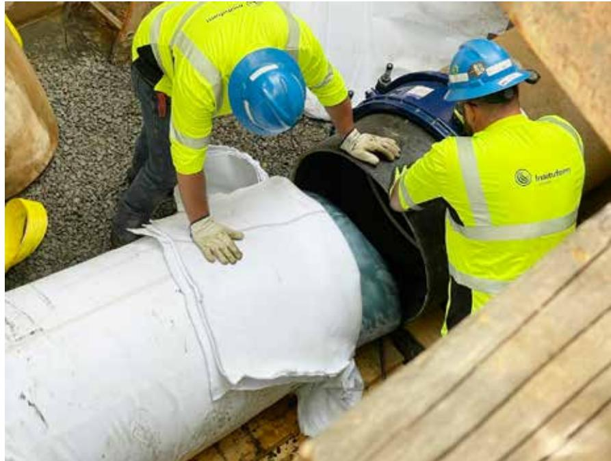
*Using an updated methodology, termination of the liner was done outside of the host pipe*
