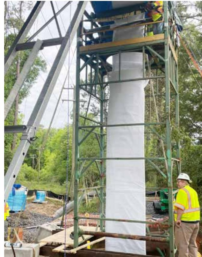
material with the resin system and is done in a highly controlled facility environment under strict quality controls that far exceed field wetout conditions. The wet tube was then shipped in refrigerated trucks to the jobsite in South Carolina sequentially for each installation and phase of the job.
