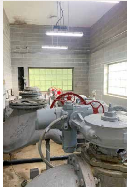
Figure 4: Lift Station Check Valves - Insertion Points
