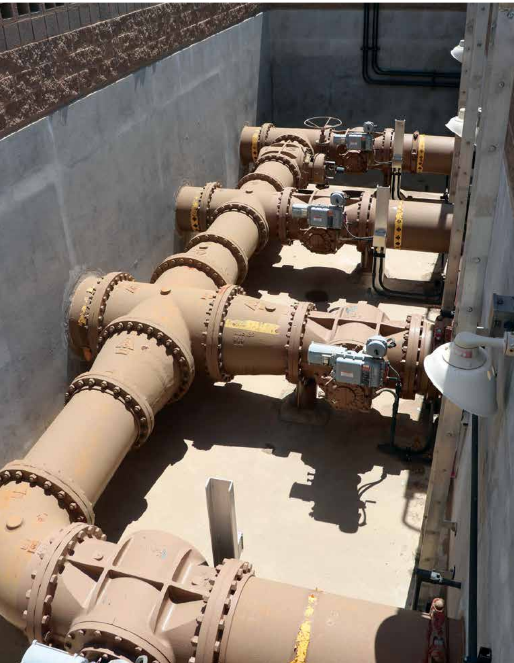
The Cave Creek facility could be operational by 2026 and could start supplying Phoenix residents with drinking water in 2028.
